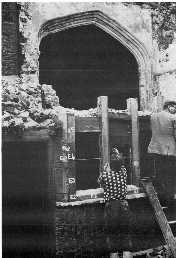
XLIX. Dismantlement of bay window, Building 3132, in 1962 (Photographer unknown)
