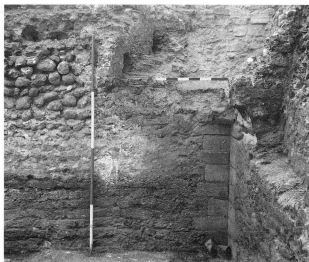
XXXII. Inserted stair 2143 in south-eastern corner of Building 2100 (contemporary surfaces removed). Recess in wall on the right may have been for a door to the stair. Scale: 2 metres (BWE4)
