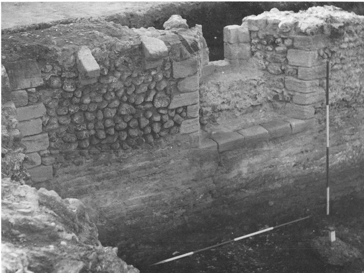
XVIII. Window opening 2130 at southern end of wall 2105, Building 2100. The photograph also shows the apparent rendering on this wall. The corbels and traces of brick vault are later insertions. Scales: 2 metres
