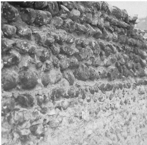
XII. Internal face of wall 115, Building 2100, showing construction 'lifts' (BWL7)
