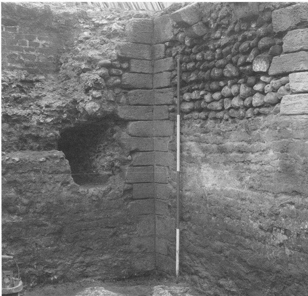
XIII. Internal quoins in south-west angle of Building 2100. Scale: 2 metres (BWE5)
