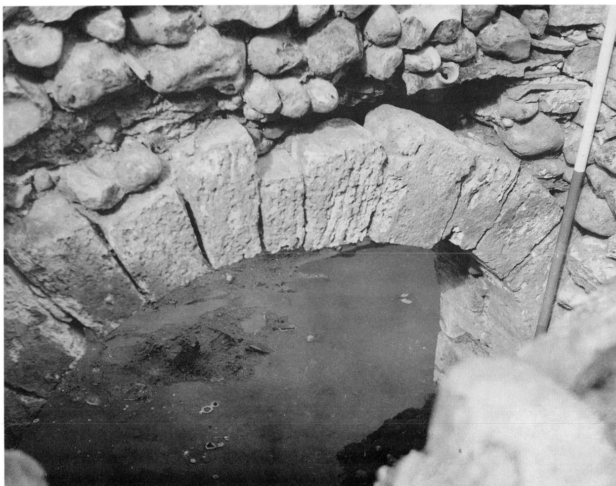
XXIX. Interior of latrine turret 2025, showing repairs using ridge tiles. Scale in half-metres (BWC1)
