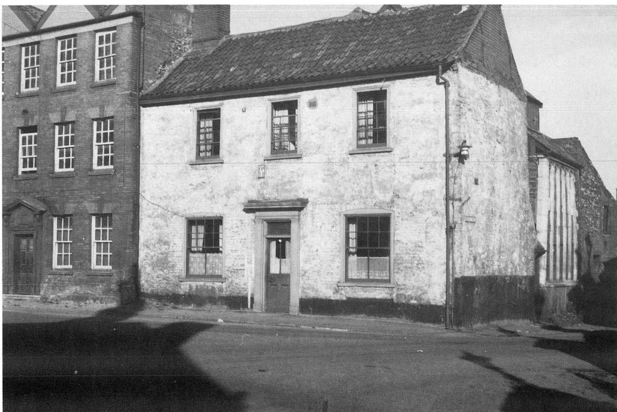
XLVI. Building 3132 (18, St. Martin-at-Palace Plain) in 1946. (Copyright: Royal Commission on Historical Monuments England)
