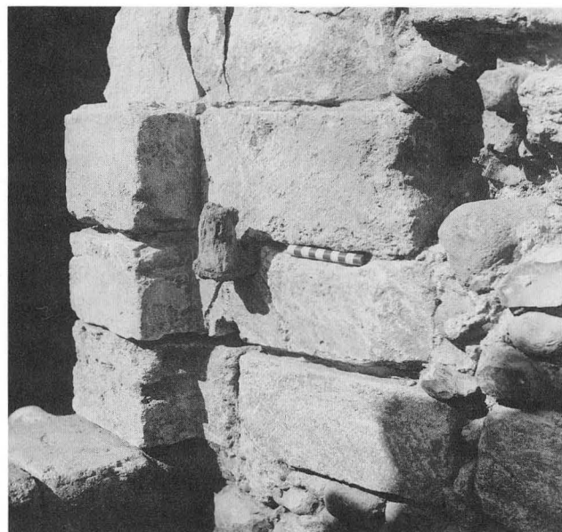
XVII. Doorpin in northern side of doorway 2004, Building 2100. Scale in centimetres (BWC8)
