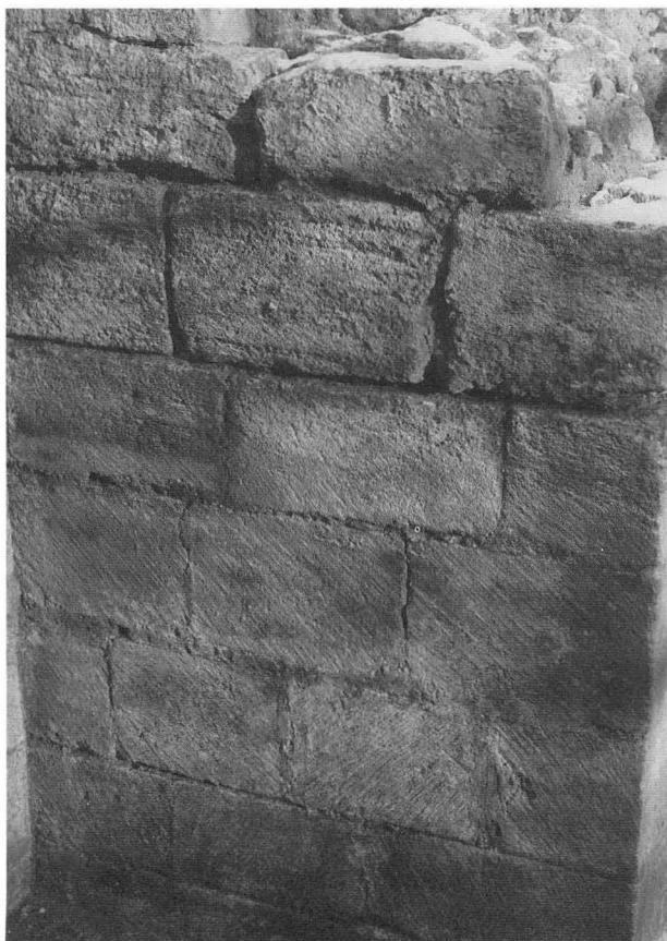
XVI. Toolmarks on western face of buttress 2135, Building 2100 (BWL19)
