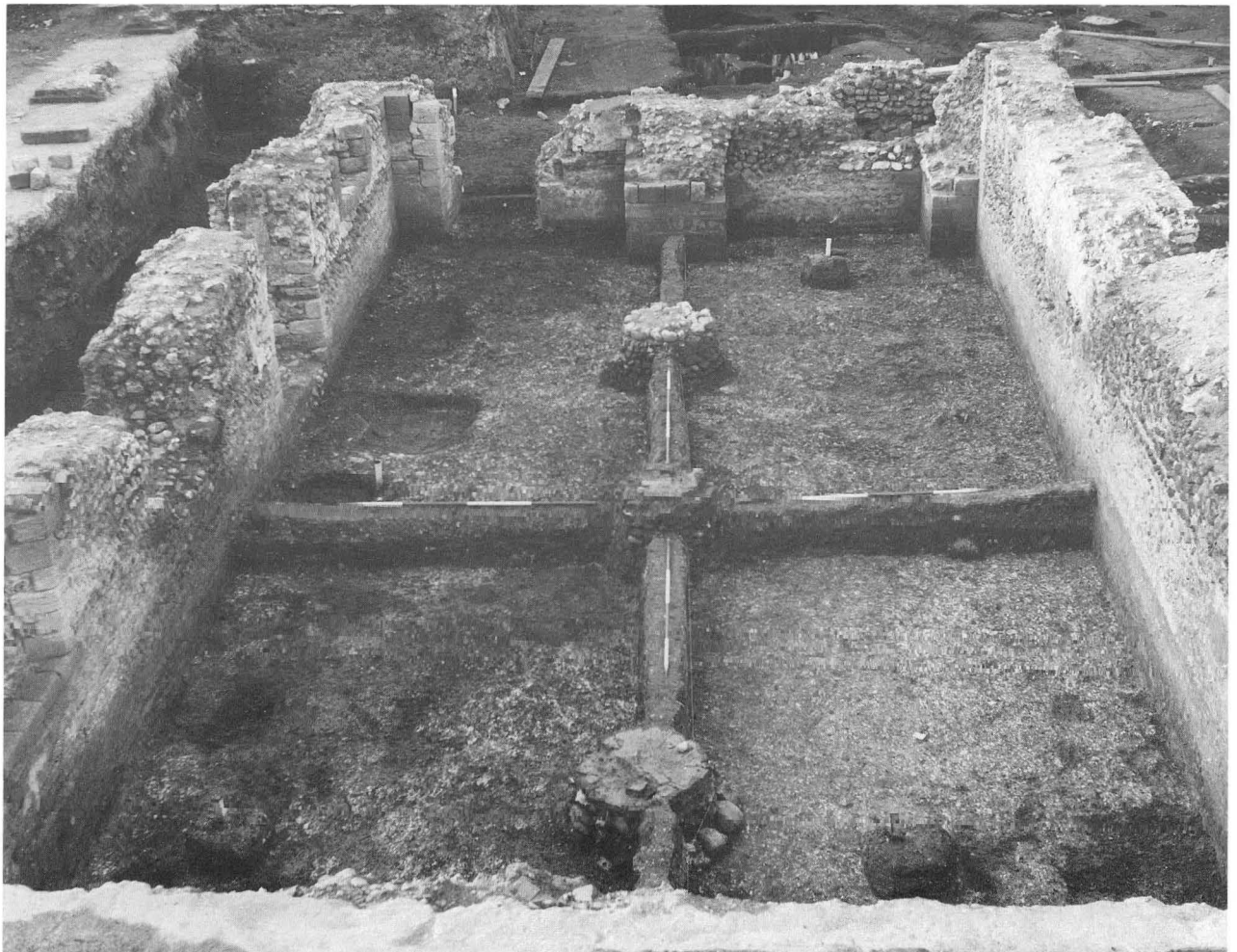
XV. Interior of Building 2100 showing floor surface 2142 and buttresses 2135 and 2136 at the north (furthest from camera) end. The pillar bases are later insertions and the scales rest on baulks of soil left by the excavation. Scales: 2 metres (BWE1)
