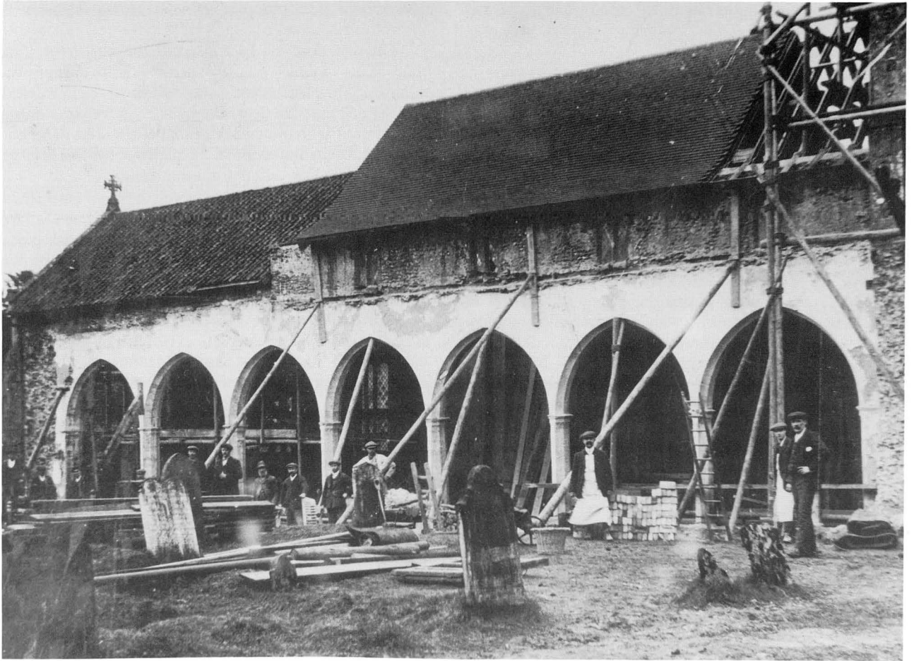
Plate XI Rougham: Undated photograph hanging in St Mary's church showing the rebuilding of the north aisle in c. 1910 (Fig. 20). (Provenance unknown).
