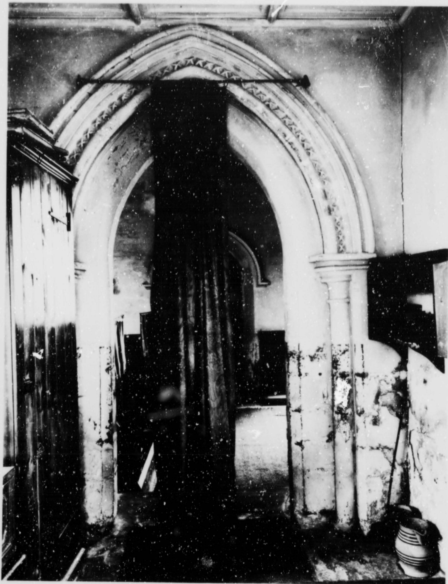
Plate CLIX. Buckenham Ferry, St Nicholas, nave north doorway from north AA52/5605
