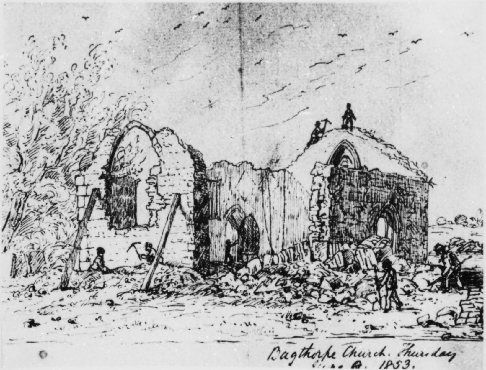
Plate CXXXV. Bagthorpe, St Mary, demolition in June 1853
