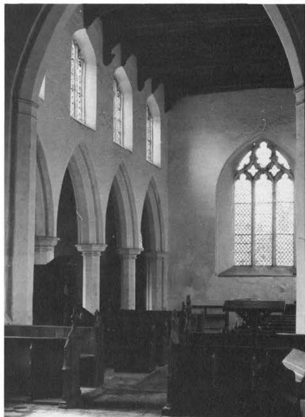
Plate XXXI. Hockwold, St Peter: looking west, with Decorated west window and arcade, but Perpendicular clerestory and roof.
