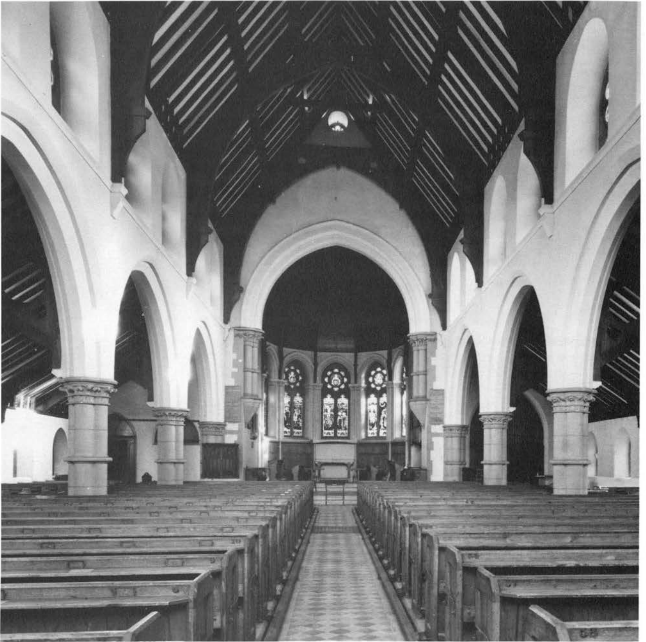
Plate CXXVIII. Heigham, St Philip: interior in 1976: in good condition and a good example of Edward Power's work (1871), demolished in 1977. BB77/5878 copyright Royal Commission on Historical Monuments (England).
