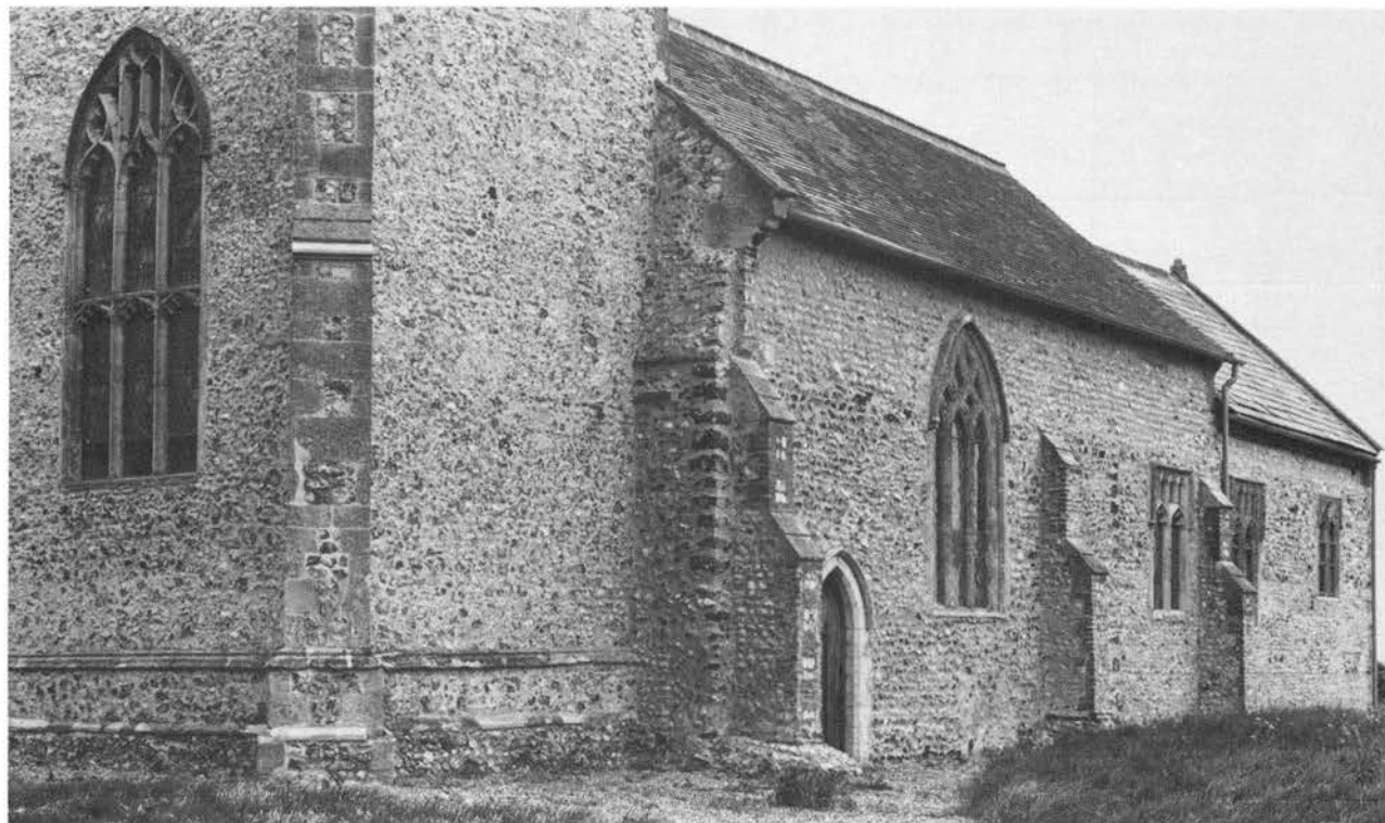
Plate LXVI. North Barningham, St Peter, from the south-west. The quoins of the Phase I nave can be made out; notice also that the nave has been first lengthened, then heightened.
