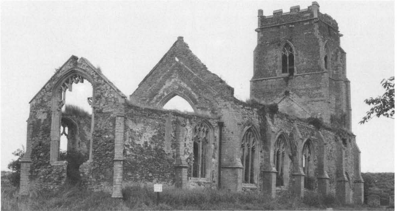
Plate XXXIV. Wiggshall St Peter: from the north-east; a complete (but roofless) Perpendicular church of the 1420s.
