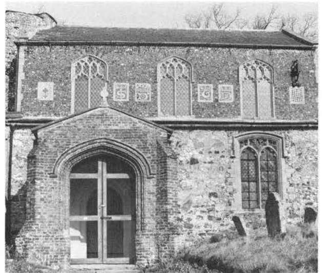
Plate XXXVI. Feltwell, St Nicholas: re-set flushwork panels in the clerestory.
