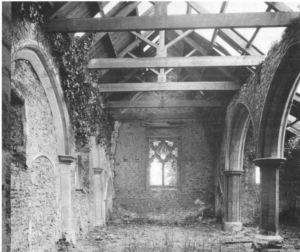
Plate LXXVII. Babingley, St Felix, nave looking east in 1947. The north arcade and the chancel arch were blocked in the 17th century; the Decorated east window probably came from the south wall of the chancel. The roof has now gone. AA47/9209 copyright Royal Commission on Historical Monuments (England), 1947.
