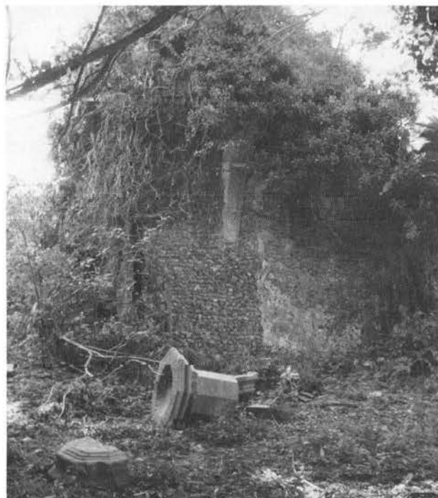
Plate CI. West Raynham, St Margaret: interior looking north-west, showing springing of west arch of north arcade.
