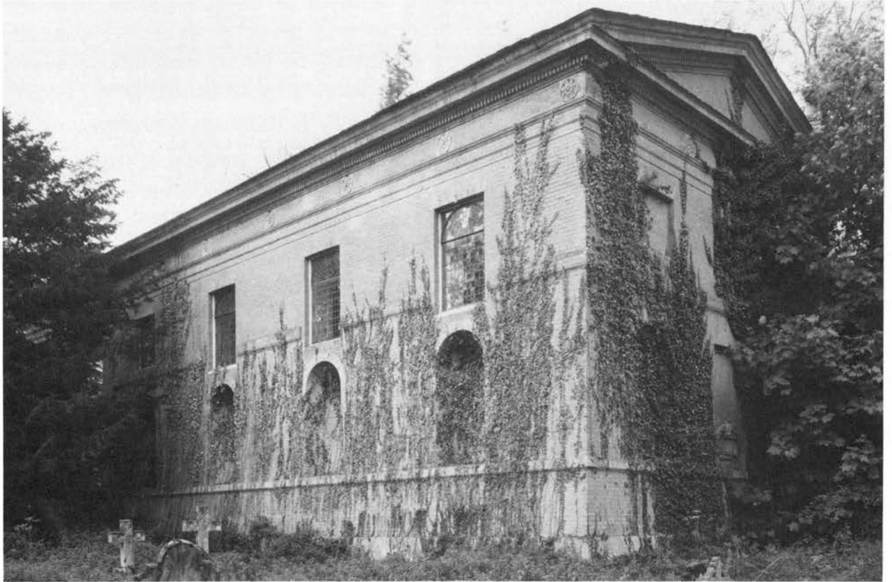
Plate XXXIX. Gunton, St Andrew: view from south-east. The 18th-century church is built on the site of its medieval predecessor. BB77/5944 copyright Royal Commission on Historical Monuments (England).
