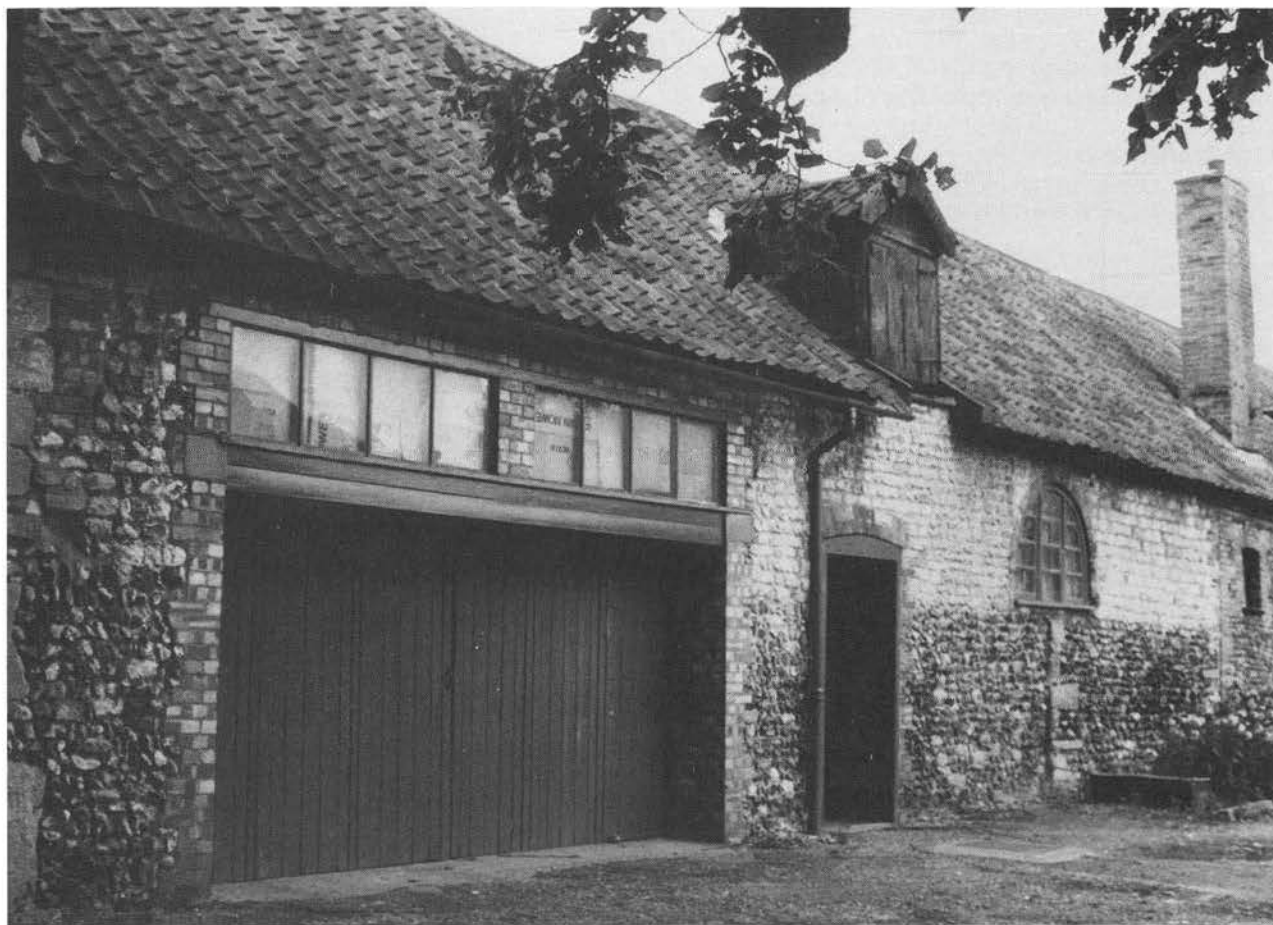
Plate CIV. Snarehill: formerly a church, later on stables, now a garage whose double doors occupy the western half of the nave south wall.
