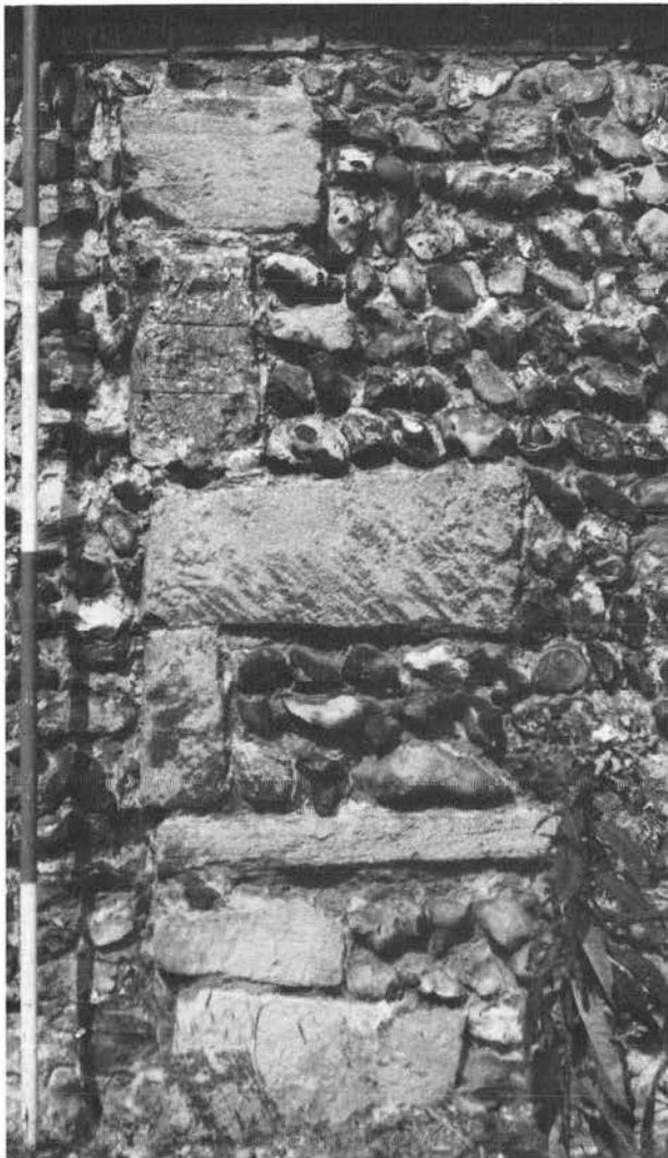
Plate CV. Snarehill: west quins of salient feature in south wall (either tower or transept); note coarse diagonal tooling.
