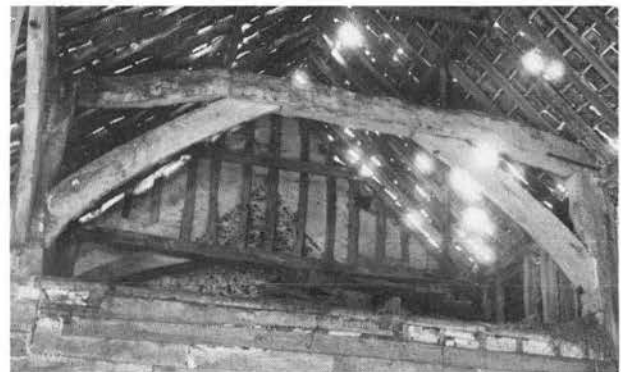
Plate CVI. Snarehill: gable of west wall of nave, seen from inside barn.
