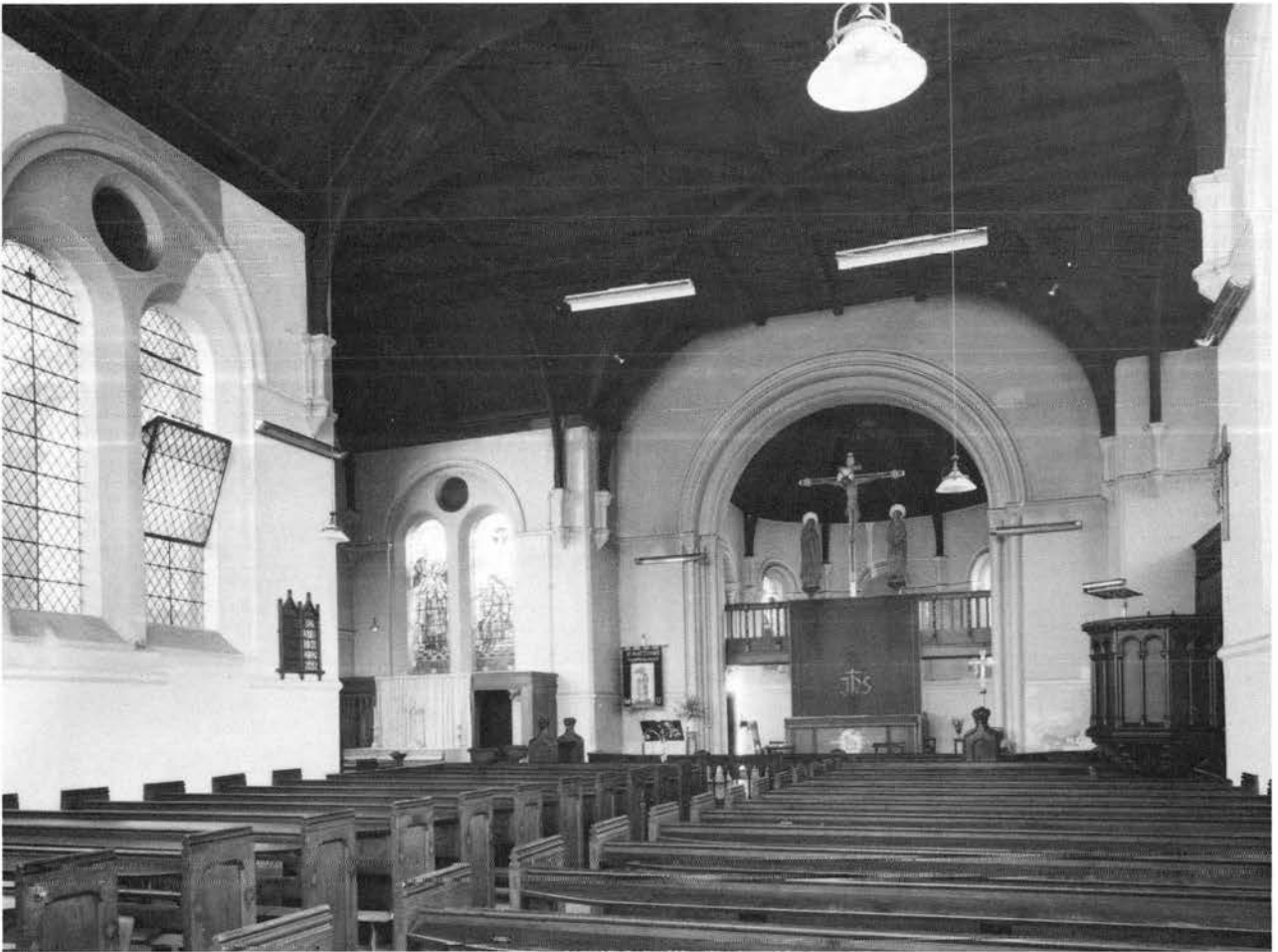
Plate CXXX. Thorpe Hamlet, St Matthew: interior in 1976. Although not destroyed, John Brown's design of 1851 has been divided into several storeys of offices. BB78/9643 copyright Royal Commission on Historical Monuments (England), 1976.
