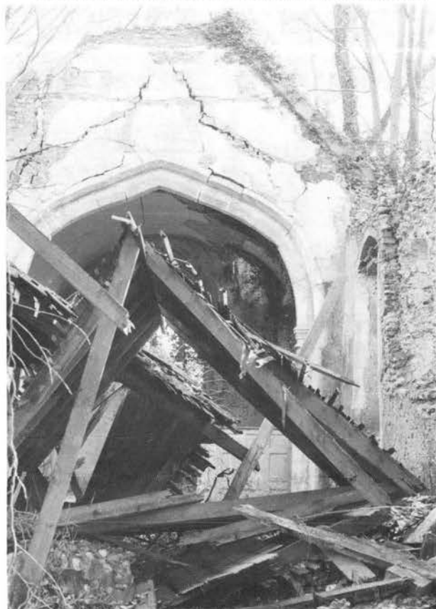
Plate LXXXVII. Kempstone, St Paul, interior looking east, 1978. The chancel arch had collapsed by 1983.
