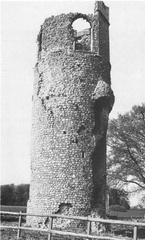
Plate XXXV. Wolterton, St Margaret: a round tower of c. 1390 with integral brick stairway. The rest of the church was demolished c. 1740, leaving the tower as a 'picturesque' ruin in the grounds of Wolterton Hall.
