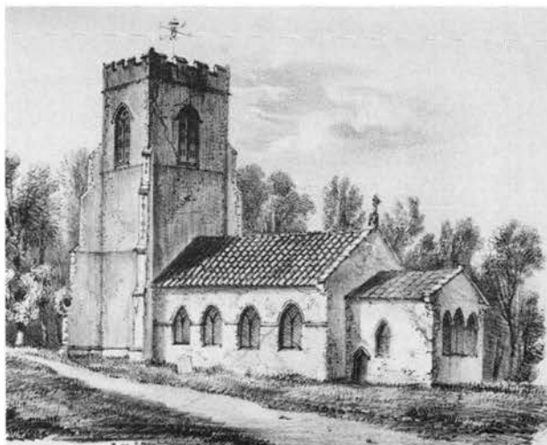
Plate LXXI. West Tofts church by Ladbrooke (1832). The chancel and north aisle had been removed in 1786 and a squat new chancel added. This shows its appearance prior to Pugin's rebuilding.
