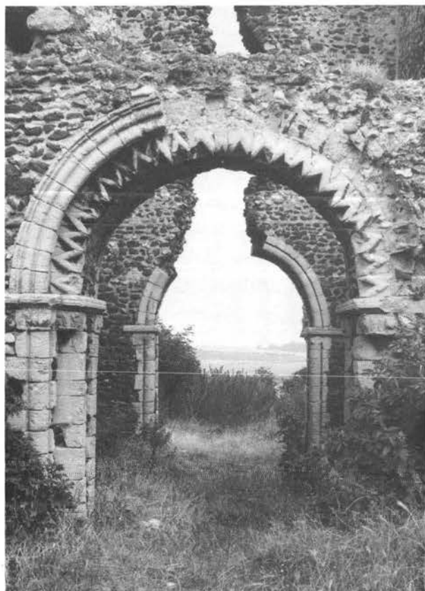
Plate XCIII. Bawsey, St James, tower arch looking east, with chancel arch beyond; tower arch shafts, with scallop capitals and arch with chevron decoration.
