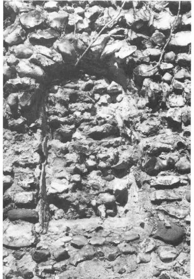
Plate CII. Saxlingham Thorpe, St Mary: chancel north wall, internal splay of a (blocked) single-splayed round-headed window.
