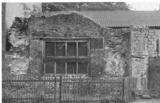
Plate CXIX. King's Lynn, St James: north wall of north transept; the wooden window belongs to its post-medieval transformation into a workhouse.
