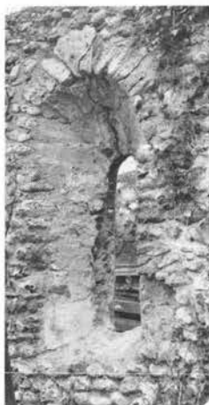
Plate XXI. Kempstone, St Paul: double-splayed window in south wall of nave.
