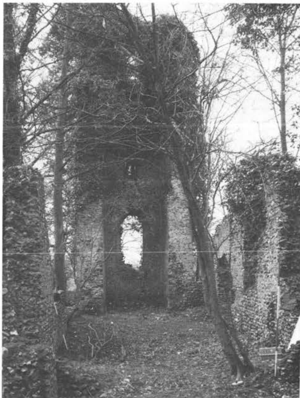
Plate CIII. Saxlingham Thorpe, St Mary: interior looking west.
