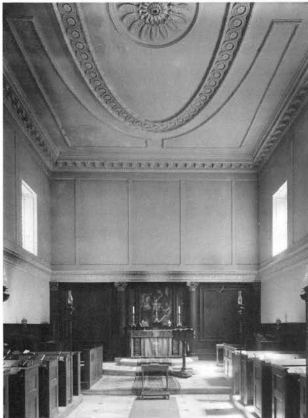
Plate XL. Gunton, St Andrew: looking east. This plaster ceiling collapsed in 1976 but has been replaced. AA49/6063 copyright Royal Commission on Historical Monuments (England), 1948.
