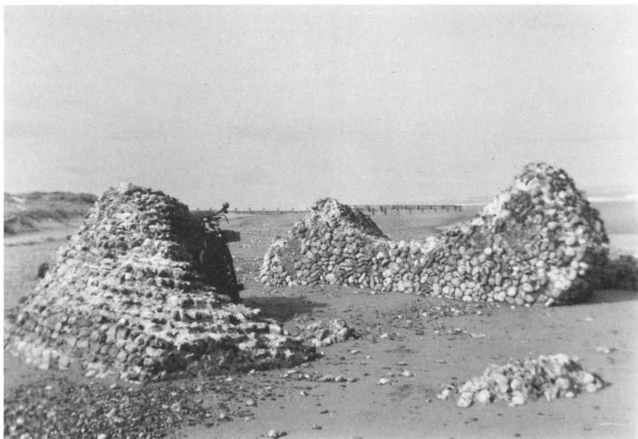
Plate XII. Eccles-next-the-Sea, St Mary: the distinctly curved masonry of the round tower exposed after a storm. Most of the village was engulfed by the sea in 1604, leaving only the church tower; the latter fell after a storm in 1895. Copy print held in Sites and Monuments Record, Norfolk Archaeological Unit.
