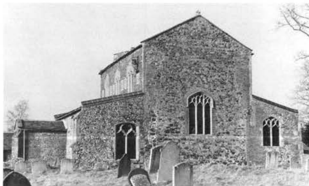
Plate LX. Feltwell, St Nicholas: from the south-east in 1980. Its oddly truncated appearance is due to the demolition of the chancel in 1861 and the collapse of the tower in 1898 while it was being repaired.
