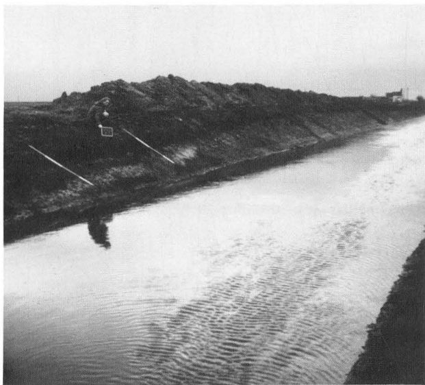
Plate XIII The southwestern edge of Northey 'island', Dyke 9 (Site 5).
