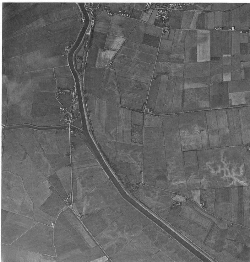
Plate III Three courses of the River Witham near Dogdyke. The Bronze Age course flowed left to right across the bottom of the picture. The modern river is the large watercourse in the centre of the plate while the irregular field boundaries in the bottom right mark the medieval course. ( Cambridge University Collection: copyright reserved )
