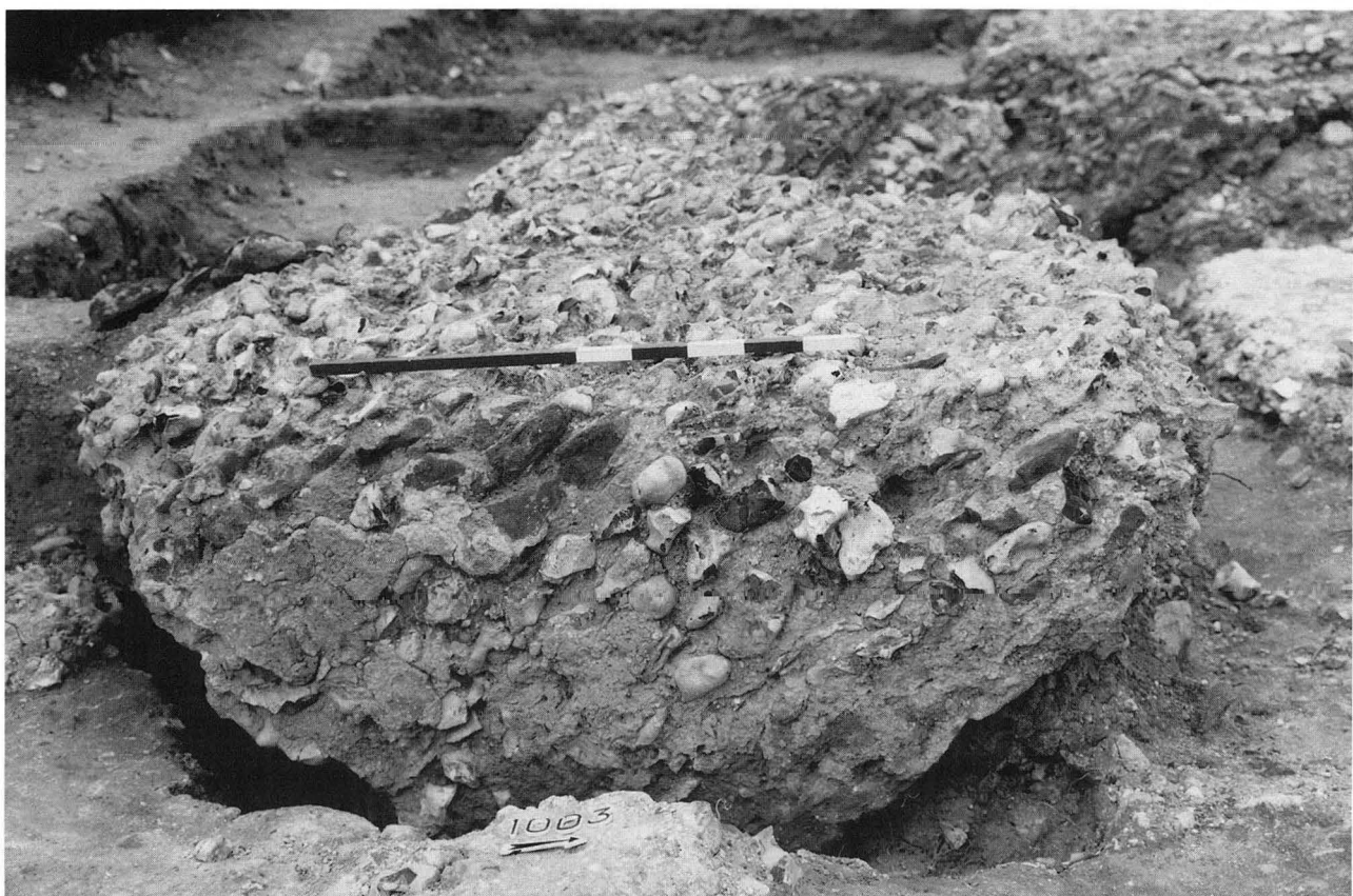
Plate XXXIII Period III. Detail of collapsed wall, south side of tower. Note that subsequent robbing has 'chamfered' the interior face. View looking west. Scale 1 metre. (Photo: B.Lloyd)
