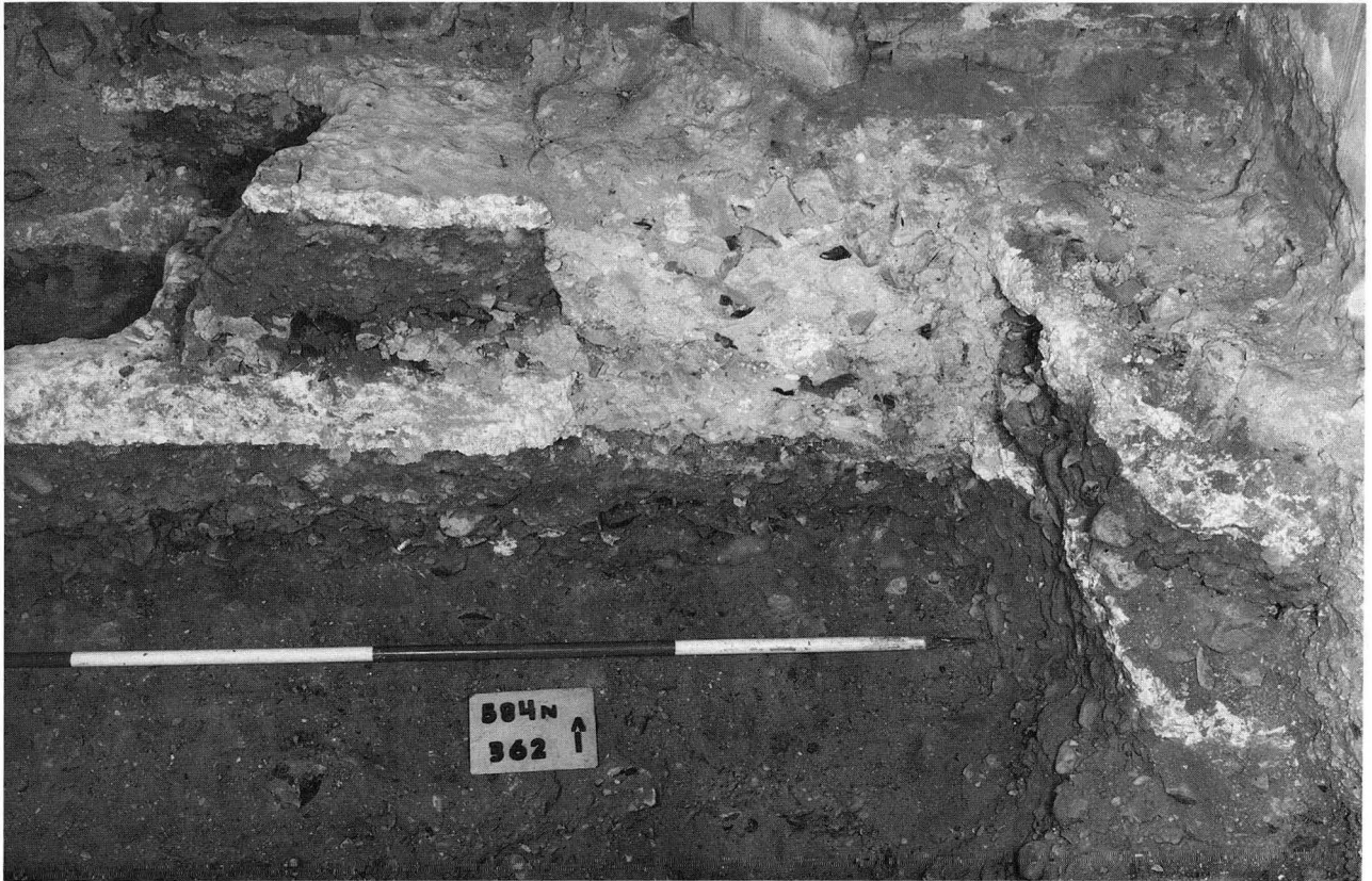
Plate XIX Foundation of rebuilt chancel arch (769). Scale 1 metre
