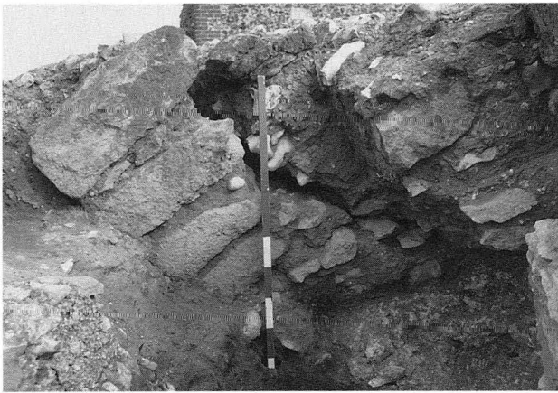
Plate XXVIII Period I church. Collapsed conglomerate quoins, exterior junction of north nave wall and tower. View looking east. Scale 1 metre. (Photo: B.S.Ayers)
