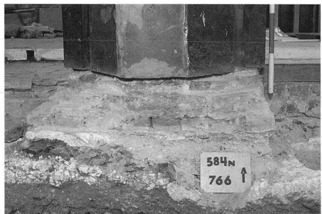
Plate XVIII Rebuilt pier base (766) in nave arcade. Scale 1 metre
