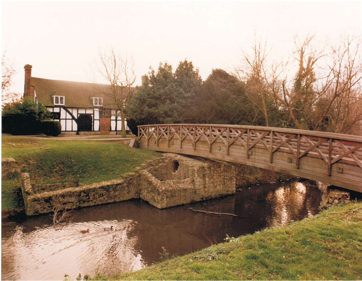
Plate 2 Hall following excavation, consolidation of excavated walls and provision of new bridge. The foundations of the gatehouse (structure III), garderobe (structure V), retaining wall of structure IV with the second garderobe (structure VI) behind, can all be seen on the bank of the moat
