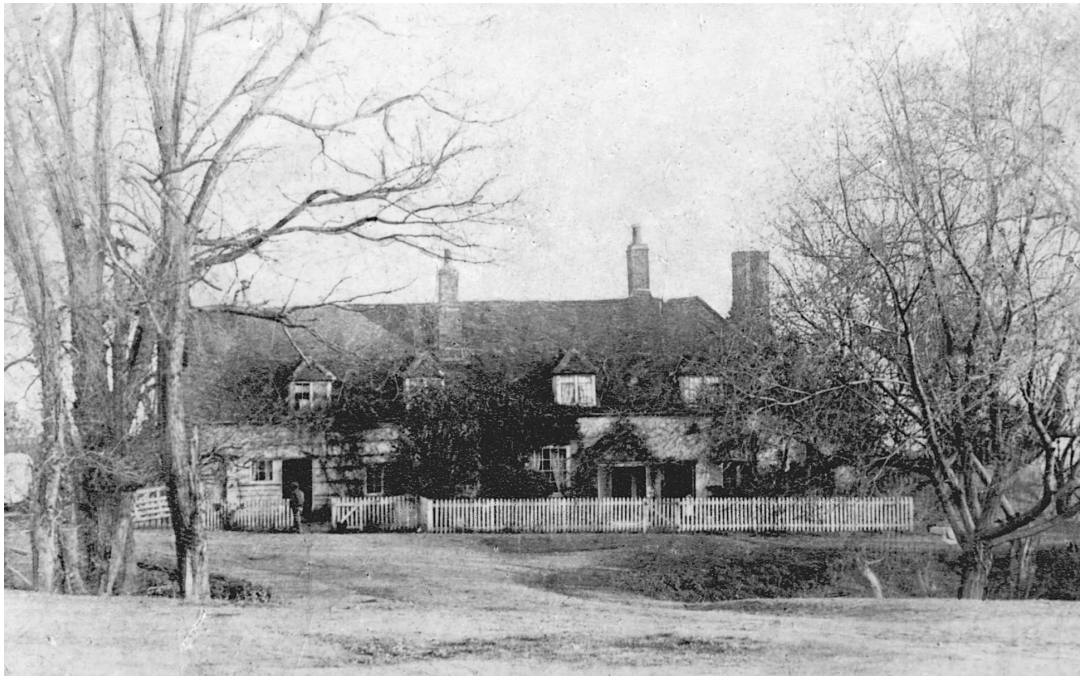
Plate 1 Southchurch Hall before restoration about 1920
