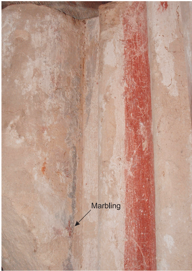
Engaged shafts 279 showing area of marbling - red over black
