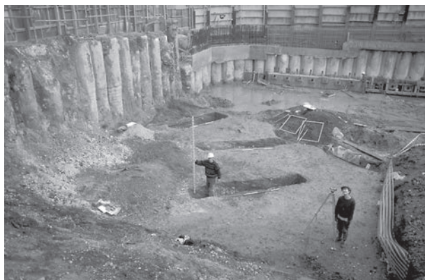
Plate 7.2 Working shot during excavation of the outermost defences of the north-east bailey (Castle Meadow), looking east (Ditch 9, Area 9)
