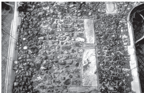
Plate 4.24 Long-and-short work in the east wall of the Church of St John the Baptist, Timberhill (formerly St John at the Castle Gate/de Berstrete)
