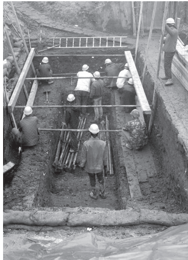
Plate 1.10 Insertion of shoring into Trial Hole 1 across the barbican ditch in 1987
