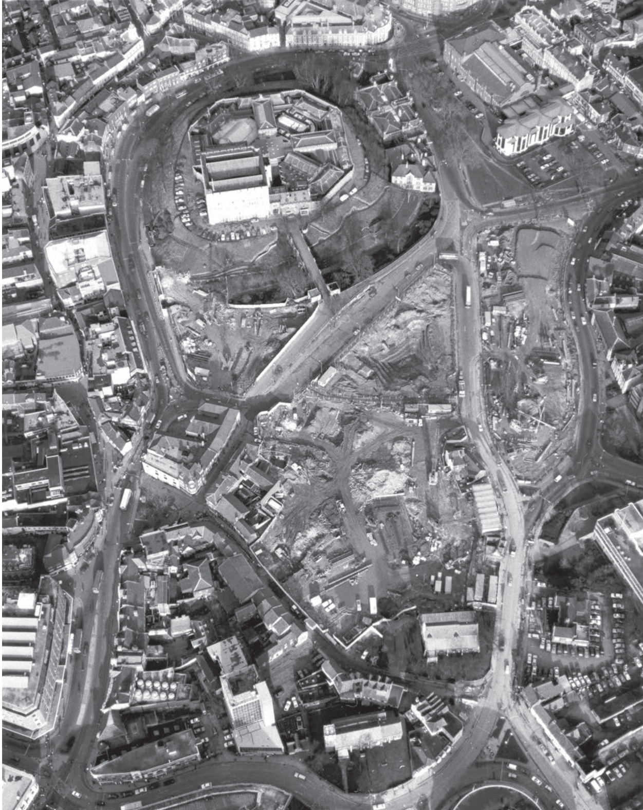
Plate 1.6 Aerial view of the Castle Mall excavations in progress, showing the stepped excavations across the barbican ditch in Area 4 photographed in February 1990 (Norfolk Aerial Photographic Library: TG231083)
