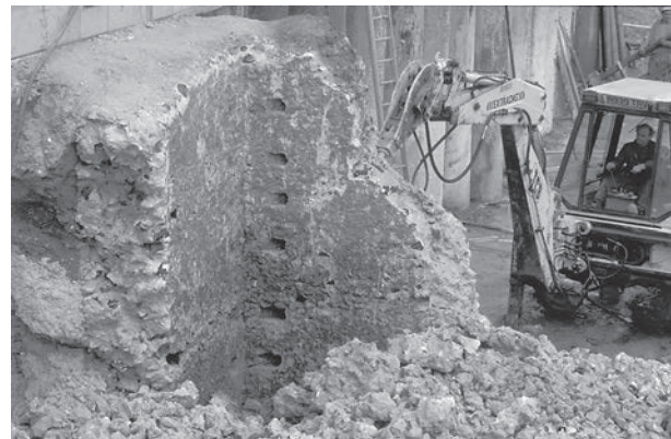
Plate 6.21 Demolition of the well shaft, showing interior putlogs (50108, Period 3.1, Area 5)
