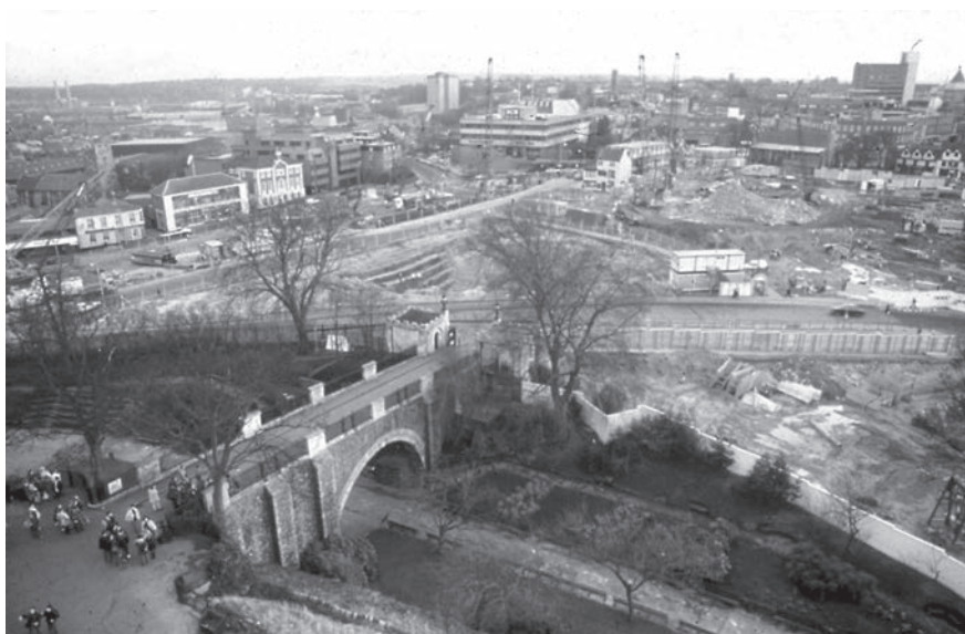
Plate 6.9 Excavations in progress, showing the castle bridge (left foreground) and, behind it, one of the stepped excavations through the barbican ditch. Viewed from the north-west
