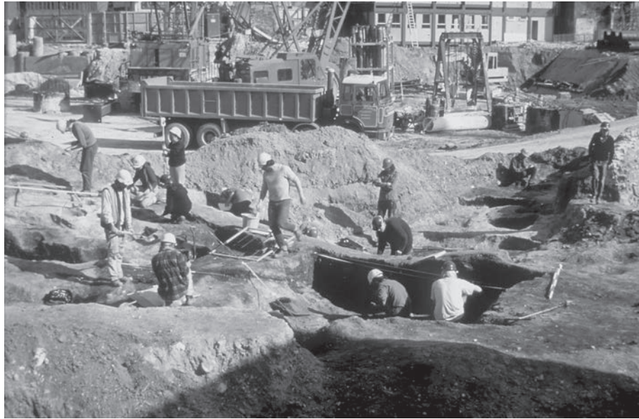
Plate 1.7 Excavation in progress at Castle Mall, showing the general character of working conditions on this joint occupancy urban site
