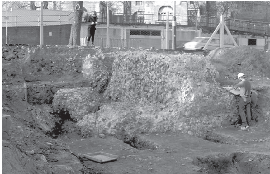
Plate 6.13 Collapsed gatehouse masonry, incorporating a buttress (40412, Period 3.1), viewed from the south (Area 4)
