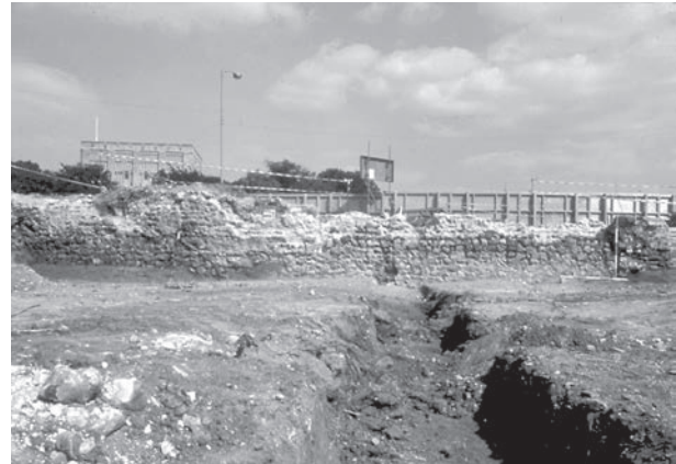
Plate 8.7 Mid 16th-century garden/terrace wall 80034, Open Area 50 (Period 5.2)
