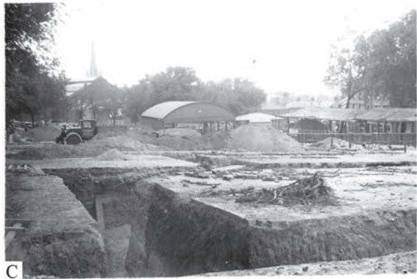
Plate 11.11 Construction of air raid shelters, 1939 (photographs by G.A.F. Plunkett; courtesy of Jonathan Plunkett):
