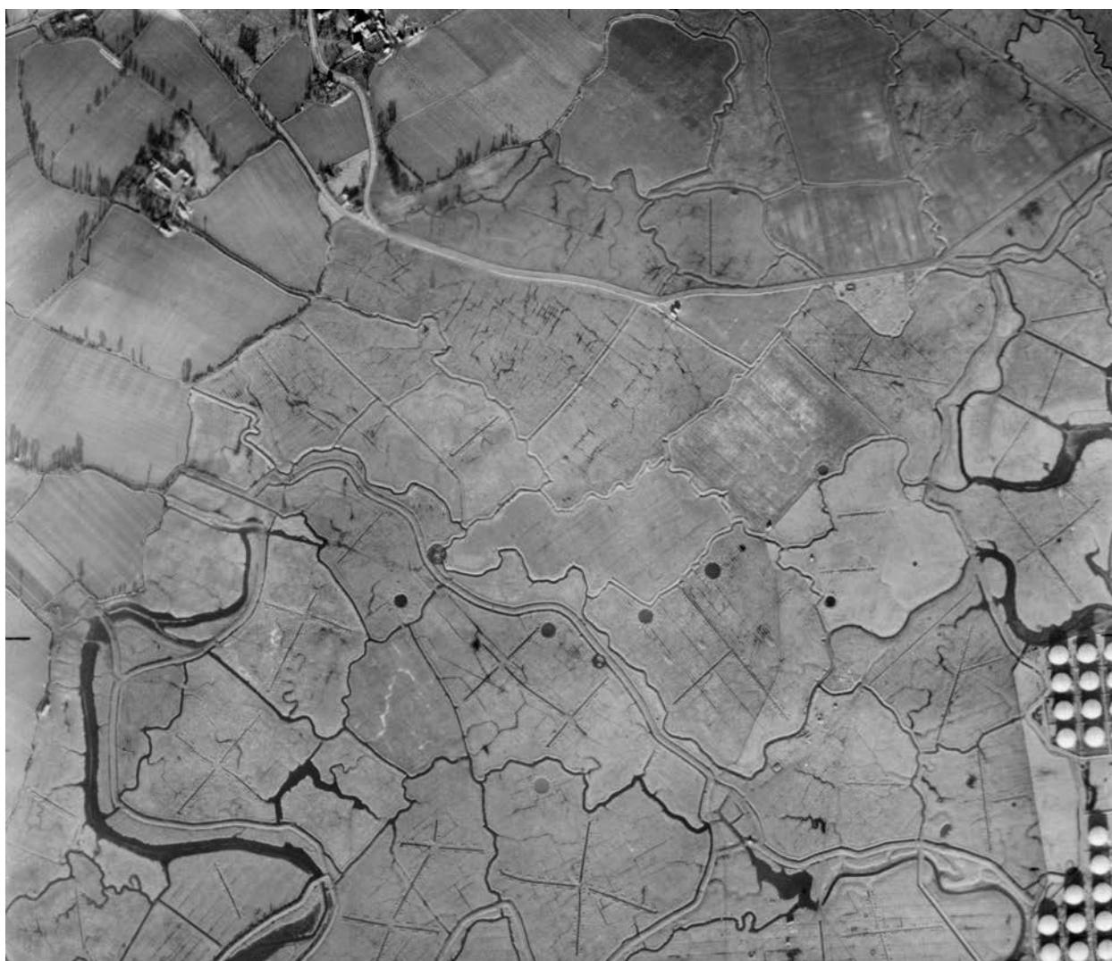
Figure 6.3 Anti-landing ditches on the Thames marshes to the south of Corringham, around the industrial sites at Shellhaven and Thames Haven. A number of bomb craters are also visible. North to the top of photograph. (CPE-UK-1923-4024 held at the National Monuments Record)
