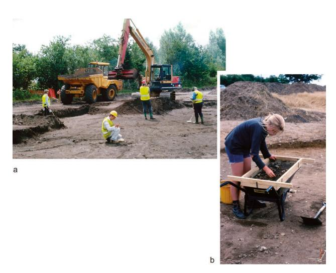
Plate 1.3 Site clearance and sampling: a – mechanical clearance was monitored intensively by metal-detector; b – overburden and 'Dark Earth' layers were sampled by targeted sieving
