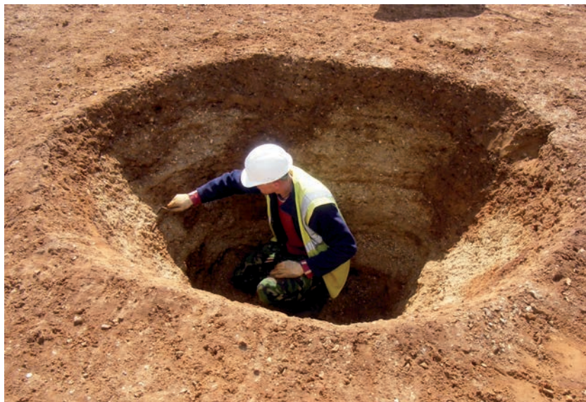
Plate 4.13 One of the fully excavated pits in alignment L2801
