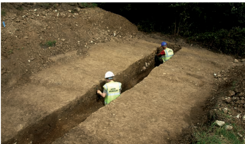
Plate 5.10 Road L5305 within pipe trench investigations, from the south-west
