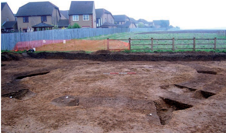
Plate 4.29 Enclosure L107/L108/L120 (farmstead SL31), from the west, with its entrance visible in foreground (2m scale)
