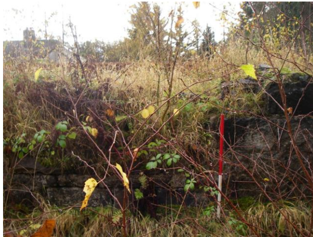
Plate 5. Northernmost, north facing wall with window aperture, Alva House (Photo 18).
