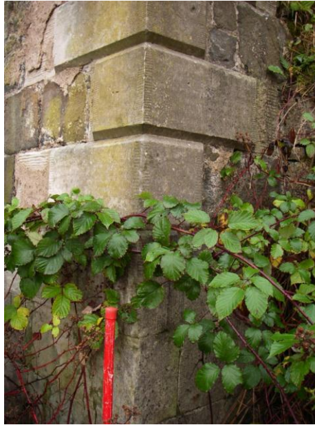
Plate 2. Rusticated quoins of west wing, south facing façade with flat, dressed stone 'simple stylobate' visible at the base, Alva House (Photo 39).
