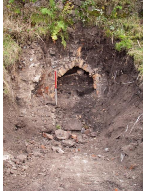
Plate 7. Brick barrel vaulted niche, Alva House (Photo 65).
