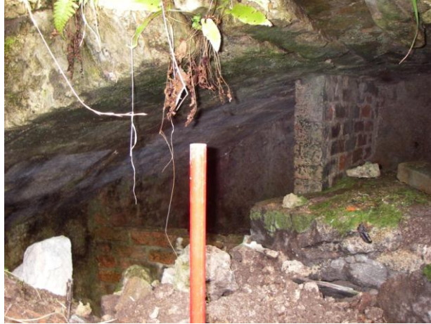
Plate 12. Stone barrel vaulted cellar with brick compartments, Alva House (Photo 61).
