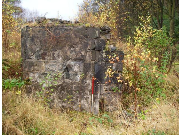
Plate 4. East facing plastered/harled wall with stone door jamb at its northern end, Alva House (Photo 15).
