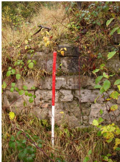
Plate 1. Wall construction of central pedimented bay of south facing façade, showing band of dressed sandstone blocks, Alva House (Photo 36).
