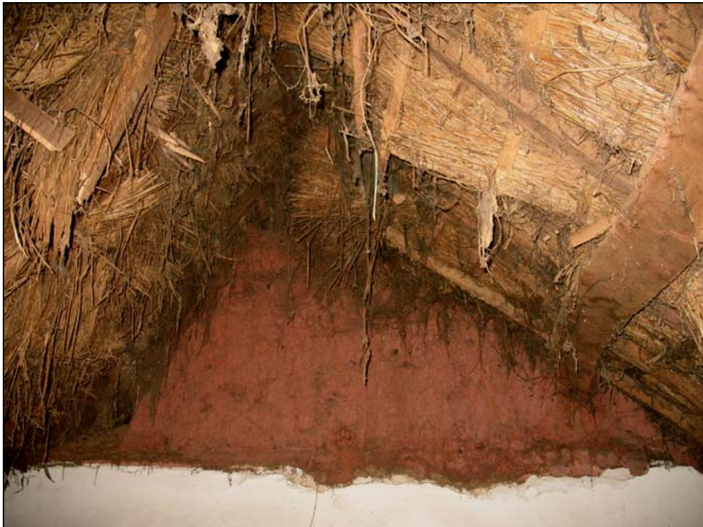
Figure 16: The west gable prior to work, from the east.
