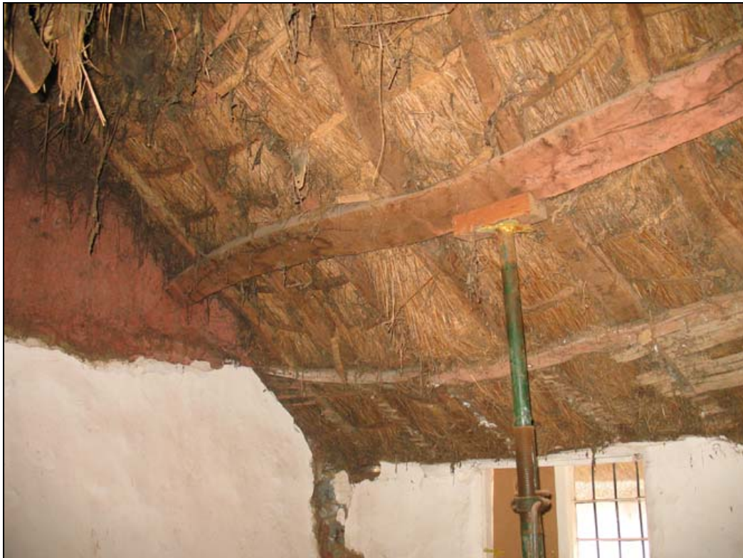
Figure 18: The western end of the north pitch, from the south-east.
