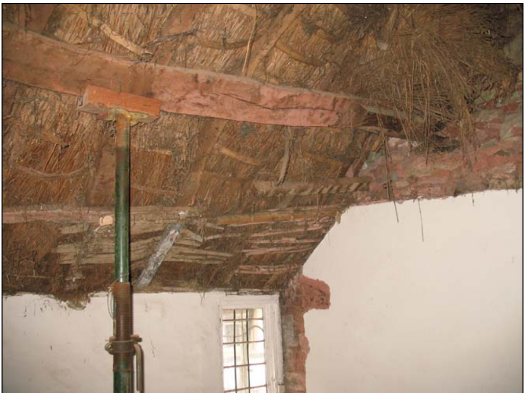
Figure 20: The eastern end of the north pitch, from the south-west.
