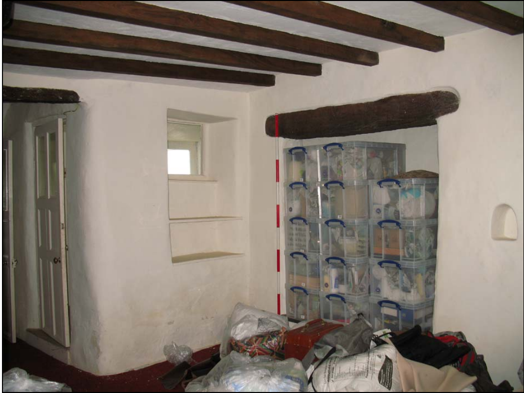
Figure 10: Interior ground floor south-west corner, viewed from the north-east.
