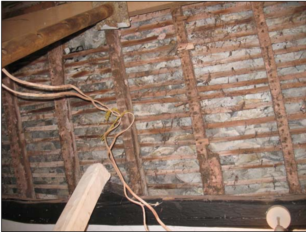
Figure 15: The stair lobby roof after removal of the interior ceiling, from the north.
