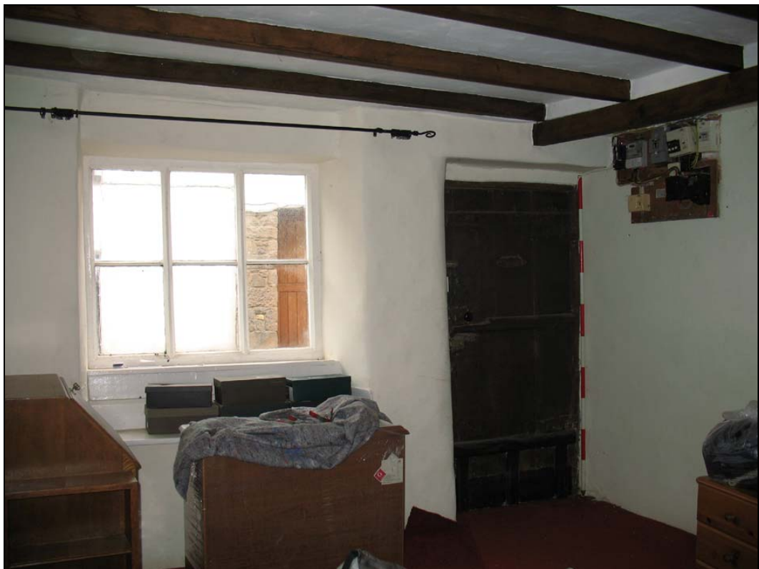
Figure 9: Interior ground floor north wall of 24A, viewed from the south-west.
