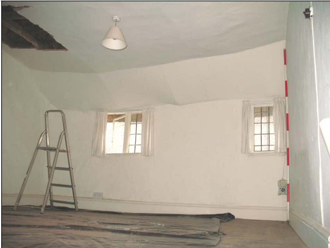
Figure 13: The first floor north wall, viewed from the south-east.
