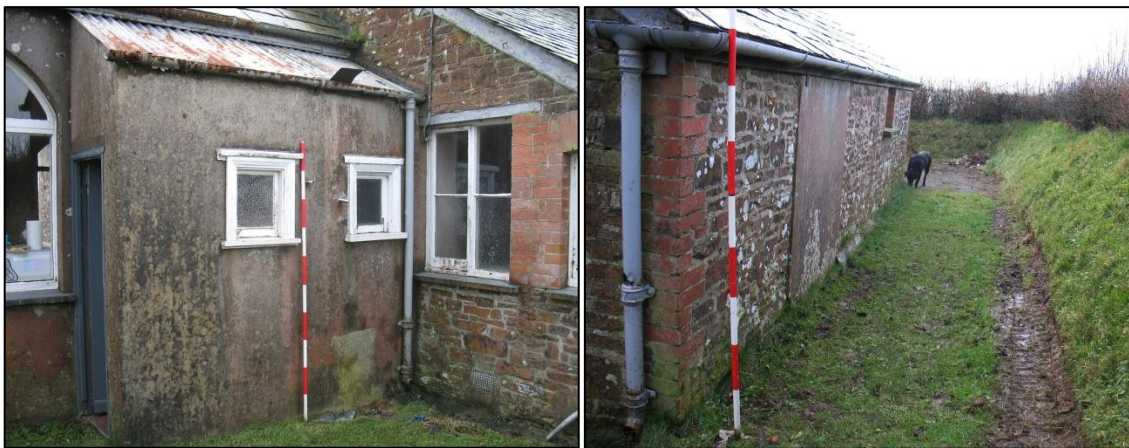
Figure 28: Left: Toilet Block, viewed from the northwest (2m scale).
