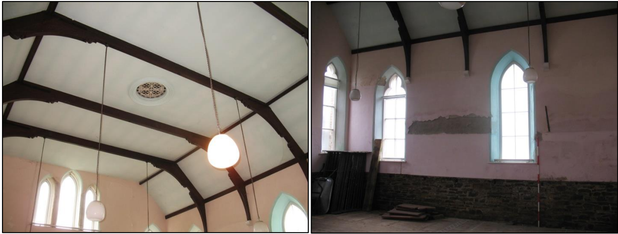
Figure 38: Left: Hall roof structure, with central vent, viewed from the northwest.
