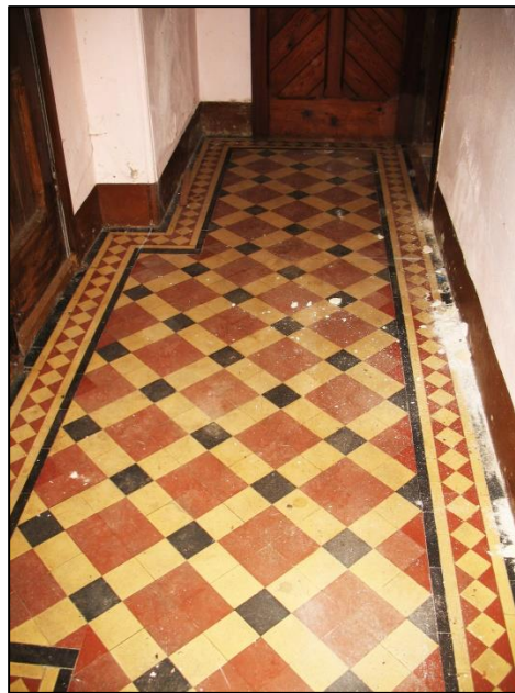
Figure 34: Detail of Vestibule floor, viewed from the north.
