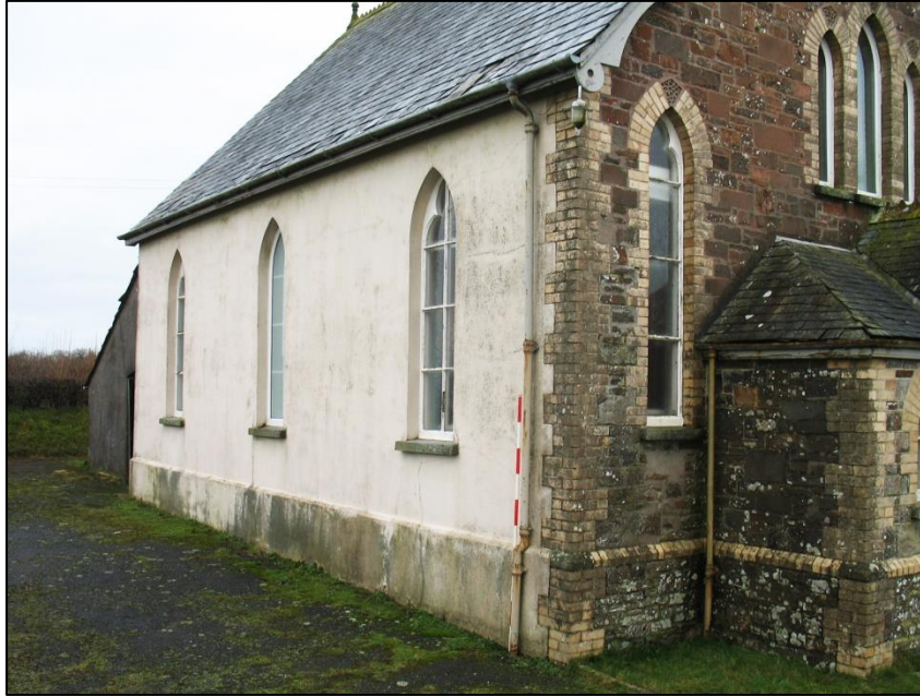
Figure 17: South elevation of the Chapel Hall, viewed from the southeast (2m scale).
