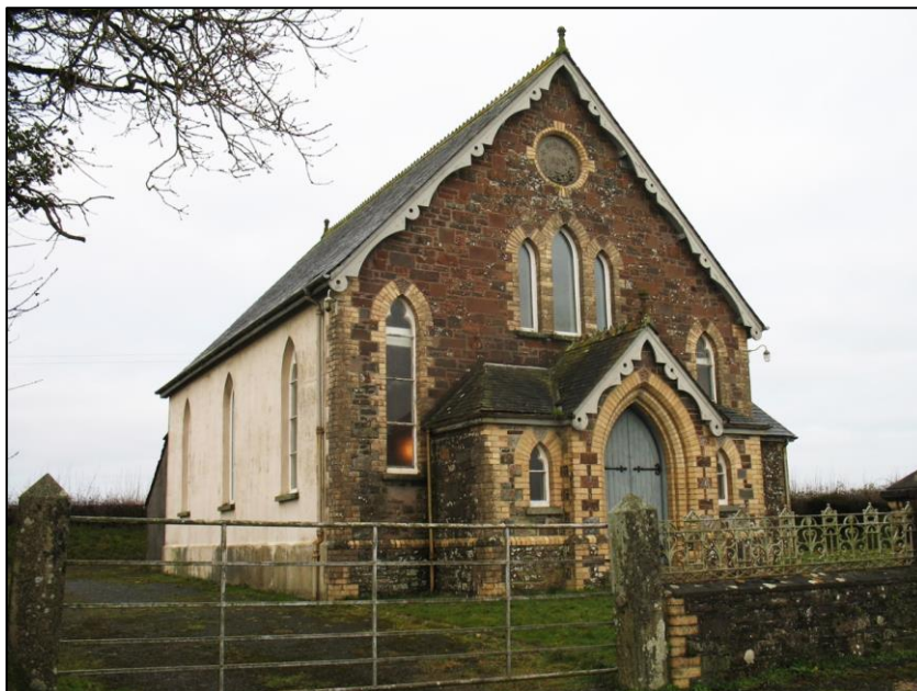
Figure 16: The Chapel Hall, viewed from the southeast.
