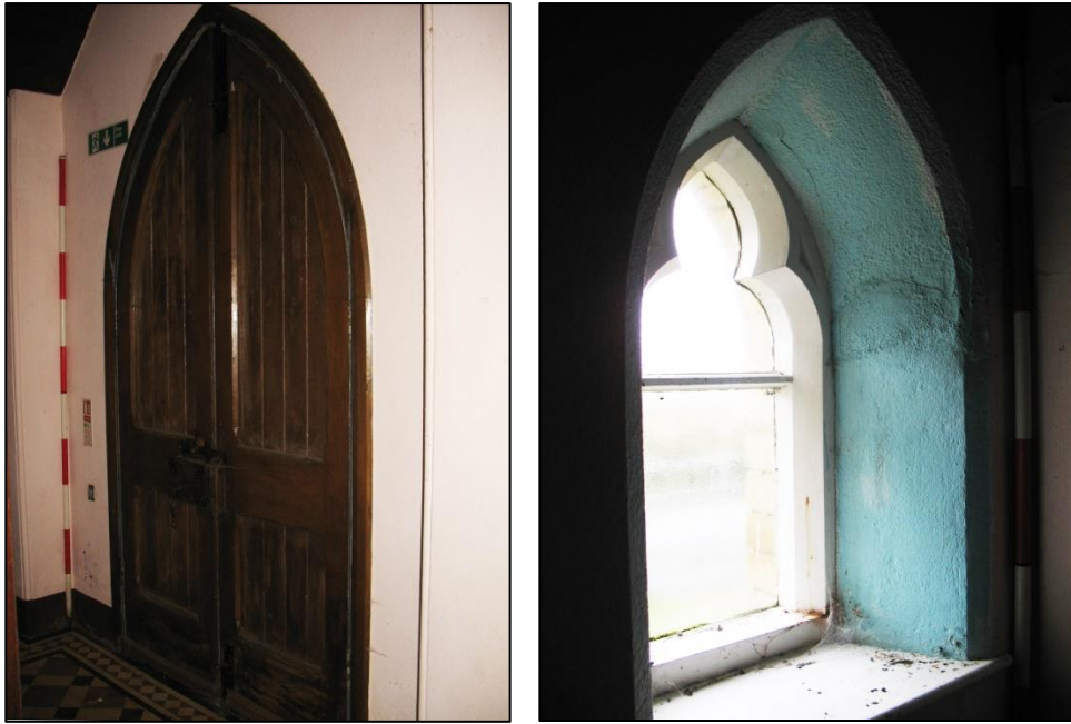
Figure 32: Left: Entrance door into Vestibule, viewed from the southwest (2m scale).
