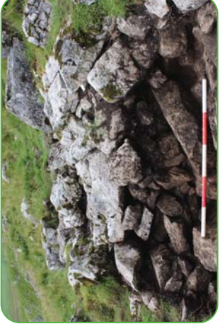
Plate 7.5 - West-facing photograph of south wall [2004]
