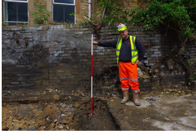
Figure 3.1 North-west facing showing existing above ground boundary wall and grubbed foundation
