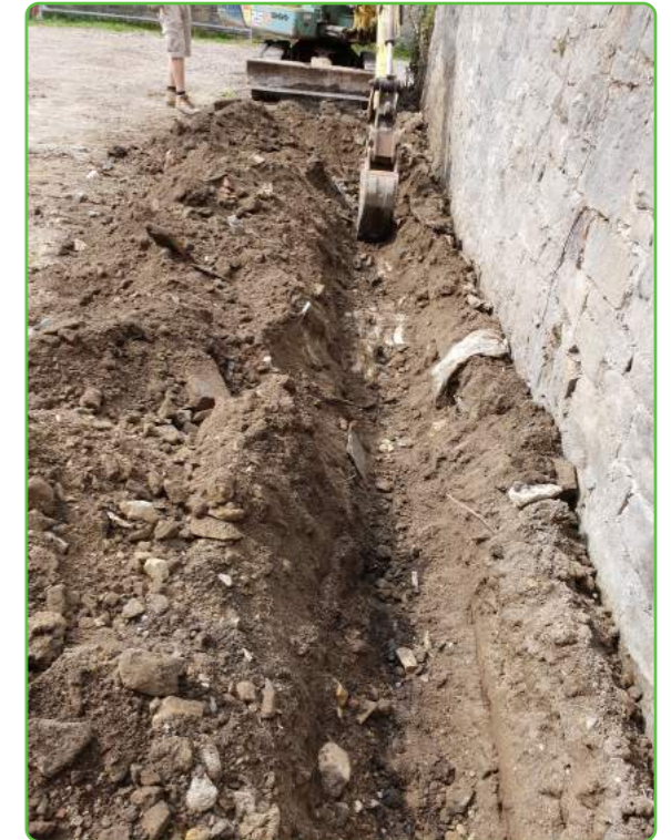
Detail of drainage pipe trench along the northwestern boundary of the site, facing southwest
