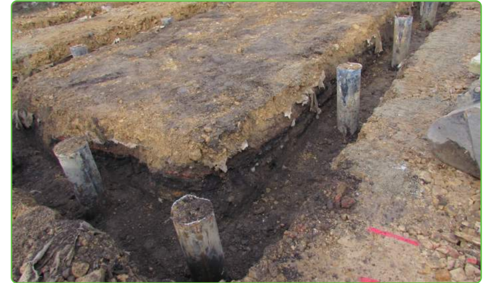
Following excavation of the foundation trenches, showing piles 22, 24, 25 and 26. Facing north
