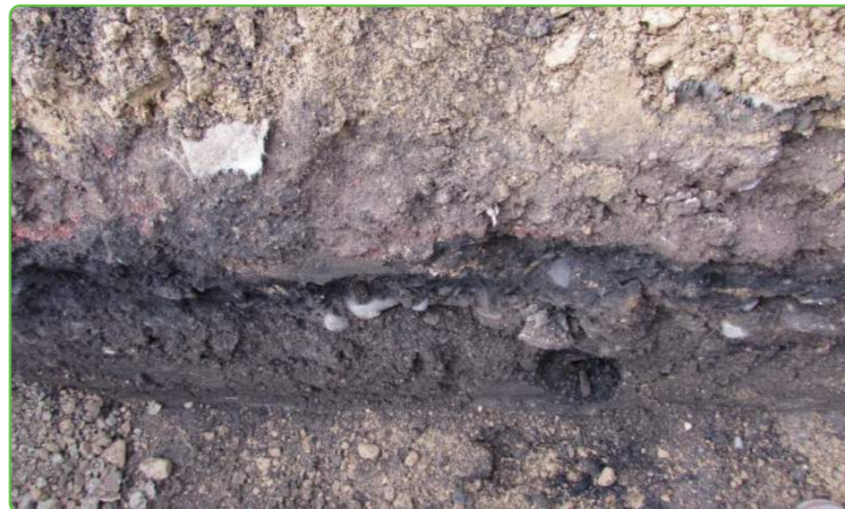
Detail of the section between piles 24 and 25, facing north
