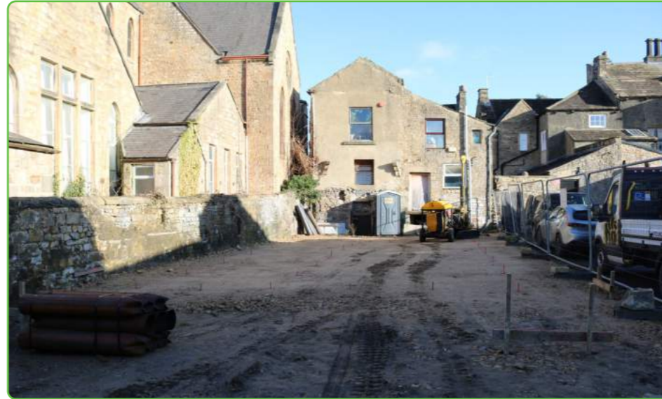
The Site, facing NE and showing location of piles
