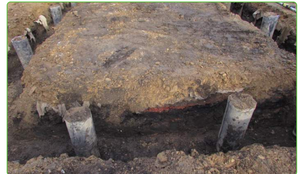
Following excavation of the foundation trenches, showing piles 21 and 22. Facing northeast
