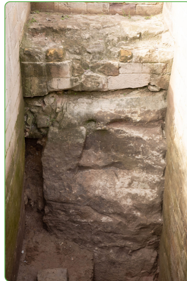
Post-ex photo of bedrock and casing wall
