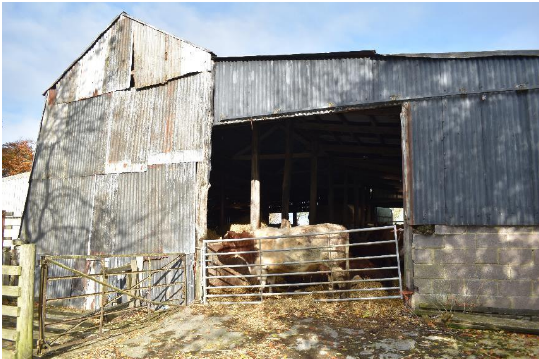
Plate 14: Pole Sheds (Cow Shed) looking north
