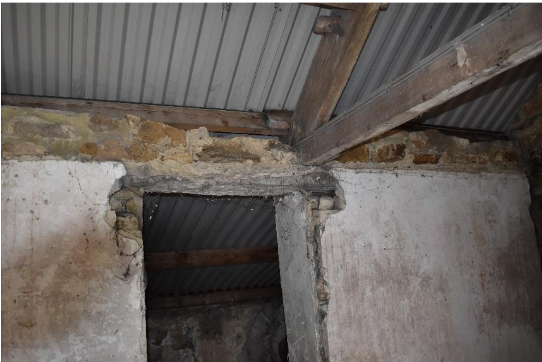
Plate 36: Granary First Floor Door Detail
