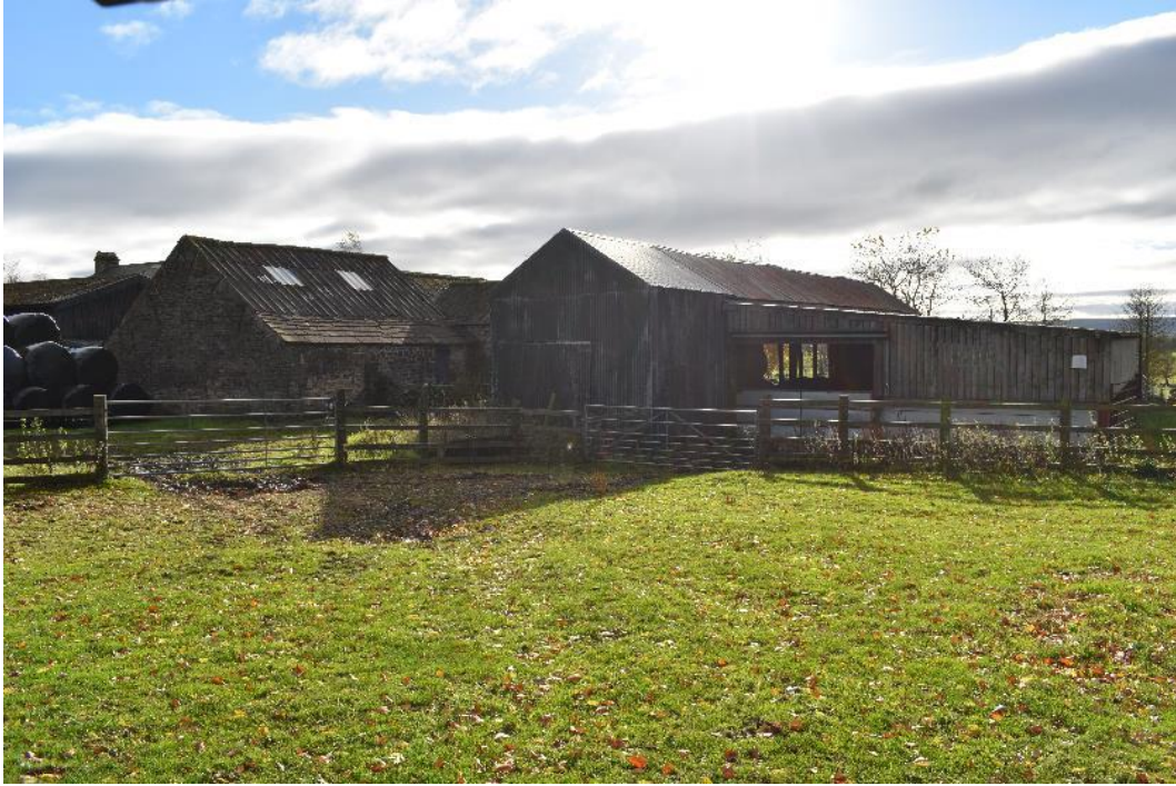
Plate 17: Pole Sheds and Workshop looking South East
