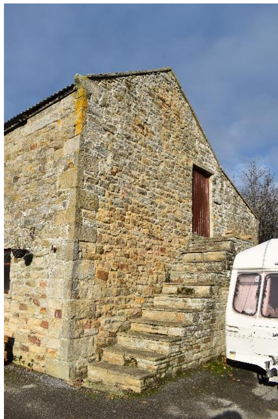
Plate 4: External stair to Granary
