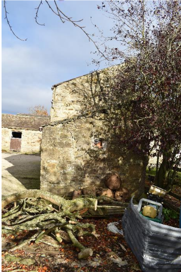
Plate 11: WC and Store looking north.
