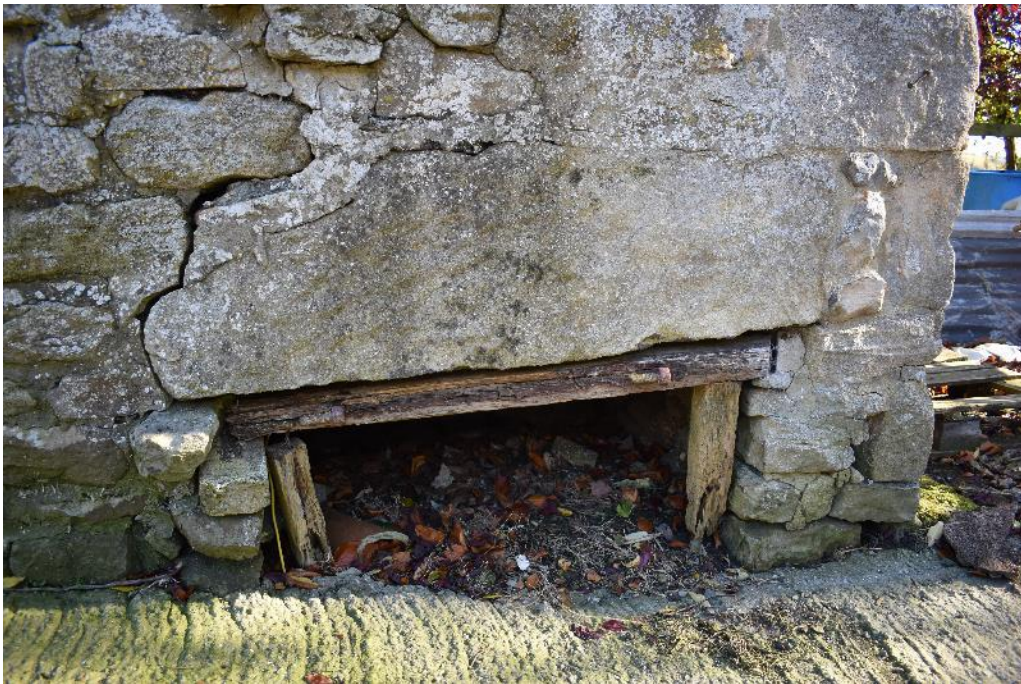
Plate 30: Detail to Toilet drop
