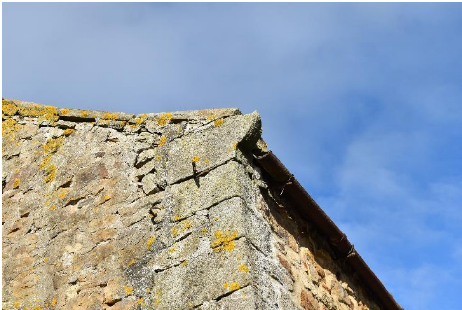
Plate 22: Corbel detail to Loose Box
