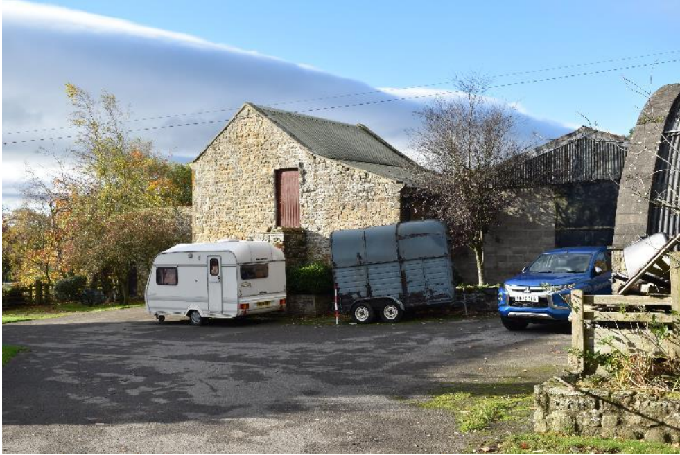
Plate 1: Approach from track to Granary.
