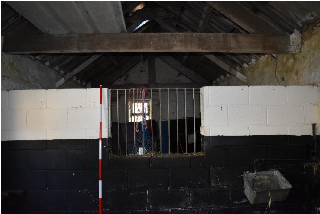
Plate 65: D3 – Milking Shed looking South.
