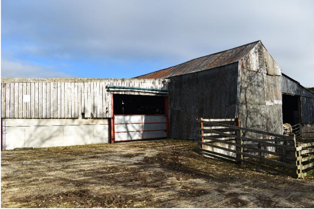
Plate 15: Pole Sheds looking North East
