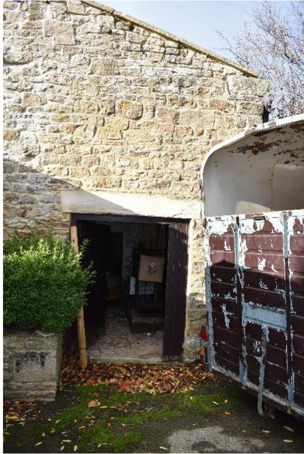
Plate 7: Granary entrance door detail
