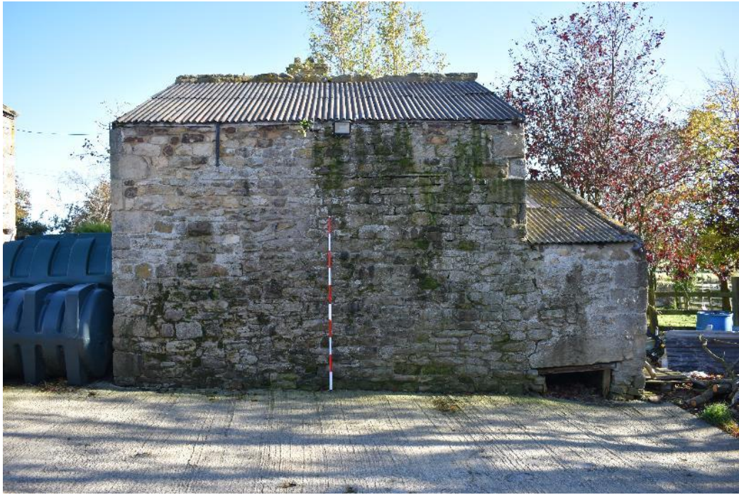
Plate 29: Store/WC Looking East
