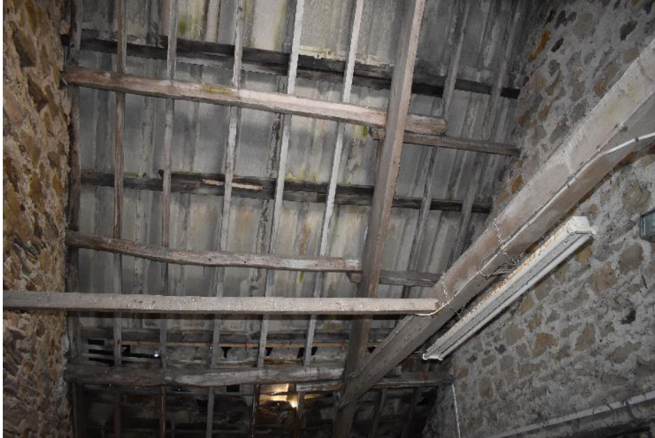
Plate 56: Workshop Roof Detail
