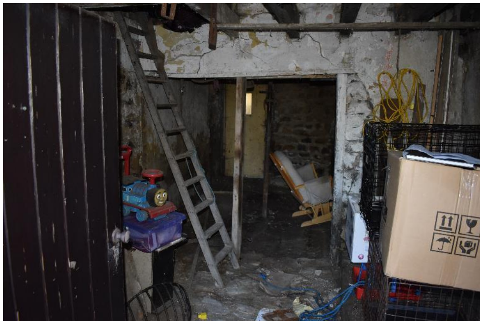
Plate 32: Granary Entrance Room.
