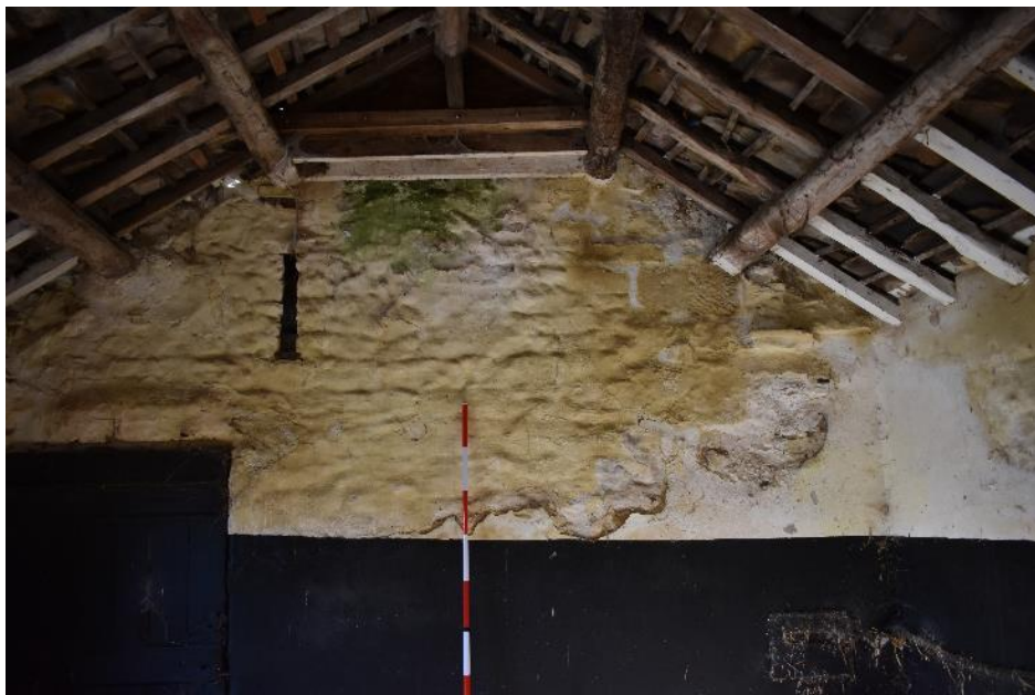
Plate 42: Stables looking West
