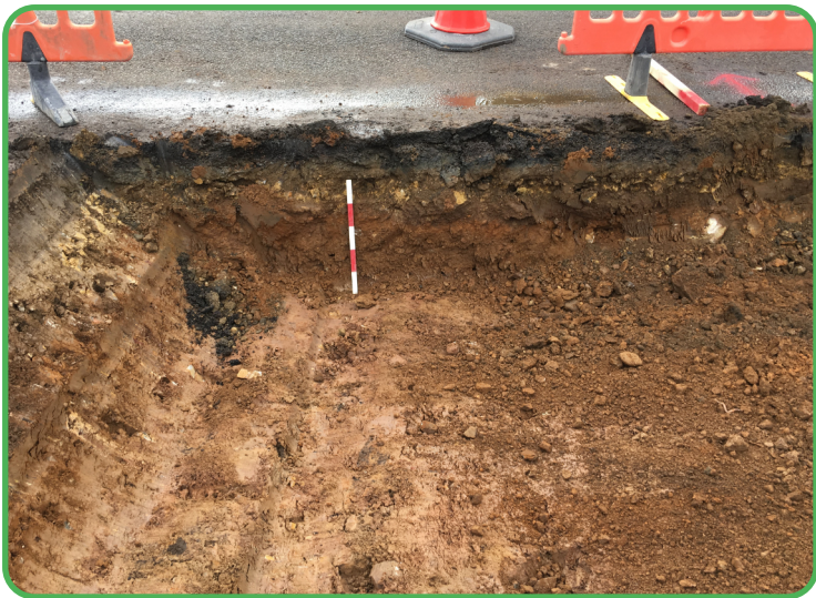
Section 02, section in existing modern road layers, facing NE
