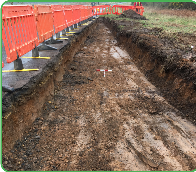
Plan view of slip road facing NW
