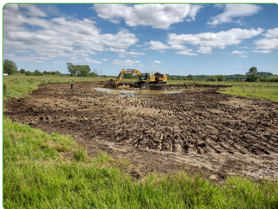
Monitoring in Church Farm - Facing SE
