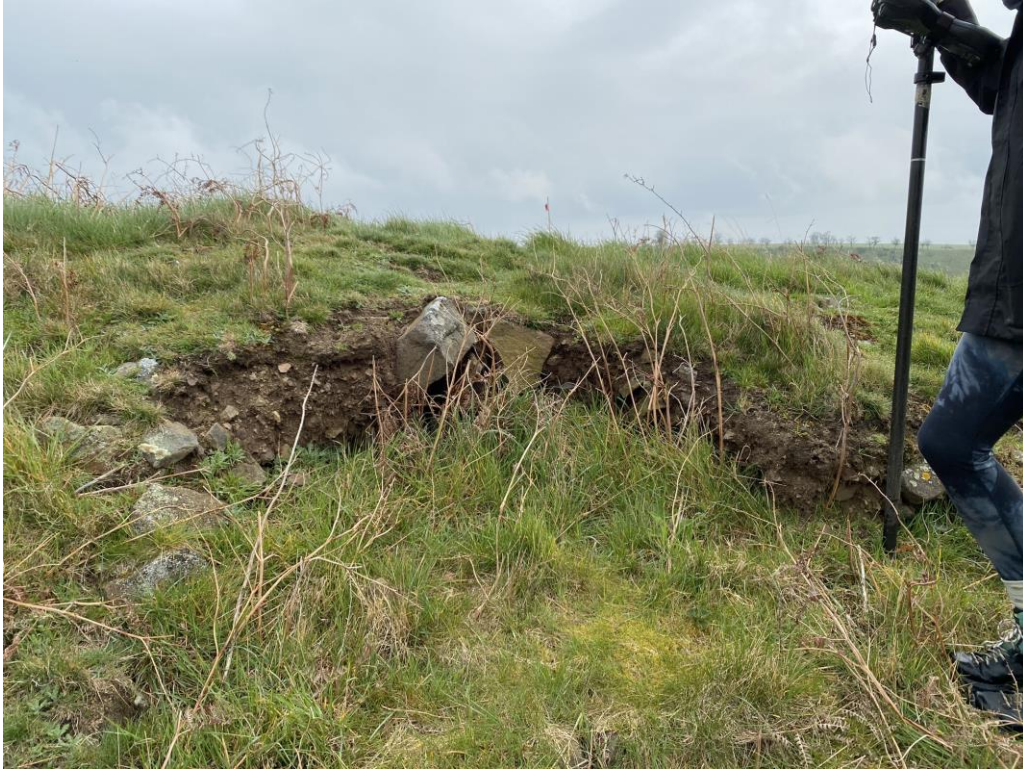
Plate 11: An area of erosion on the north-western outer banks of the hillfort, showing the exposed stones forming the makeup of the banks
