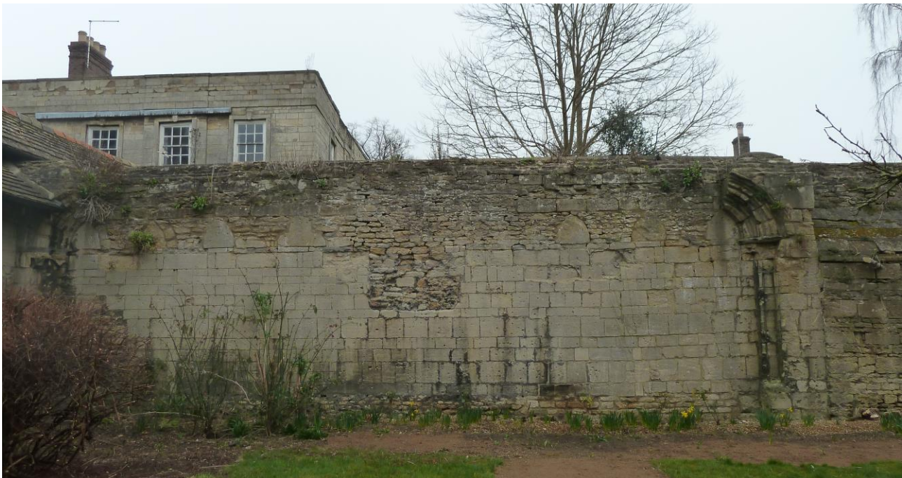
Fig 3: Northernmost section of 'Wall 17', west side, interior of medieval refectory with details of blind arcade and later refacing and repairs (taken March 2015)
