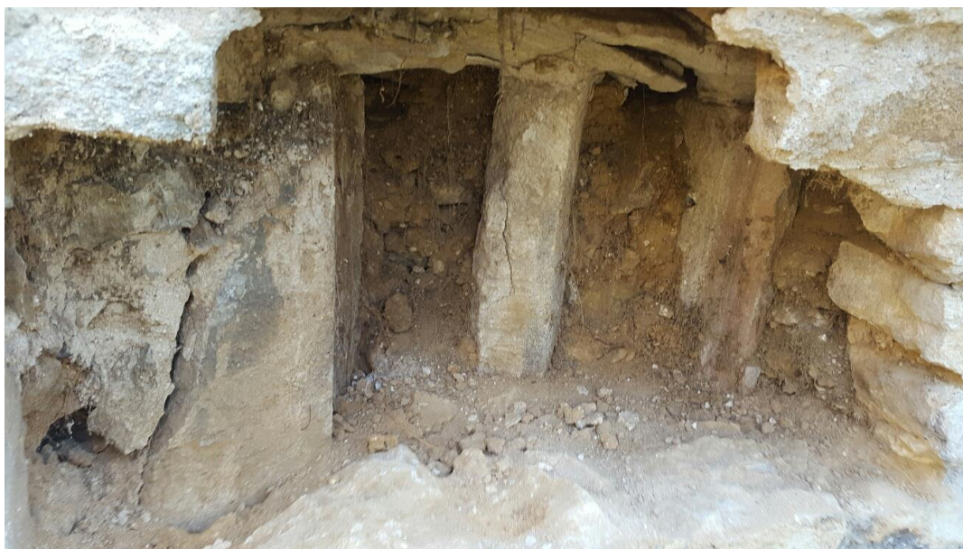
Fig 22: Partially unblocked window in centre of refectory east wall (Julian Vosper)
