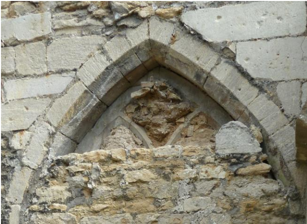
Fig 23: Bay 8, with upper blocking removed, showing the blocking of three quatrefoils from which mortar samples were taken
