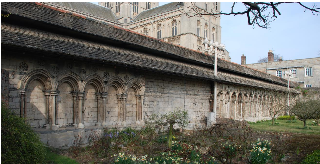
Fig 5: North wall of refectory (taken March 2009)
