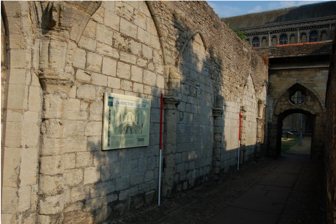
Fig 2: Northernmost five bays of 'Wall 17', east side, with 13th-century vault responds and wall ribs, looking north-west (taken July 2006)
