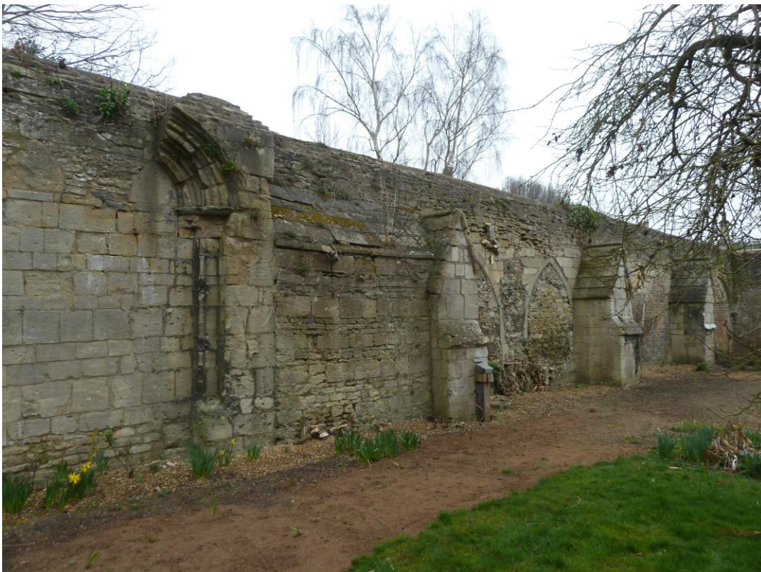
Fig 7: General view of west side, with 13th-century refectory in foreground, then bays 6–12, 14th-century covered way with gabled buttresses and numerous blockings and refacings (taken March 2015).
