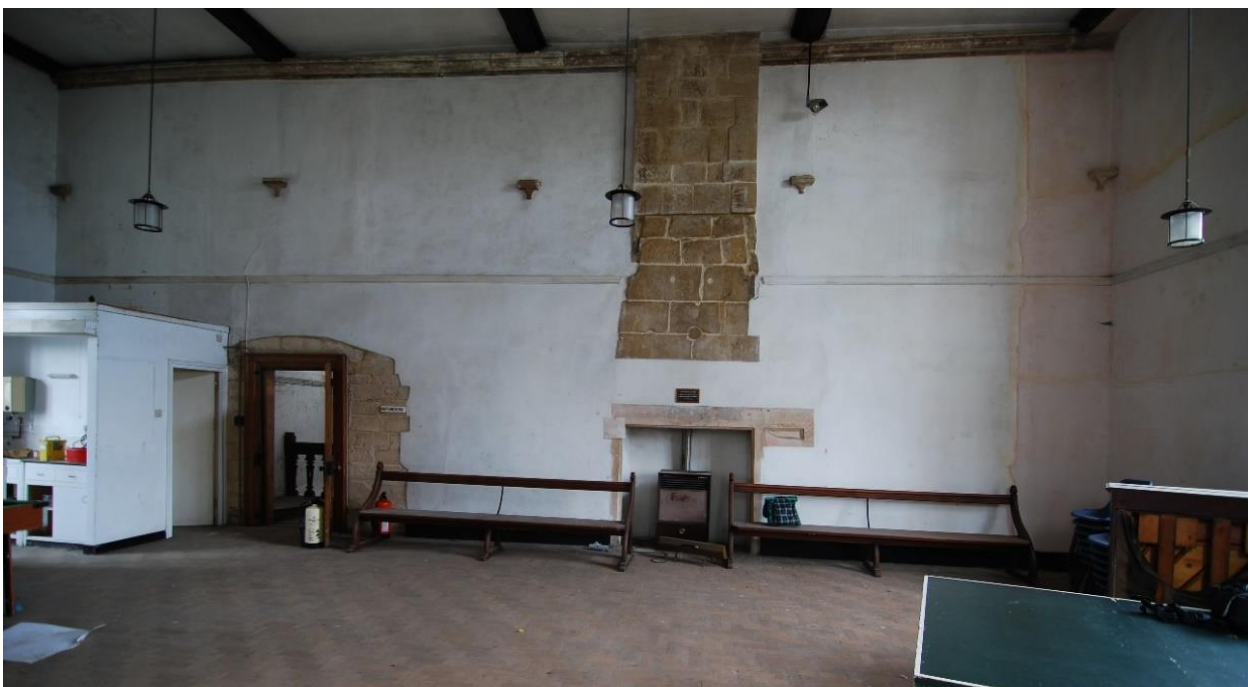
Plate 24 (Archive image PCKC 677) Knights' Chamber. West wall, showing chimney, corbels and upper cornice Photograph: Jackie Hall (2012)
