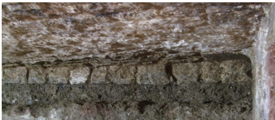
Plate 66 (Archive image: PCKC 183) Lift Foundation Trench: the northern half of footing 929 exposed at the limit of excavation. Photograph: Caroline Atkins
