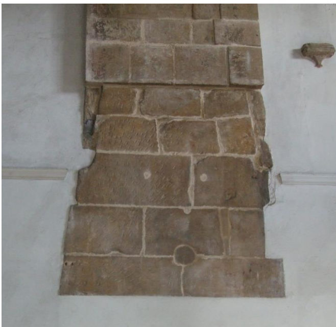
Plate 31 (Archive image PCKC 048, detail) Knights' Chamber. Detail of chimney flue, showing cut-back top of fireplace canopy with reused stones blocking flue below Photograph: Caroline Atkins
