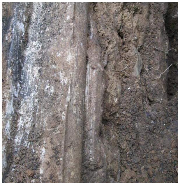
Plate 58 (Archive image: PCKC 026) Trial Pit 2: keeled moulding capping offset footing. Photograph: Caroline Atkins
