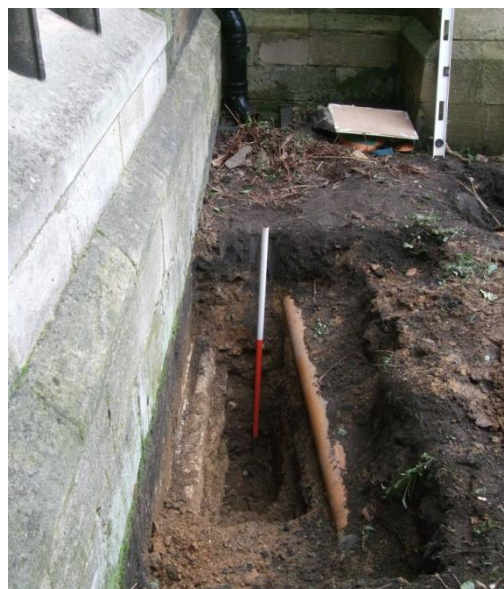
Plate 56 (Archive image PCKC 016) Trial Pit 2: the offset footing. Photograph: Caroline Atkins
