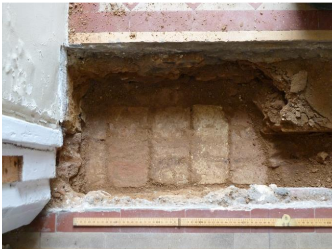
Plate 86 (Archive image PCKC 715) No. 25. Threshold, brick floor, before removal. This was set on a brown clay-based bedding layer Photograph: Jackie Hall
