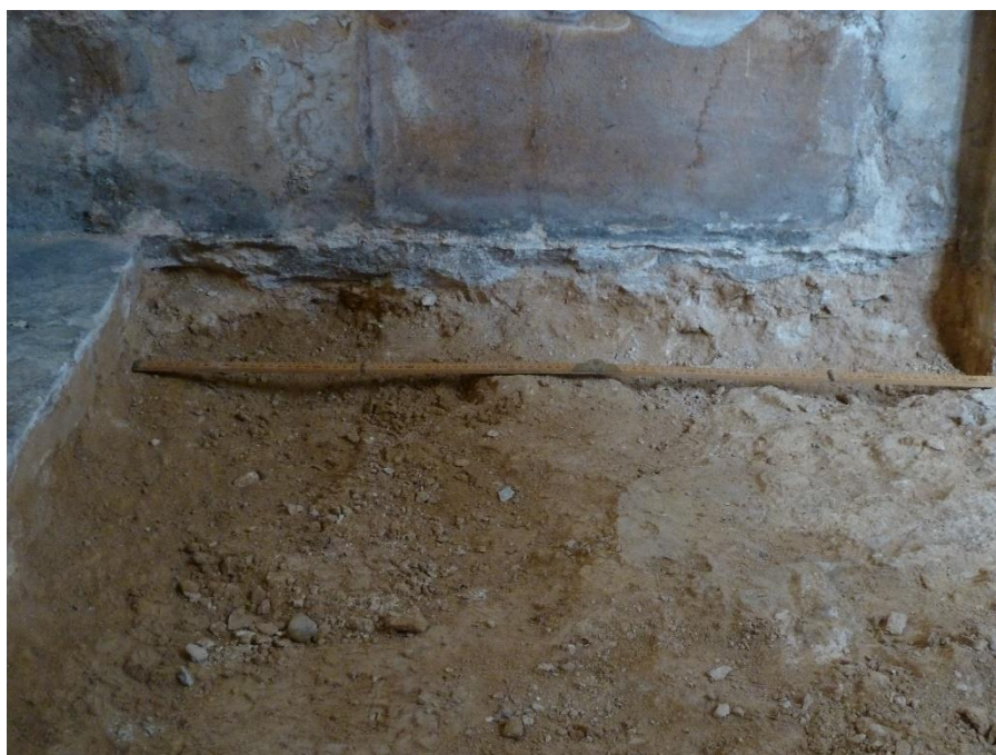
Plate 7 (Archive image PCTAR 45) Section at north-east side of apse step; buff mortar upper and right; sand and rubble lower and left Photograph: Jackie Hall
