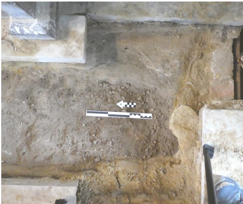
Figure 11: South end of south aisle-nave trench, after further investigation. Parts of mortar floors have been removed, and the loose grave fill can be seen. All of these are cut, on the south side, by the trench made to create the brick-lined duct (scale = 0.30m)
