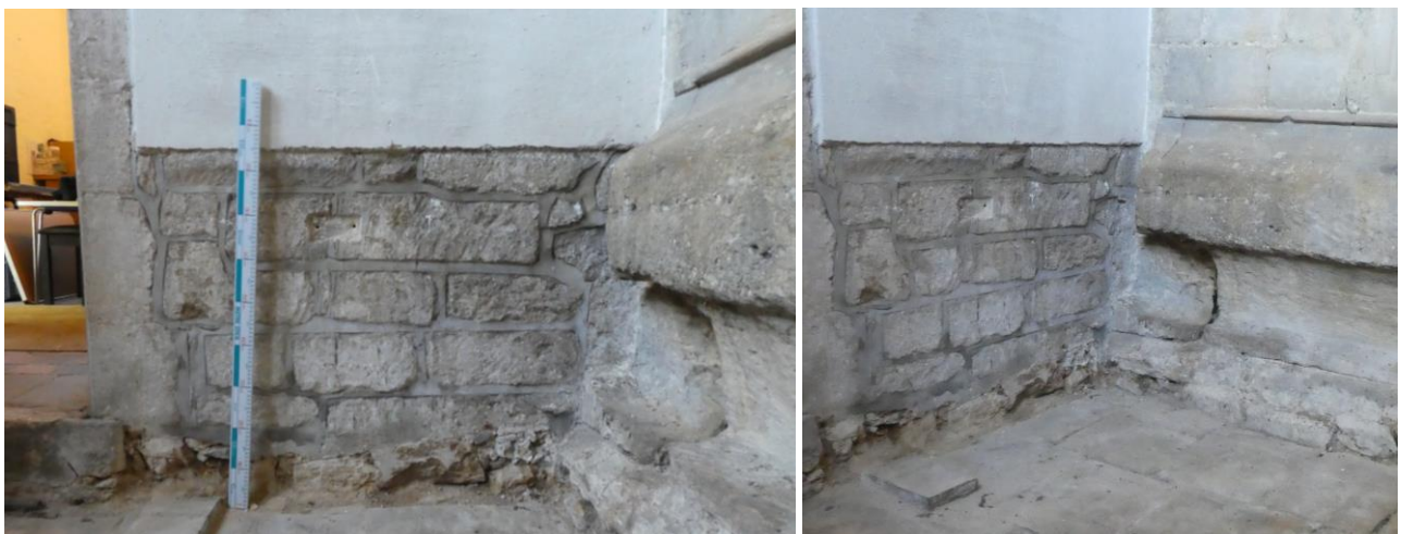
Figure 18: East wall of north chapel, temporarily exposed; foundations and earlier external wall of chancel can clearly be seen (scale = 1m)
