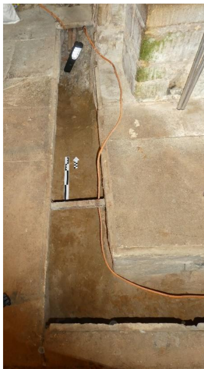
Figure 4: Duct in tower, after cleaning, looking north (scale = 0.30m)
