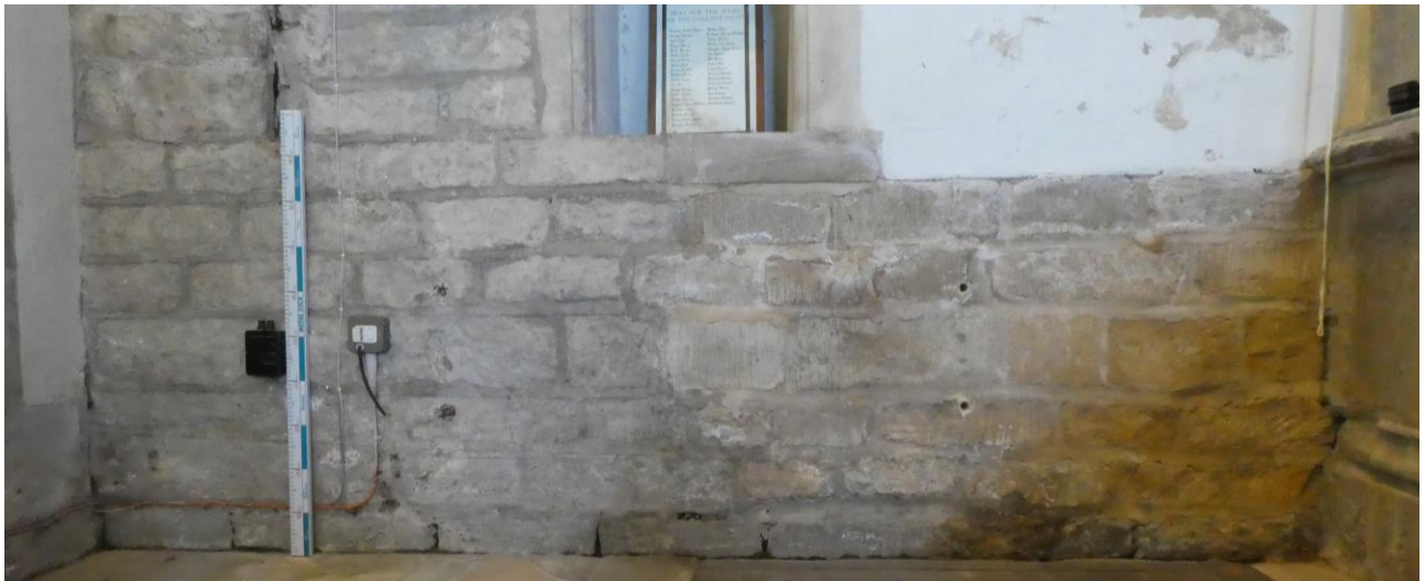
Figure 17: South wall of south aisle, temporarily exposed (scale = 1m)
