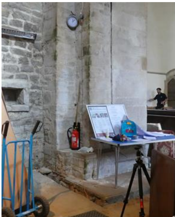
Figure 3: General location of duct in tower, looking north-east
