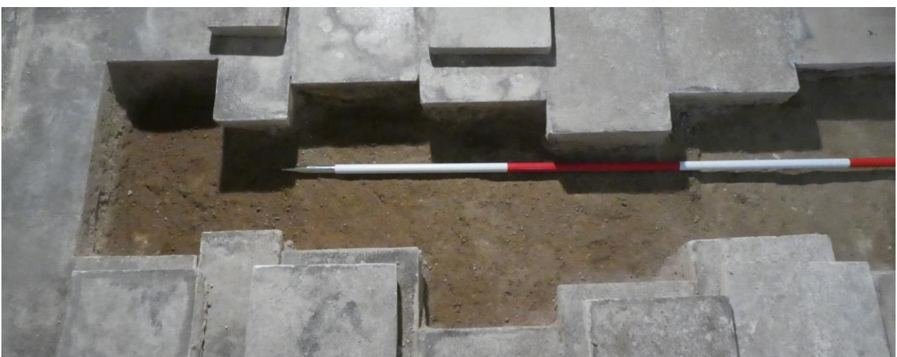
Fig 12: Deposits in the open area, bounded by foundations and sleeper foundations – here in area E, looking east. The grey area on the right side probably indicates an area of deeper limecrete bedding here
