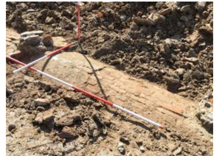
Fig. 8 Central part of conduit looking south west.
