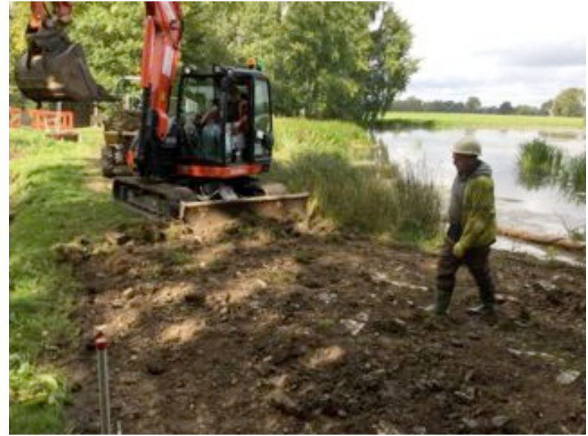
Fig. 4 Work to strip the topsoil begins, view looking west.
