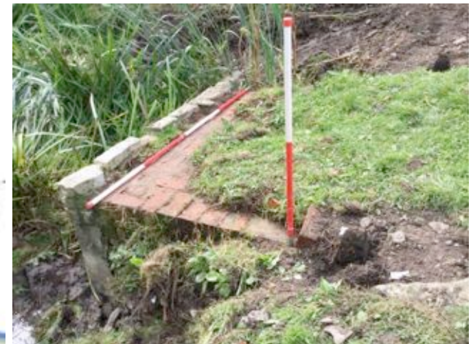
Fig. 9 Brick pier with stone edging looking south west.
