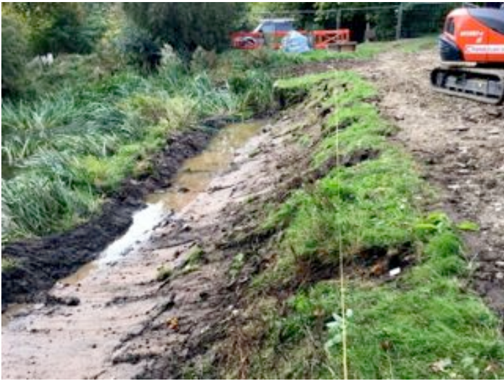
Fig. 11 Line of posts looking west.
