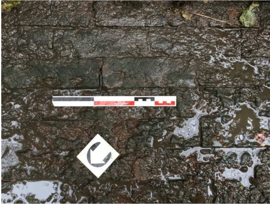
Fig. 21 Detail of brick lining to channel.
