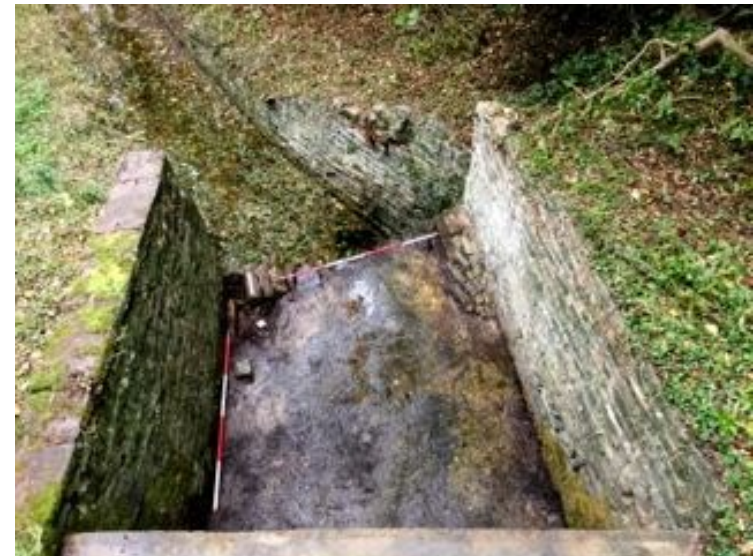
Fig. 12 Channel approaching lip of weir 2 with flanking walls and remains of pitched stone base looking south east.
