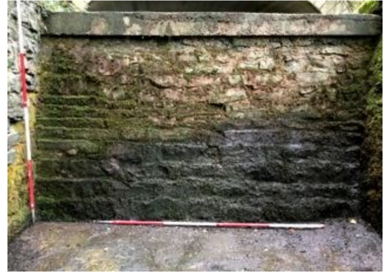
Fig. 11 Weir 1 showing repair and diminishing courses of original work looking west.
