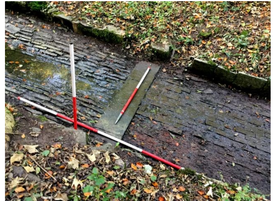
Fig. 16 Junction between the stone and brick base for the channel looking north.
