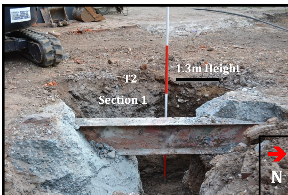
A1 – Pile Shaft T2 – West Size: 0.5m Width x 1.2m Length x 1.3m Depth With steel and concrete pad-stones from previous construction still in situ
