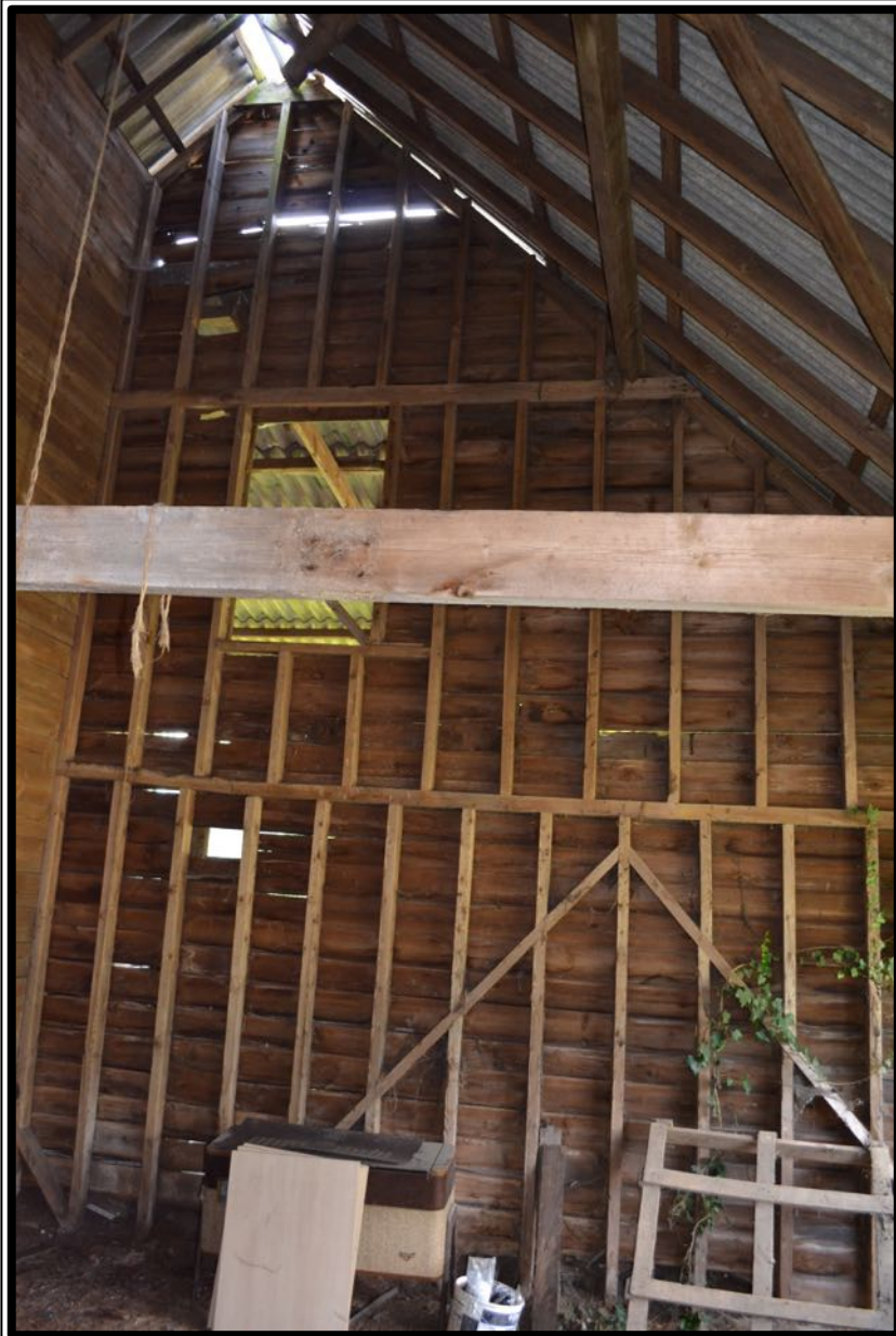
Plate 4. The Black Barn internal west elevation
