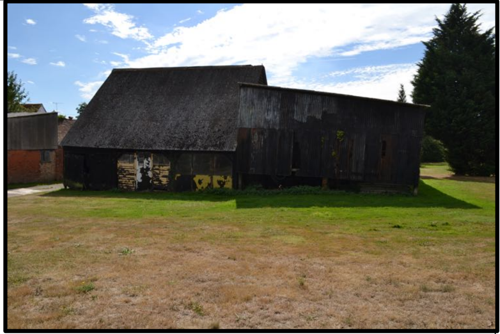
Plate 3. The Black Barn north elevation and west lean-to extension
