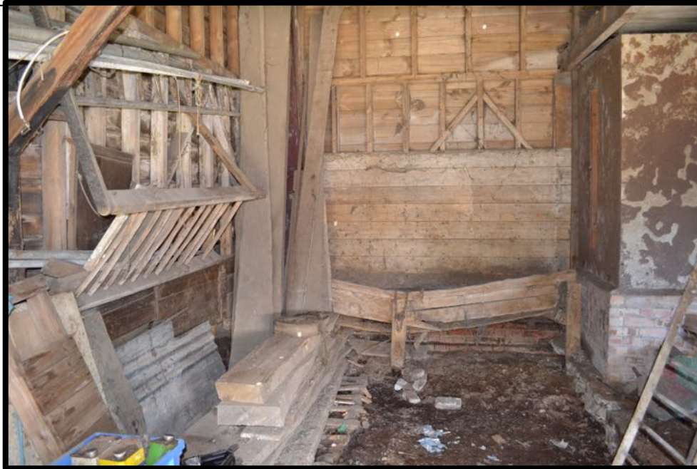
Plate 5. The Black Barn manger and feeding rack to southwest area of barn
