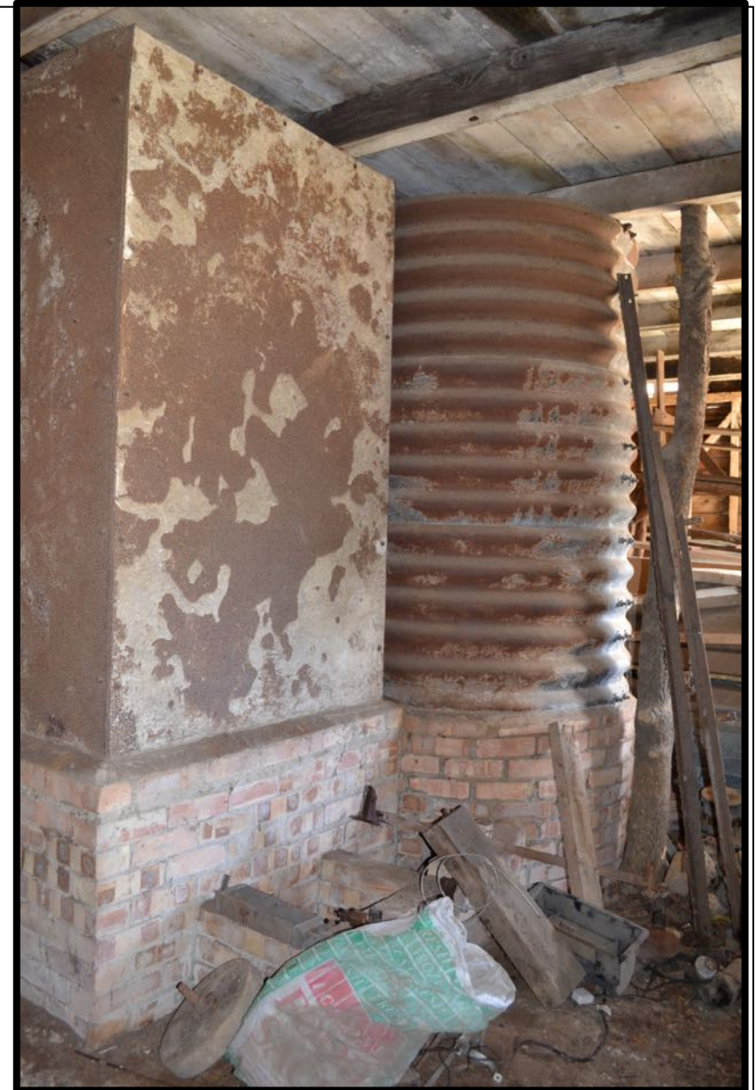
Plate 6. The Black Barn grain Silo to southeast area of barn
