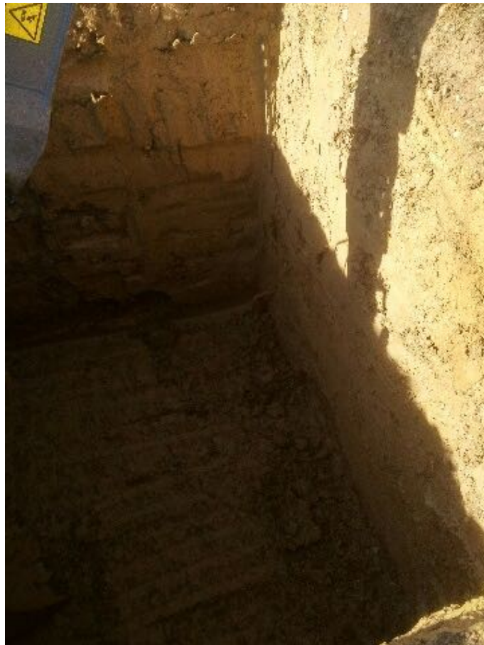
Plate 9: Foundation trench (taken by owner)
