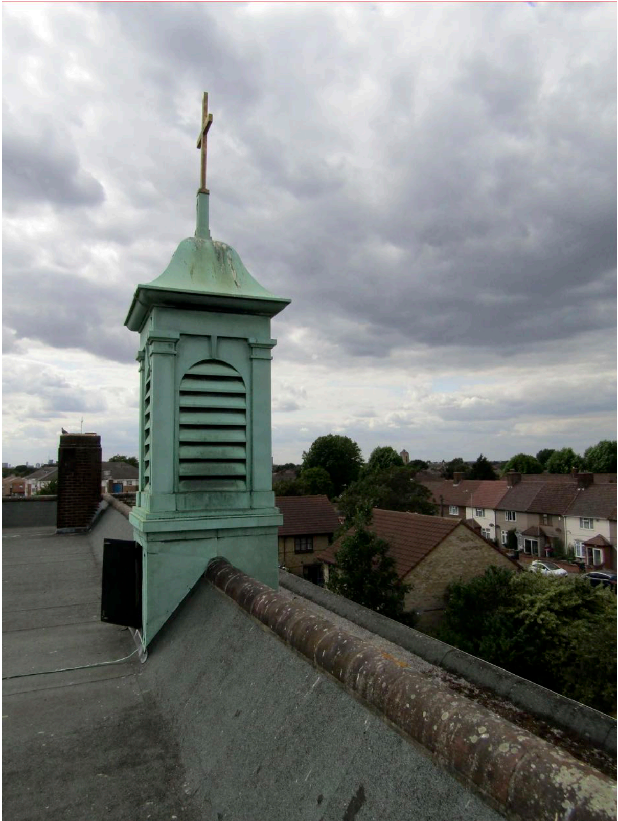
Figure 9 - roof and bell tower
