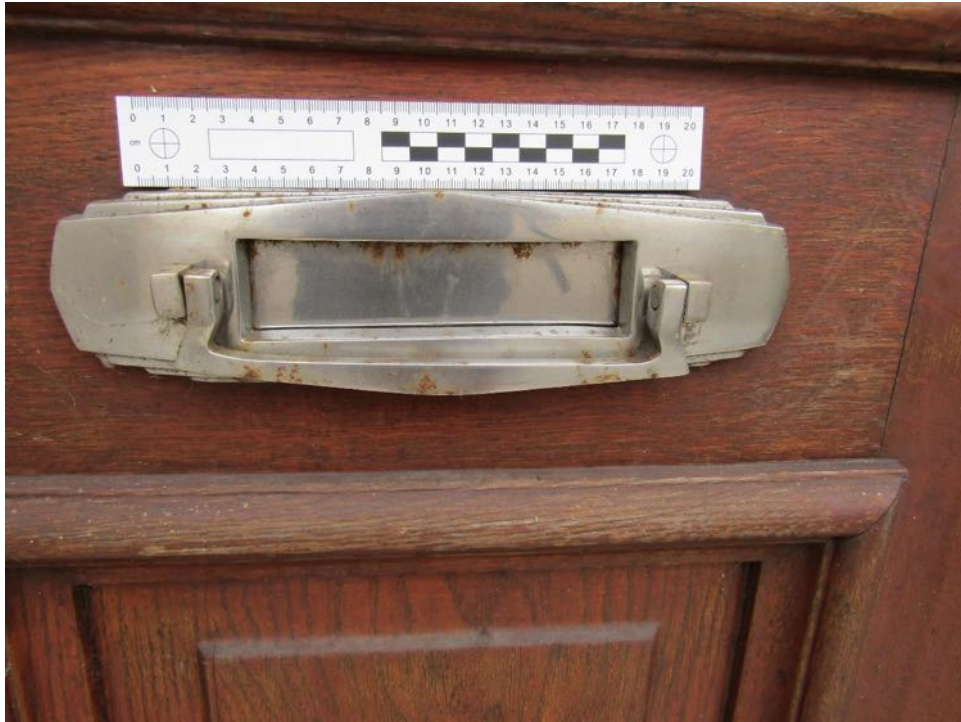
Figure 10 - front entrance door letter box
