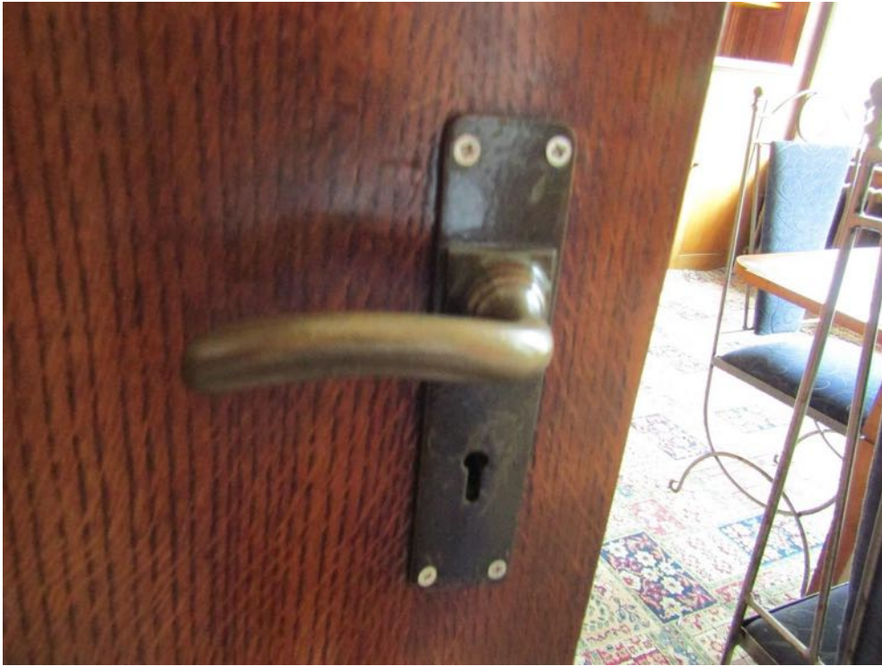
Figure 37 - original door handle (ground floor only)
