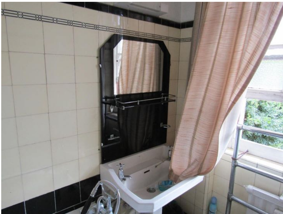
Figure 29- bathroom on first floor by communal "kitchen"
