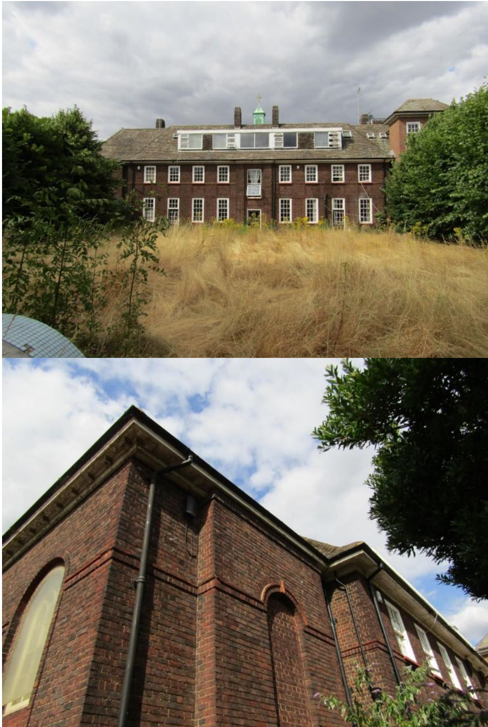
Figure 14 - detail to the rear elevation of the chapel
