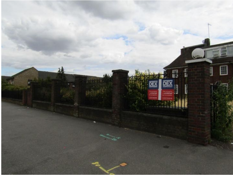
Figure 43 - front boundary wall
