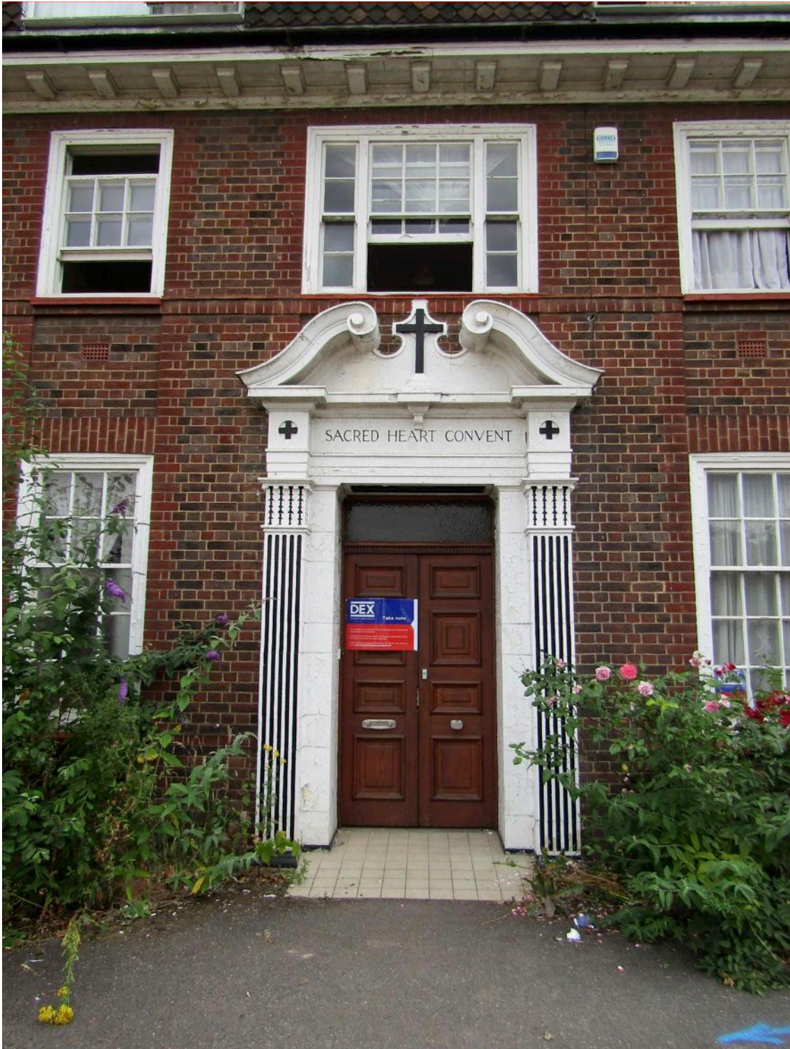
Figure 8 -front entrance door to Convert
