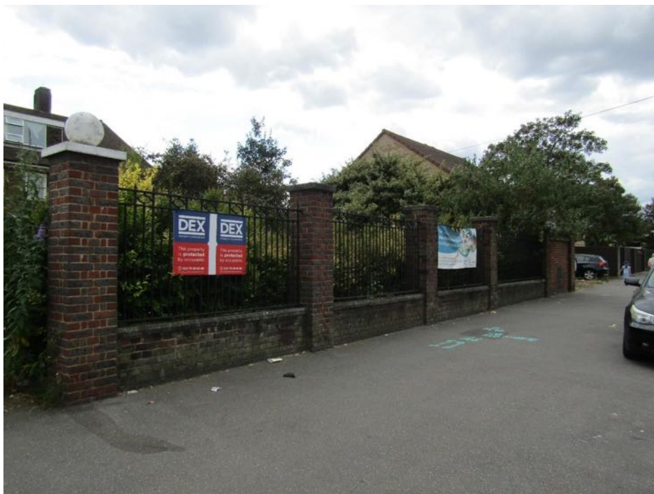
Figure 44 - front boundary wall
