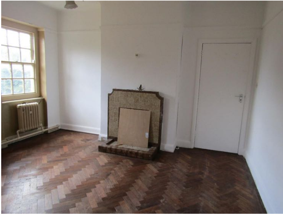
Figure 28 - communal 'Kitchen' on first floor
