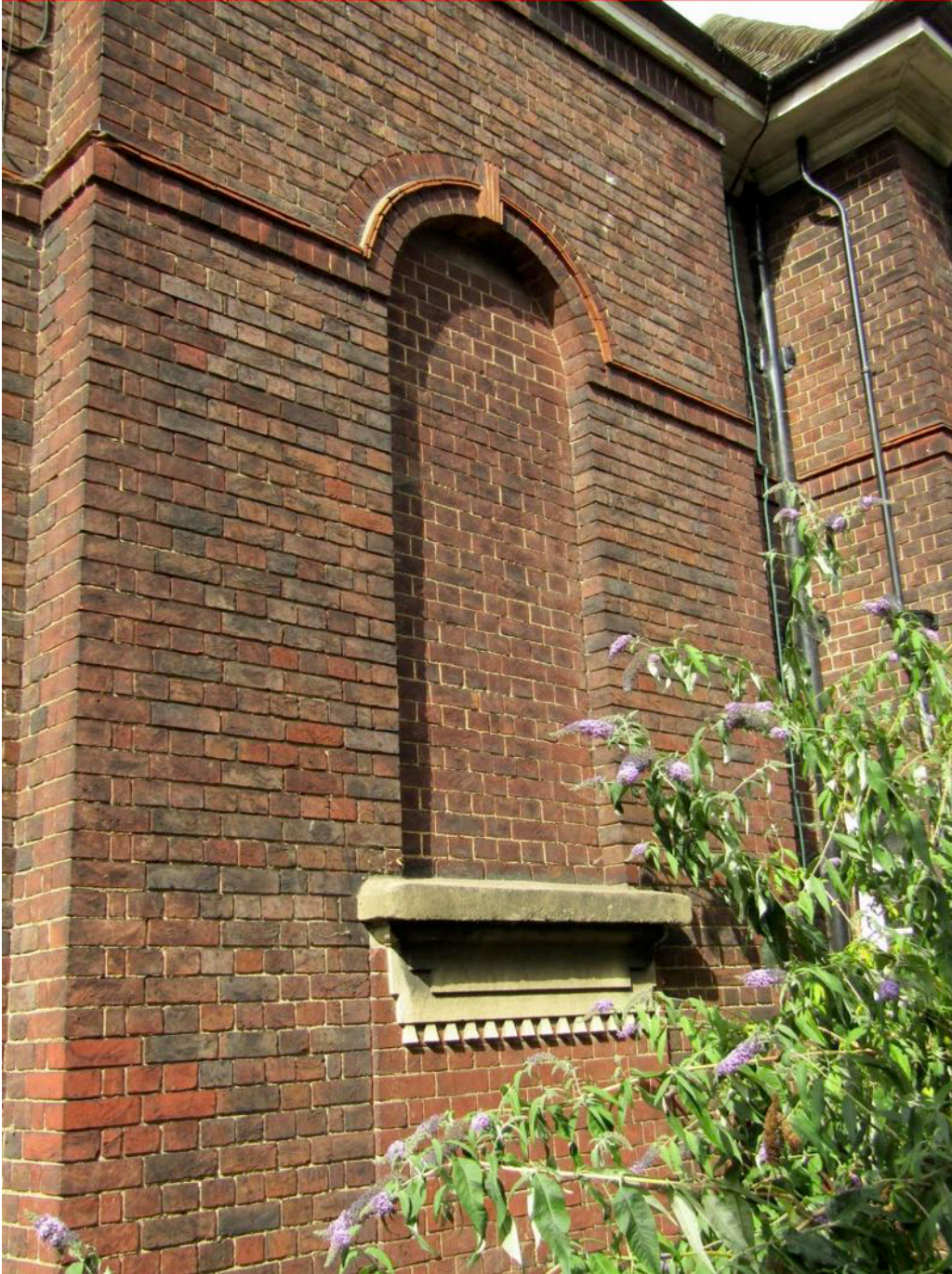
Figure 15 - detail to blind window to chapel
