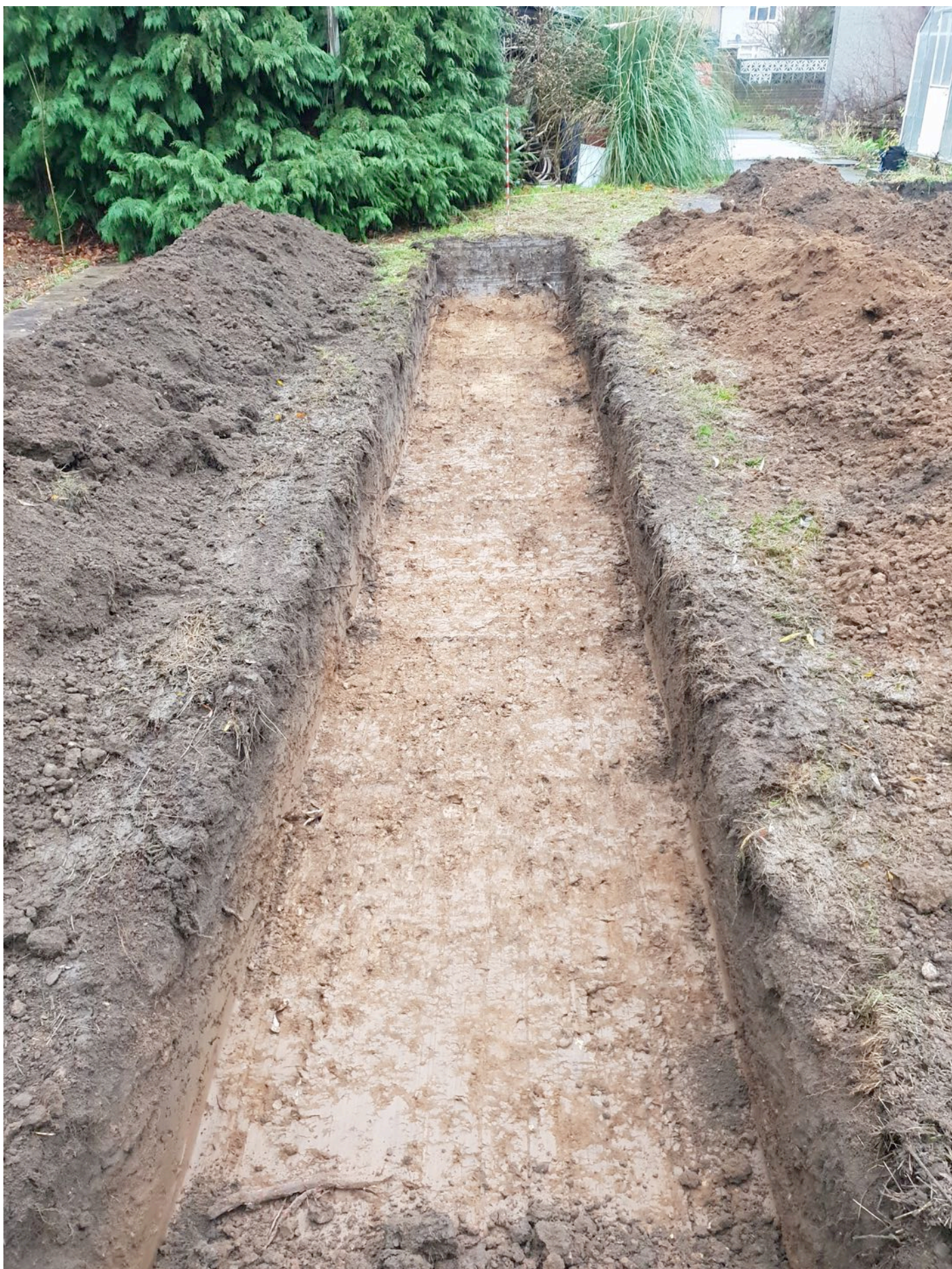
Plate 3. Trench 5 facing south
