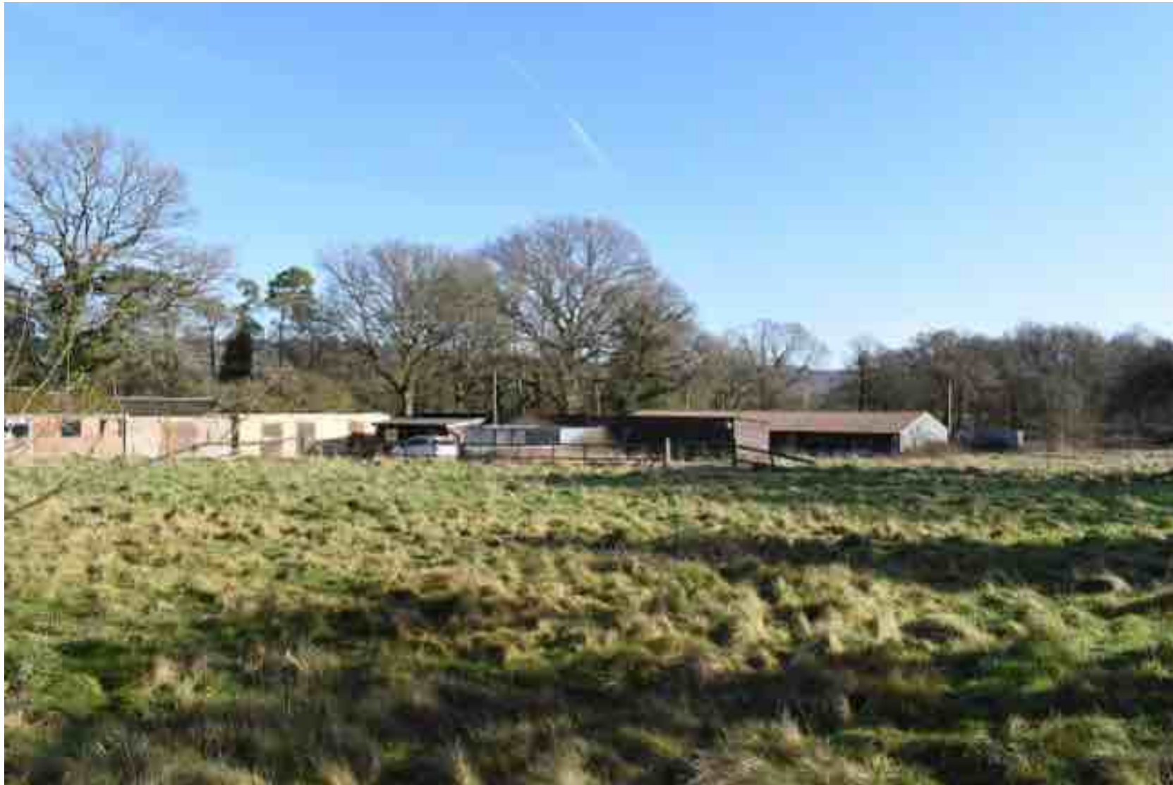
Plate 10: View across PDA from south west corner (facing NE)
