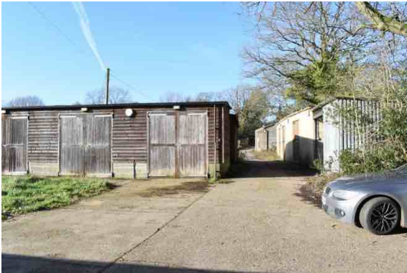
Plate 13: View along the PDA hardstanding access (facing W)
