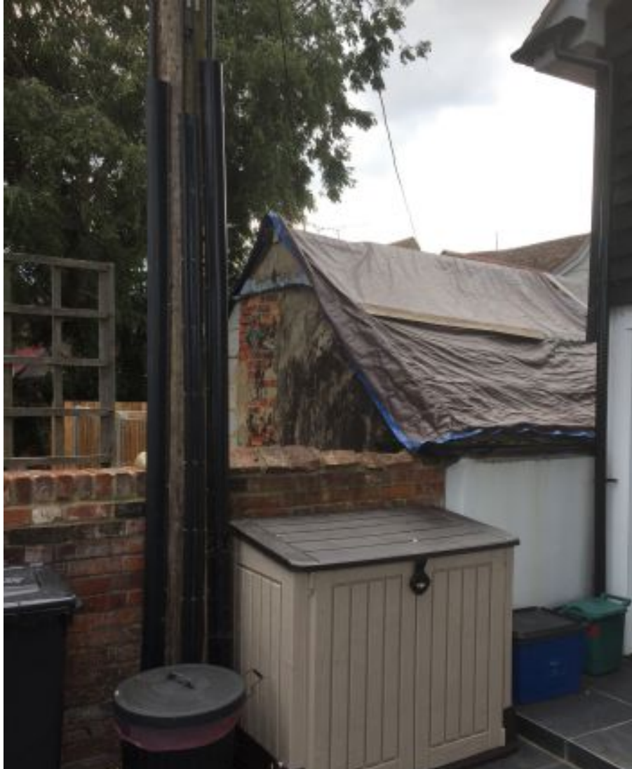
Plate 9. View of site and east elevation of extant building (facing southwest)
