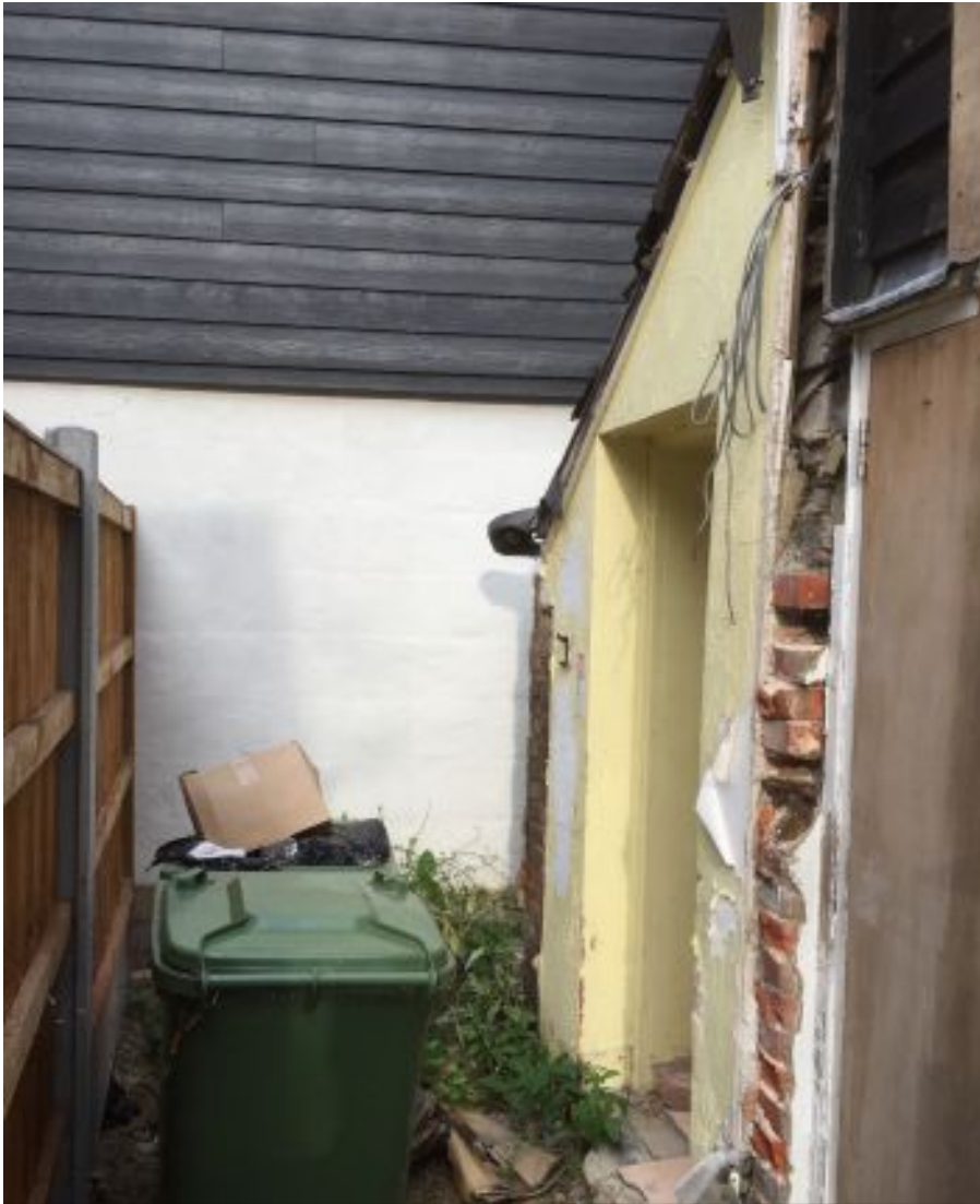
Plate 6. View of site and north elevation of extant building (facing east)
