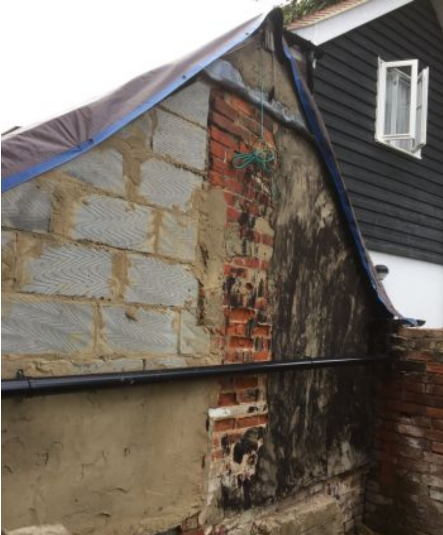
Plate 7. View of site and south elevation of extant building (facing northeast)
