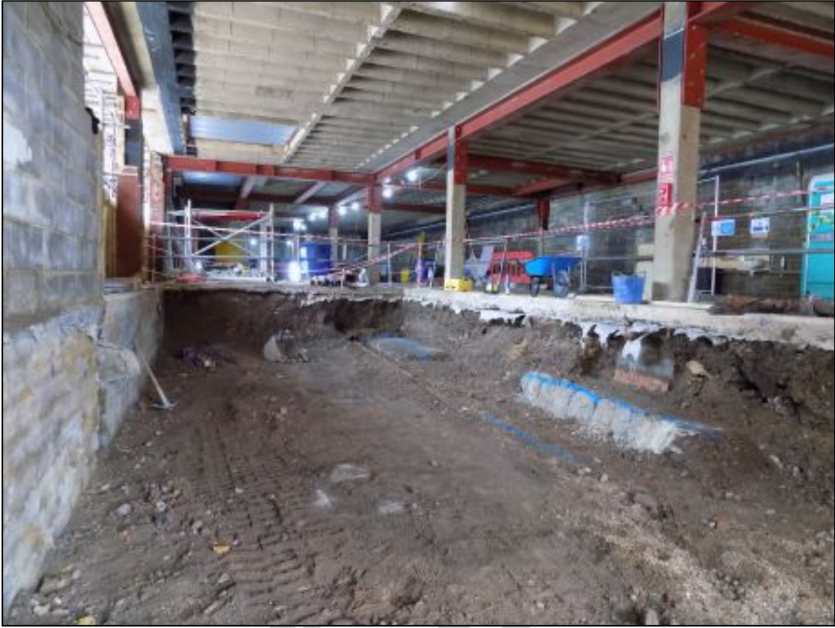
Plate 3. Site following the removal of modern sub base facing E.
