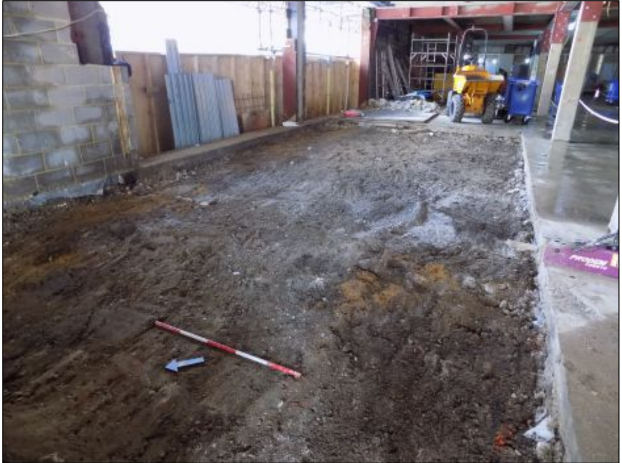
Plate 2. Site prior to excavation facing NE.
