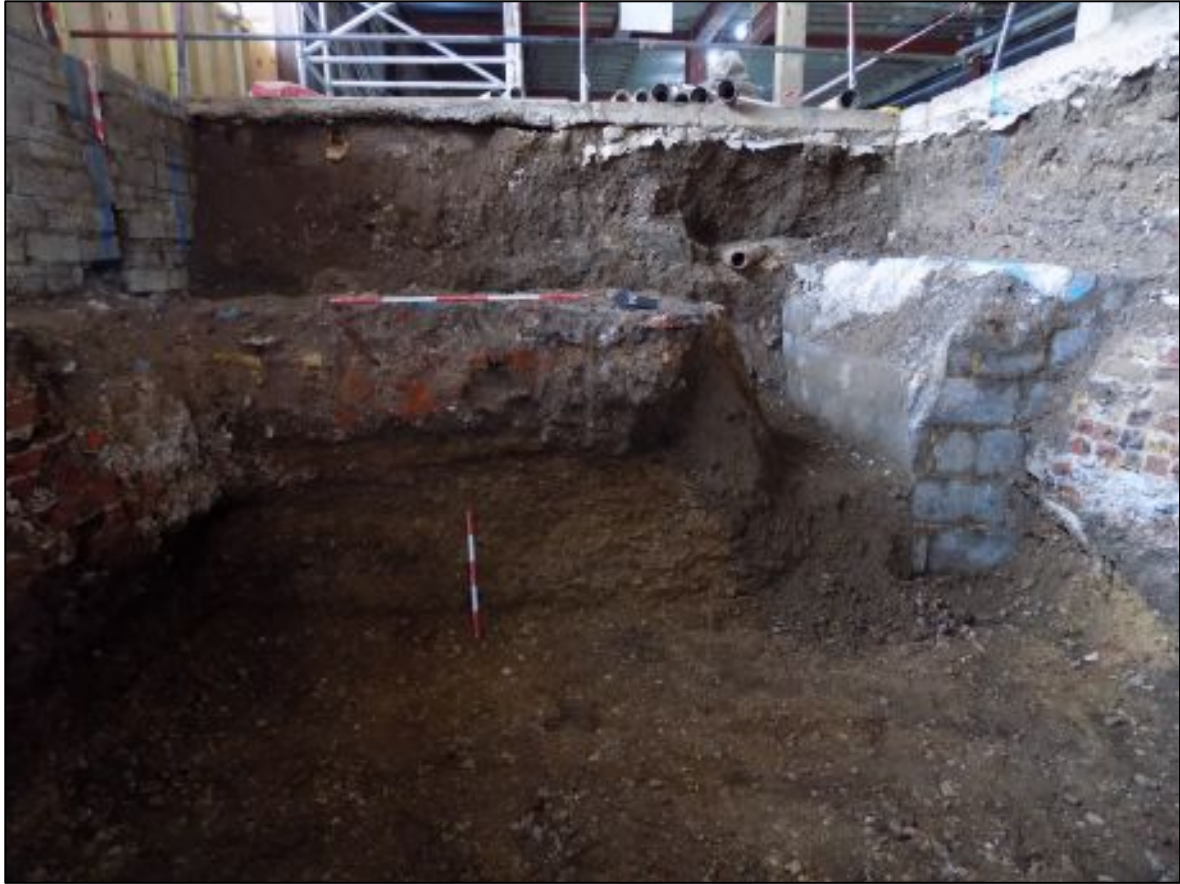
Plate 5. East section facing E showing 19 th and 20 th century foundation.
