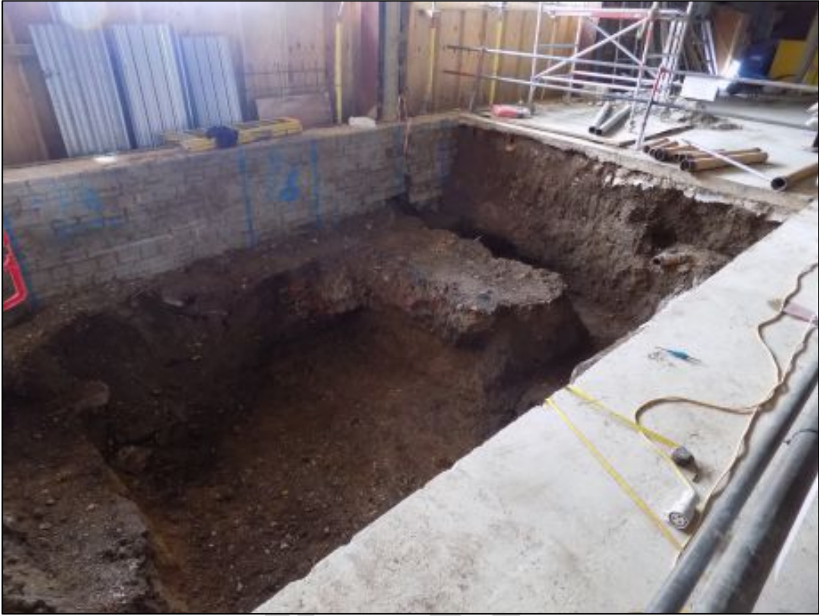
Plate 7. View of site following excavation facing NE.
