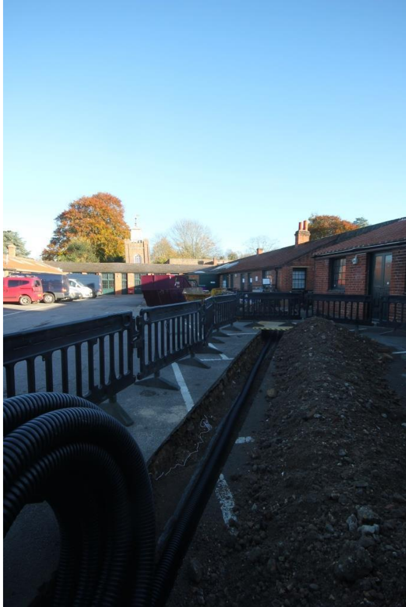
Fig. 4: IS cable trench looking north in the Works Yard, Area II
