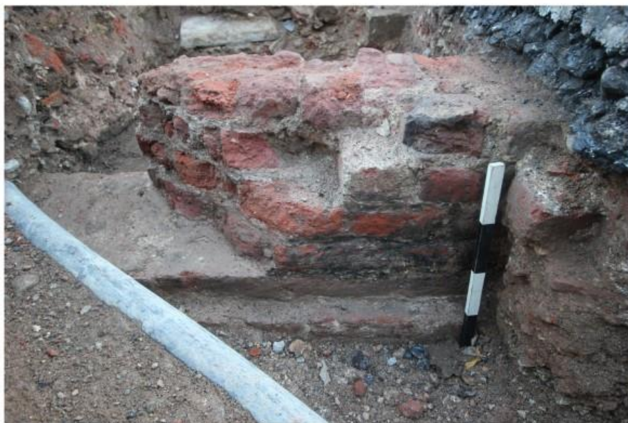
North-facing elevation of wall 136
