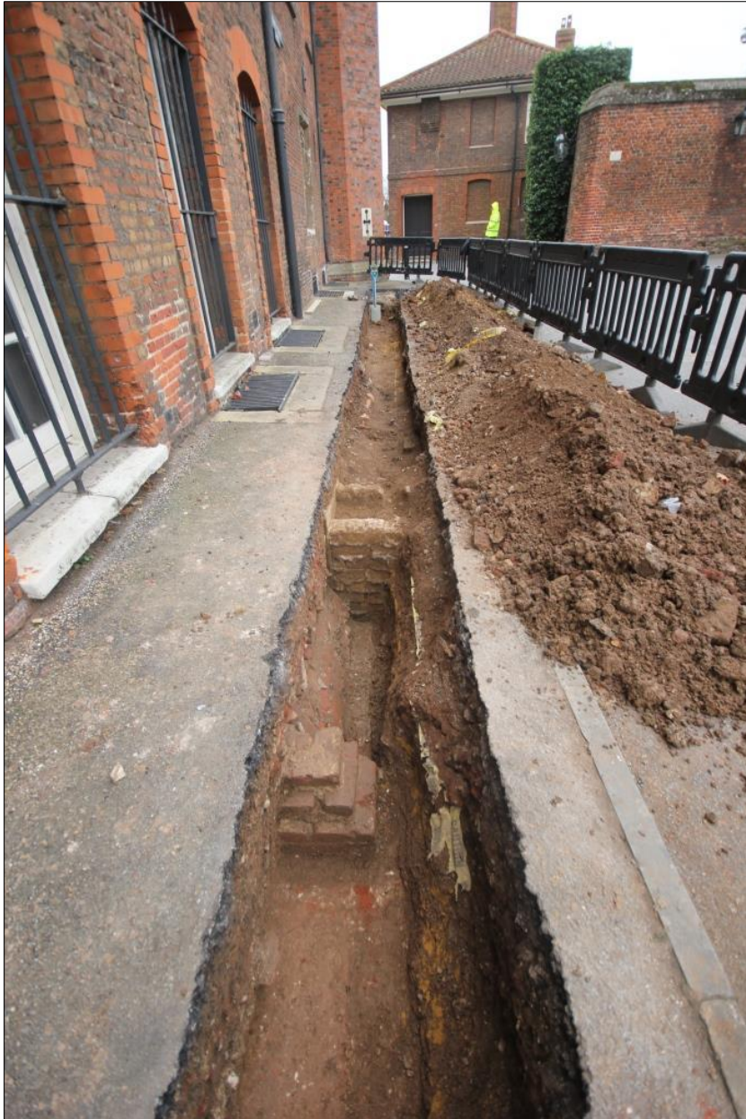
Fig. 7: Area IV, IS Cable trench on Tennis Court Lane, looking west
