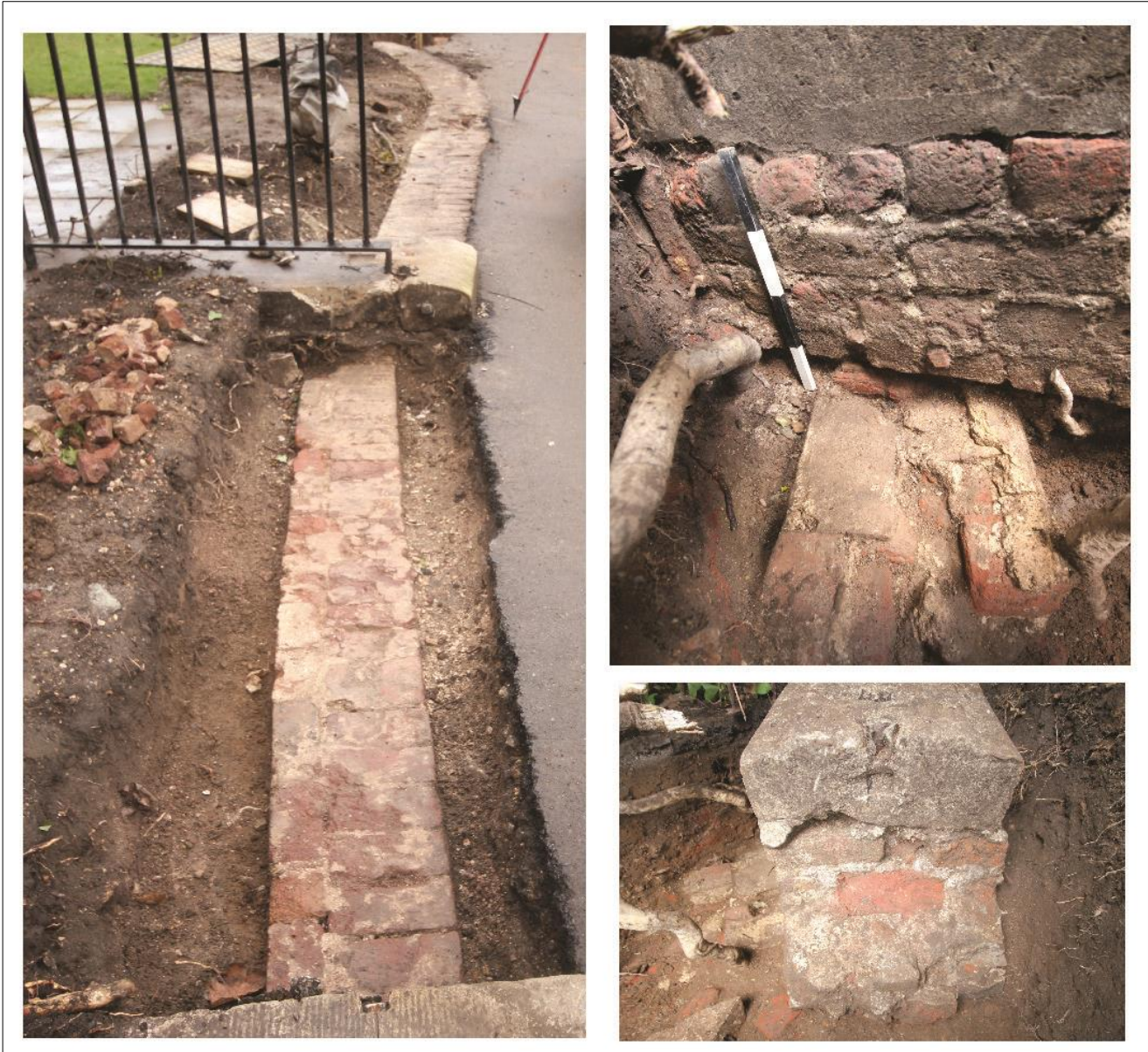
Figure 16: Left: Wall 16 and Wall 15 in the background. Right: Wall 15 overlying Tudor Wall 8 (images from HCP 144).
