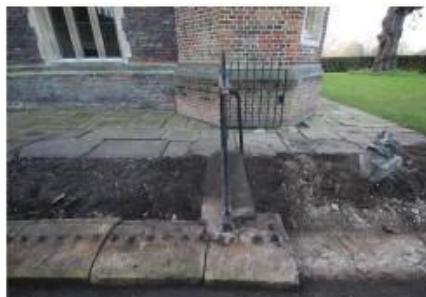
Type III plinth stones in situ, before conservation
