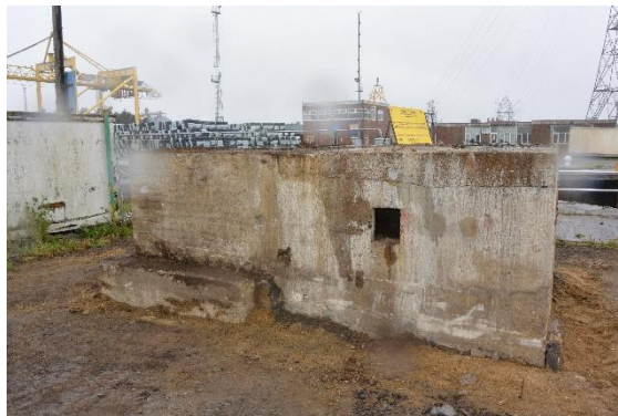
Photo 4.2: Southern elevation. Showing southern embrasure and step round open chamber.
