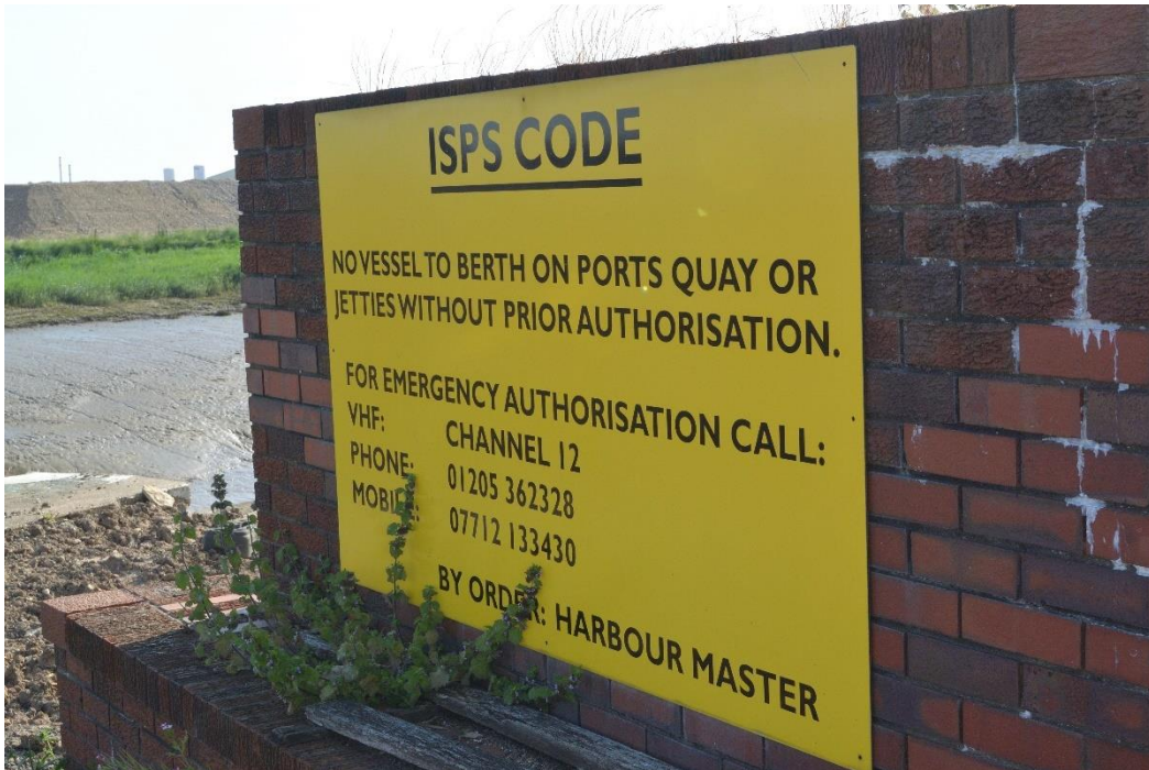
Photo 3.3: Photo of structure before removal of bricks and Port of Boston Signage (eastern end of structure)
