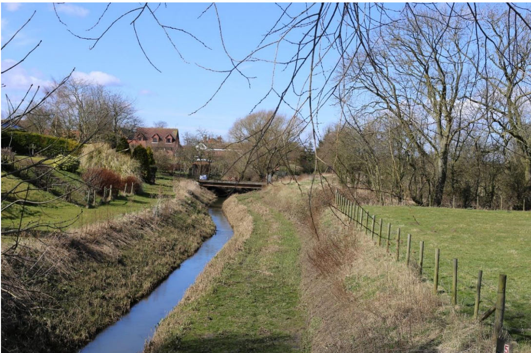
Photo 4: Overview of riverside embankments
