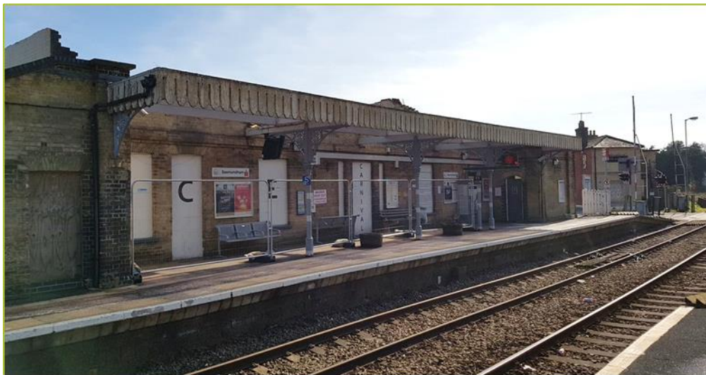
Figure 4: Platform side of Saxmundham Station with historic canopy and brickwork.
