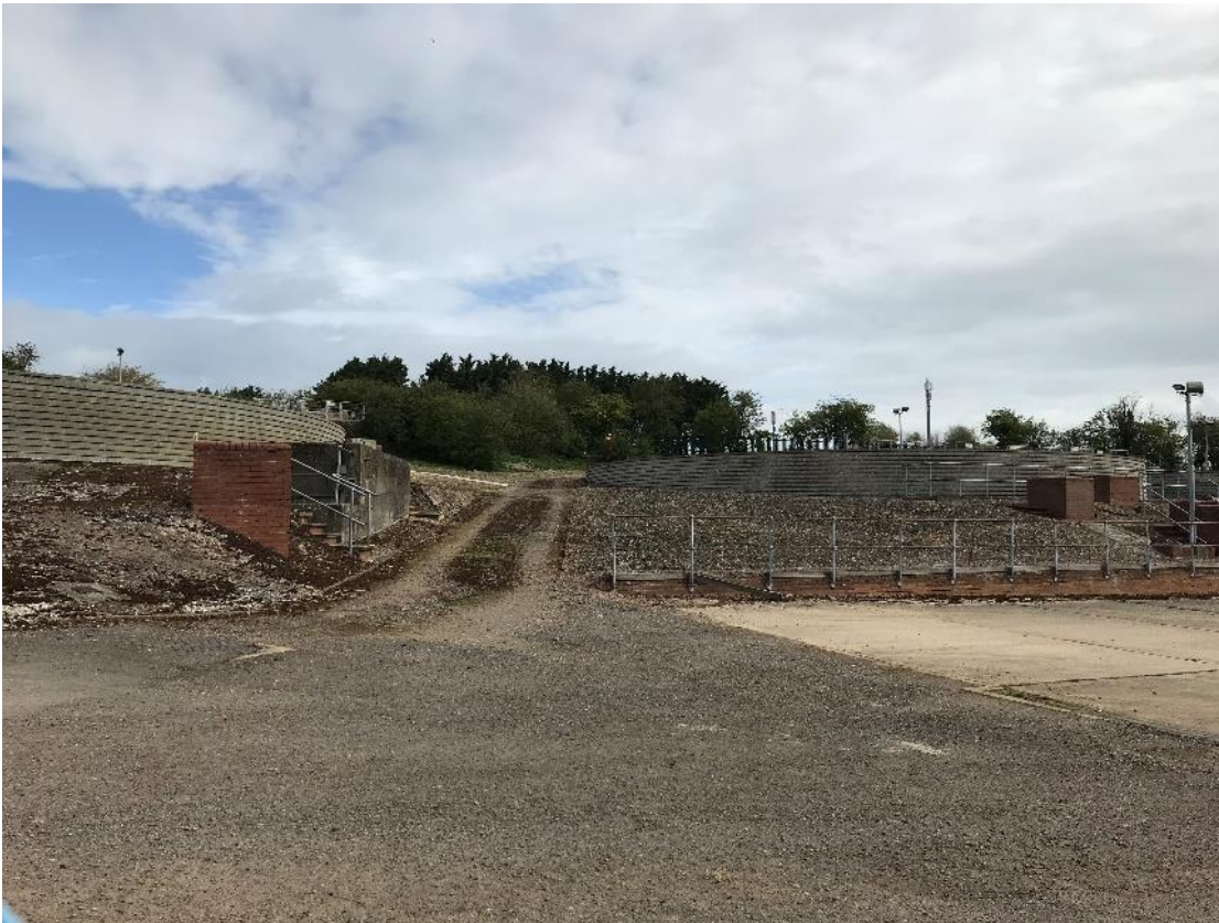
Figure 2. Primary Filter 1 and Secondary Filter 1, facing north-east
