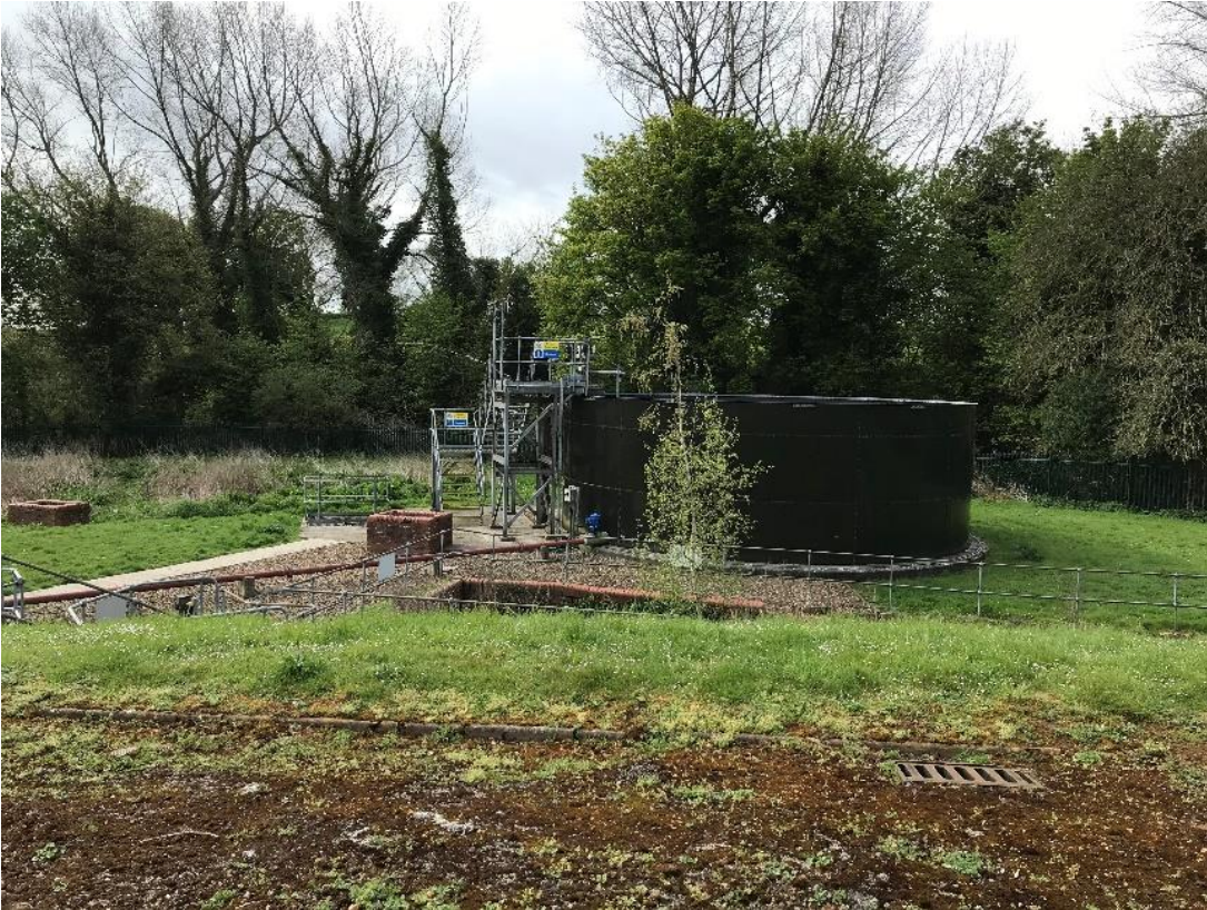
Figure 3. Disused storm tanks and storm tank, facing south
