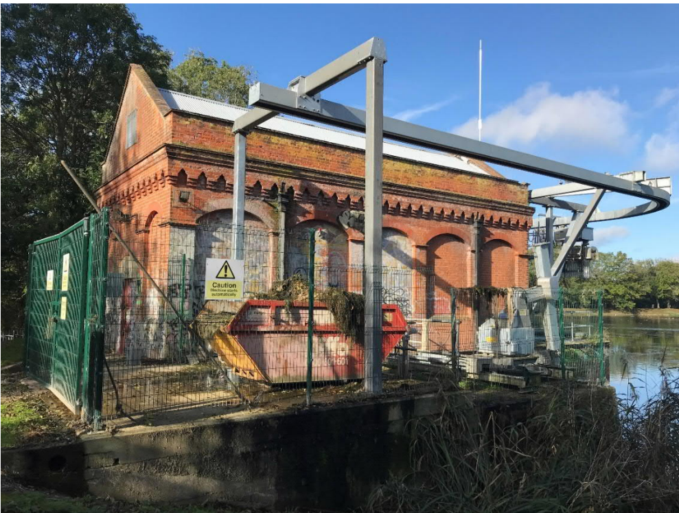
Figure 4.7: Pump house at the southern edge of Hampton Distribution Reservoir, facing south
