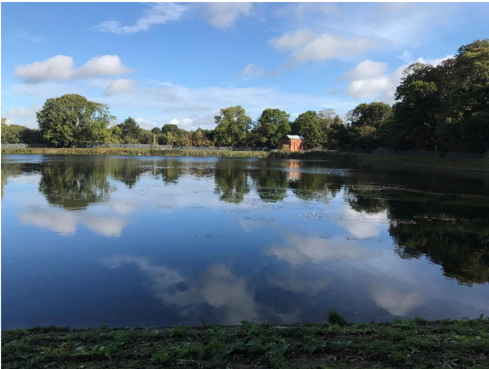
Figure 4.12: Hampton Distribution Reservoir, facing north-west
