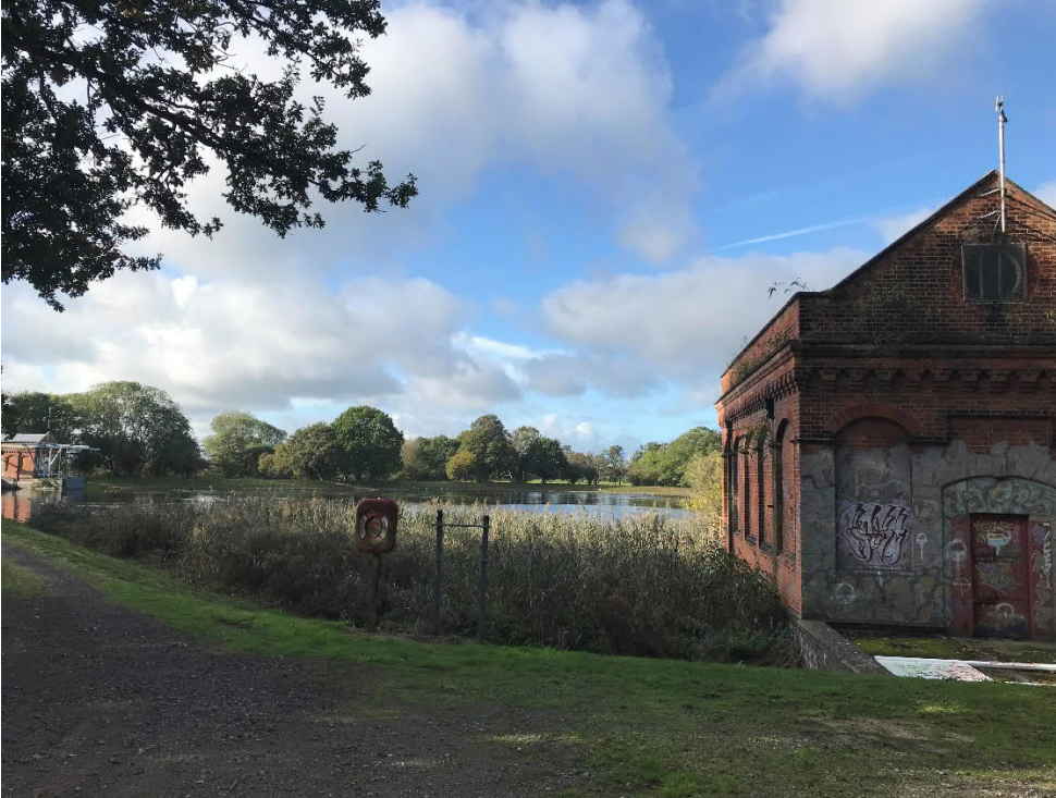
Figure 4.4: Hampton Distribution Reservoir, facing north-west
