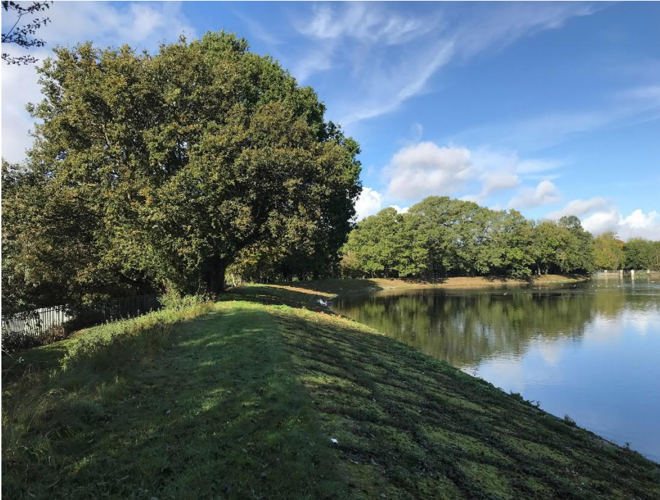
Figure 4.9: Dam crest along south-western margin of Hampton Distribution Reservoir, facing west
