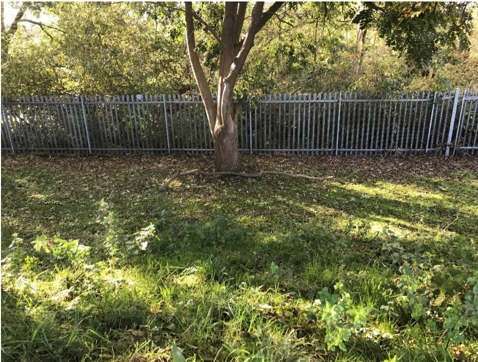
Figure 4.11: Boundary fence along the dam crest along south-western margin of Hampton Distribution Reservoir, facing south-west
