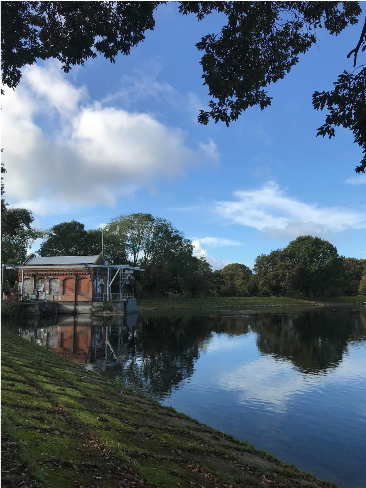
Figure 4.8: Pump house at the southern edge of Hampton Distribution Reservoir, facing south
