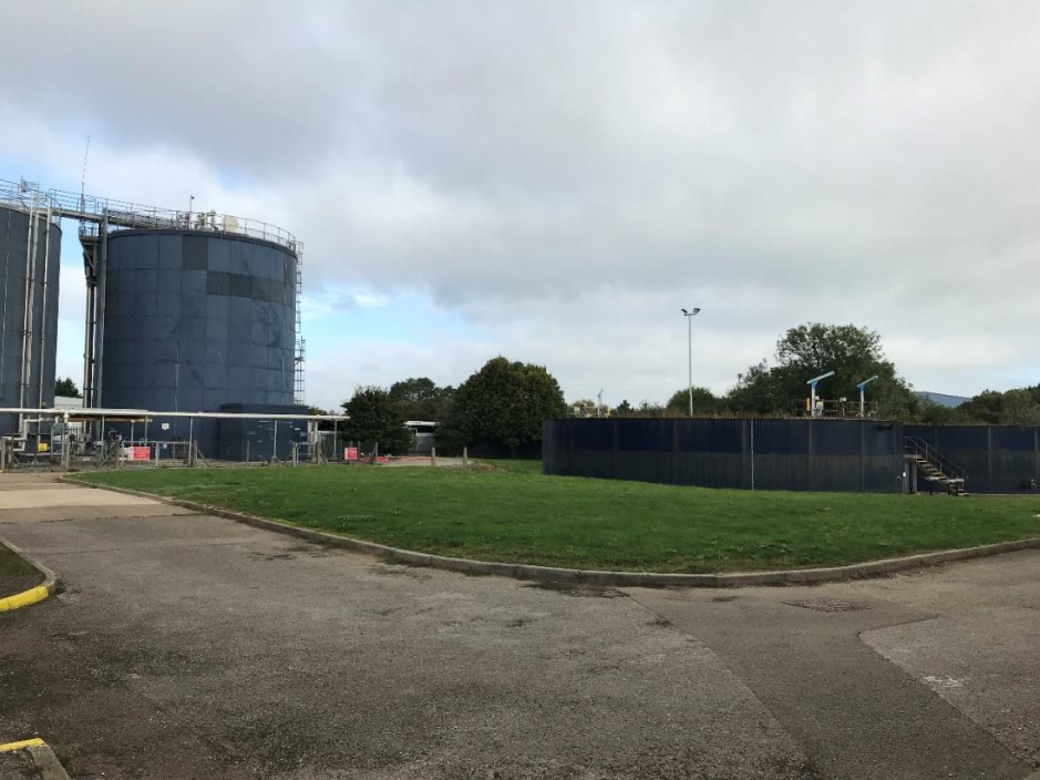
Figure 4.1: View north-east across proposed location of new CHP and associated installations
