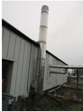
Figure 2 Existing Boiler exhaust stack
