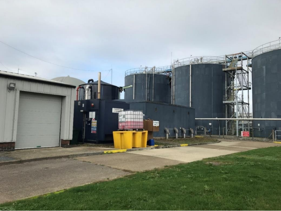
Figure 4.2: View north-west across proposed route of new LV cable
