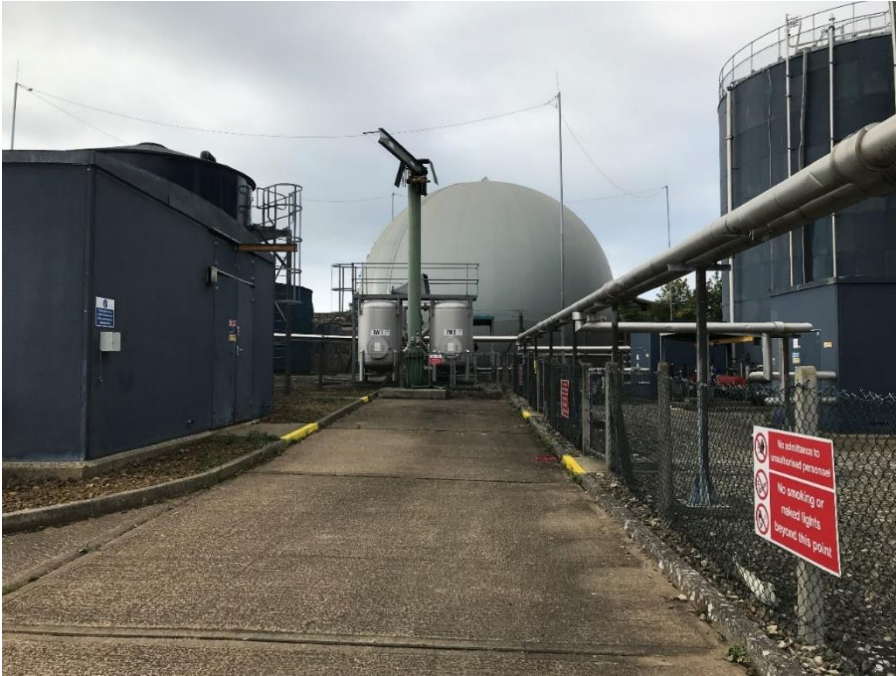
Figure 4.3: View west along proposed route of new biogas pipework
