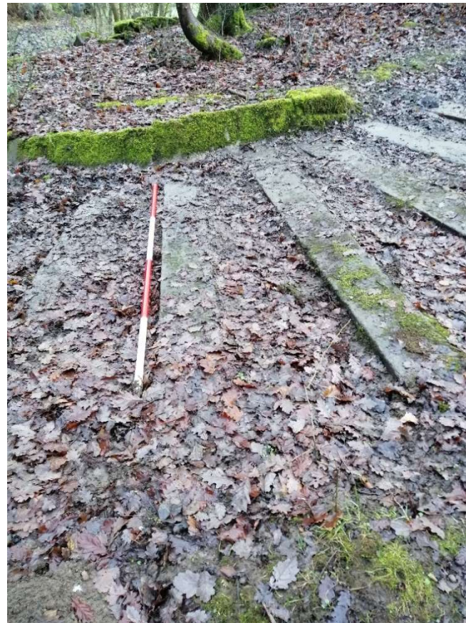
Photo A2.4: Concrete steps near above ground pipe 2. Facing East.
