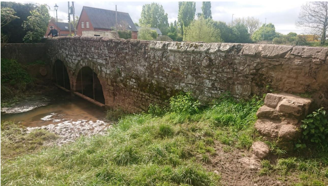
Figure 6: North parapet of Clyst St Mary Bridge, showing stone arches crossing the Mill Leat, with existing concrete flood defence wall and start of Clyst St Mary Village beyond, looking south-east.
