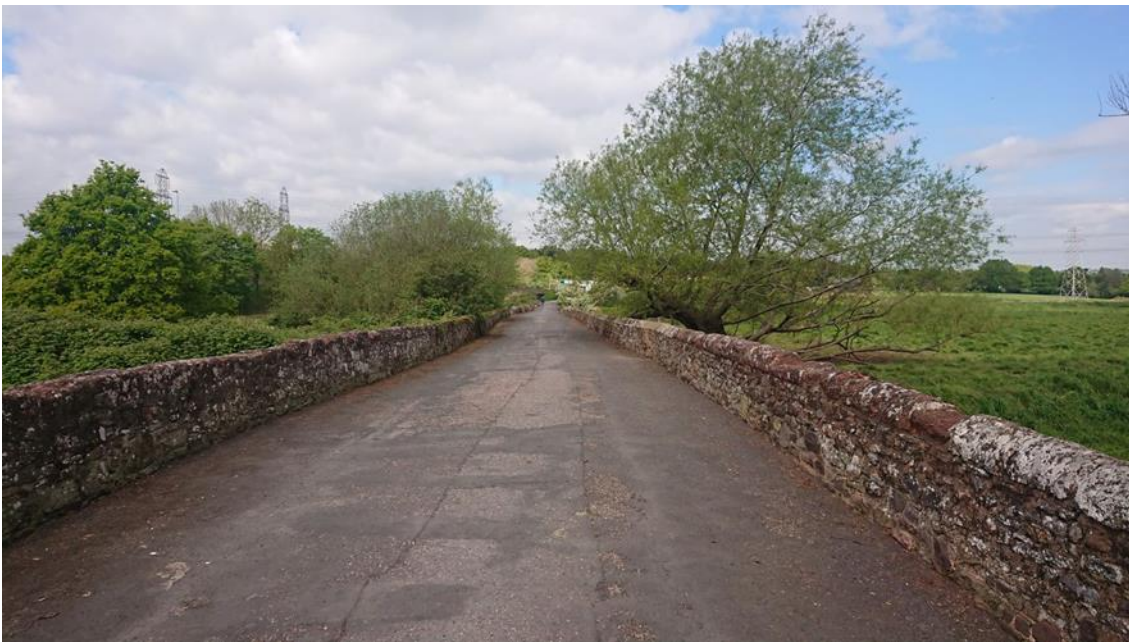
Figure 7: View along the Clyst St Mary Bridge and Causeway, looking west.
